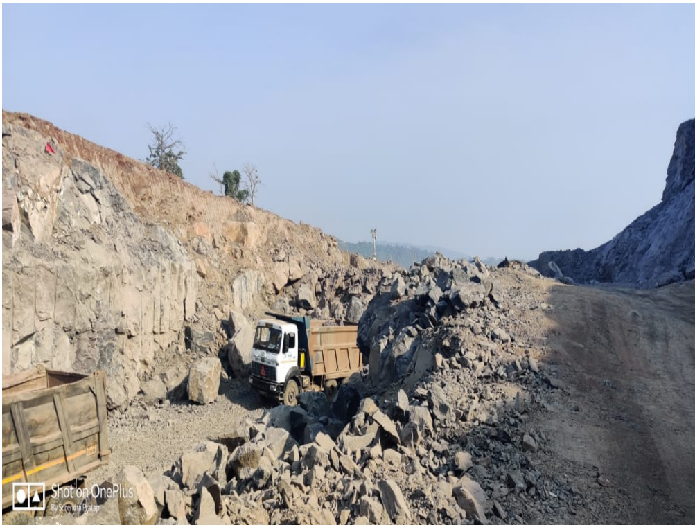
Photo No. 12: Excavated material shifting at At-grade area Ch @ 19+720
