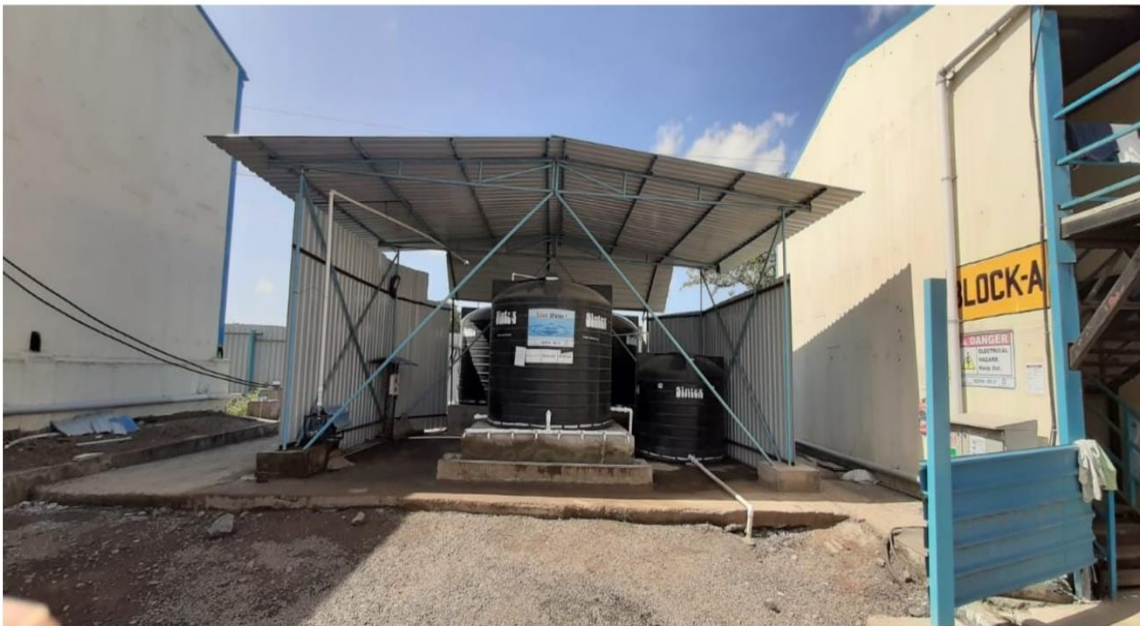
Drinking water facilities at labour camps
