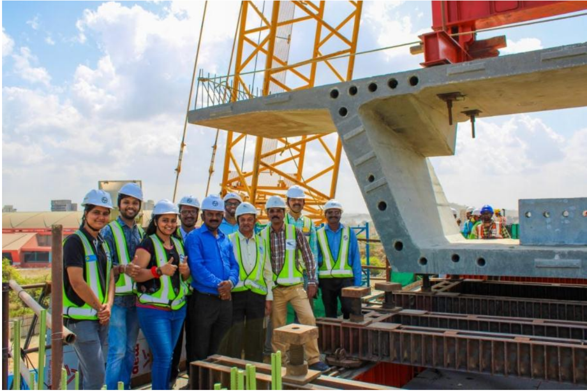
Photo No. 7: 1st Segment Erection at RMP267-268 in progress
