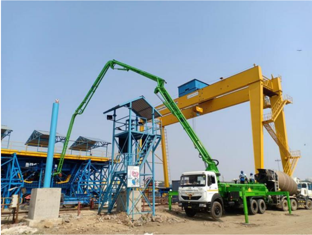
Photo No. 7: Segment Concreting works at Bay-2 in progress
