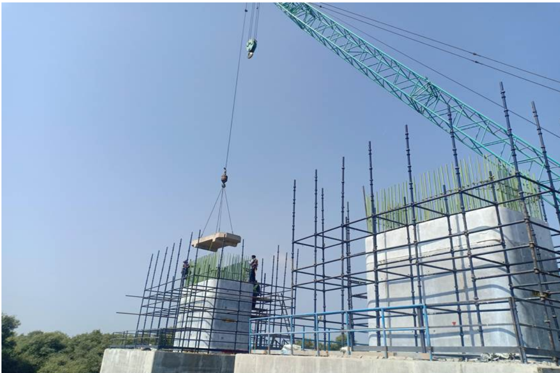
Photo No. 8: Placing of sacrificial slab at MP 238 RHS in progress
