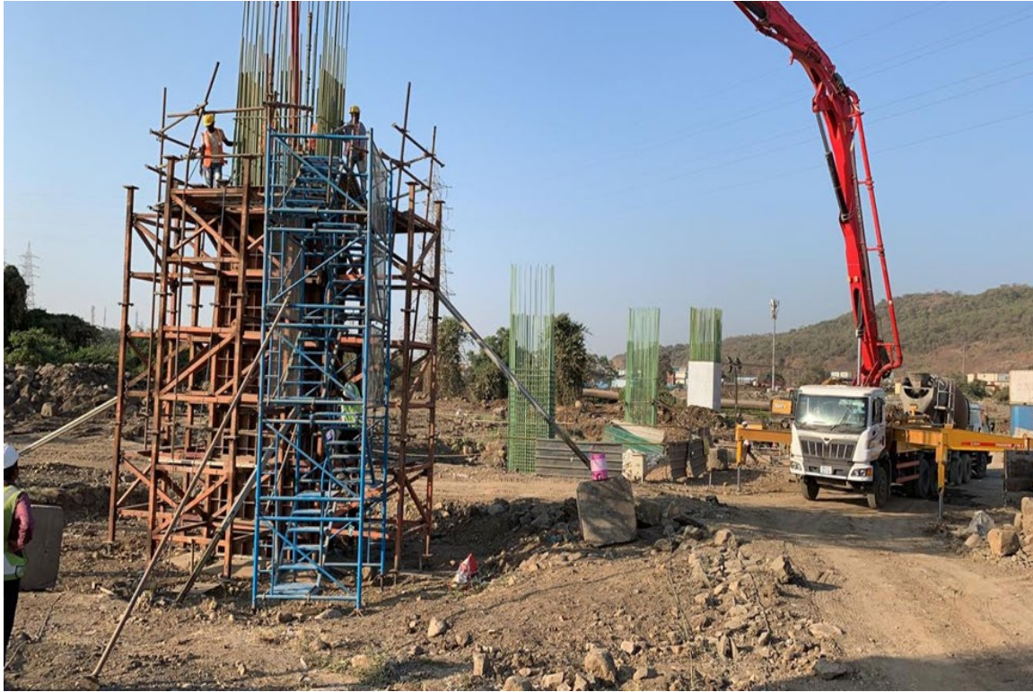
Photo No. 5: Pier concrete at location MPP14 in progress
