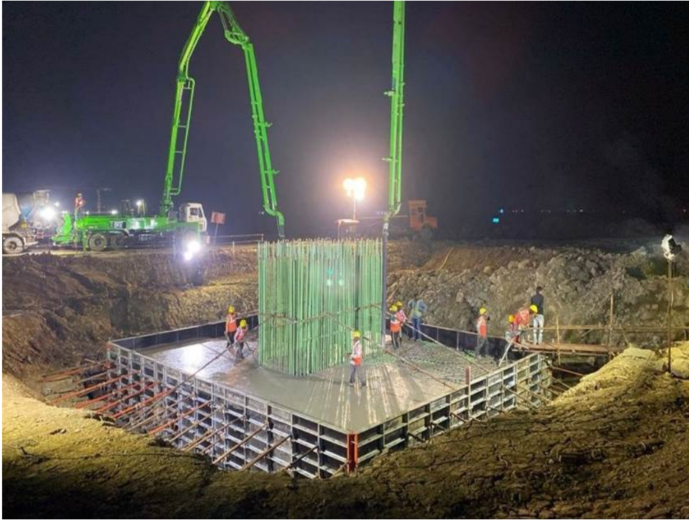
Photo No. 11: Open foundation concreting at ACP 03 in progress
