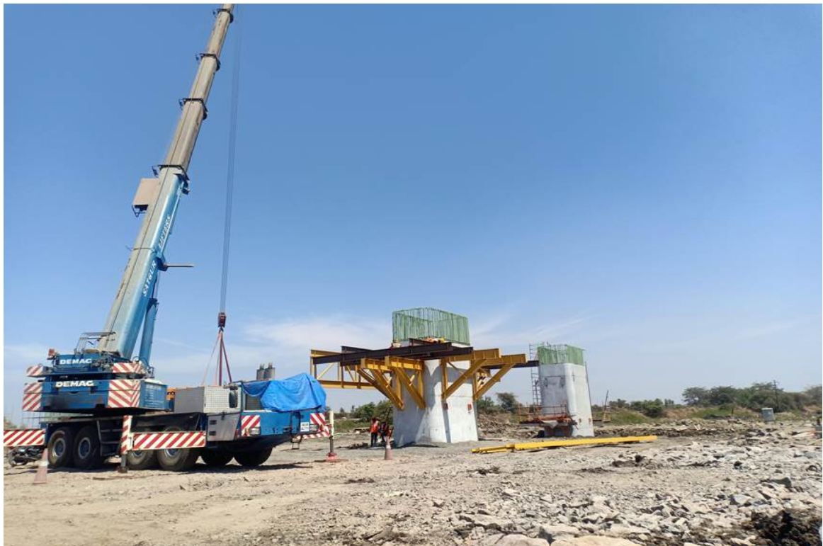
Photo No. 10: Bracket fixing for Pier Cap at MP 243 RHS in progress
