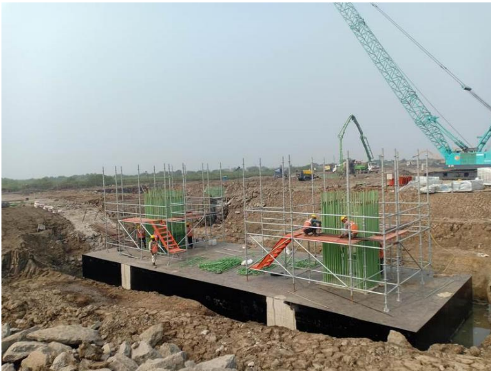
Photo No. 12: Pier reinforcement tying at MP 245 LHS location in progress
