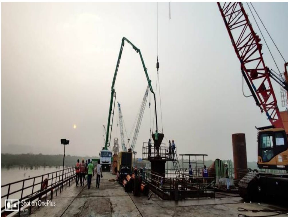
Photo No. 4: Pile concreting at MP 232/02 LHS in progress
