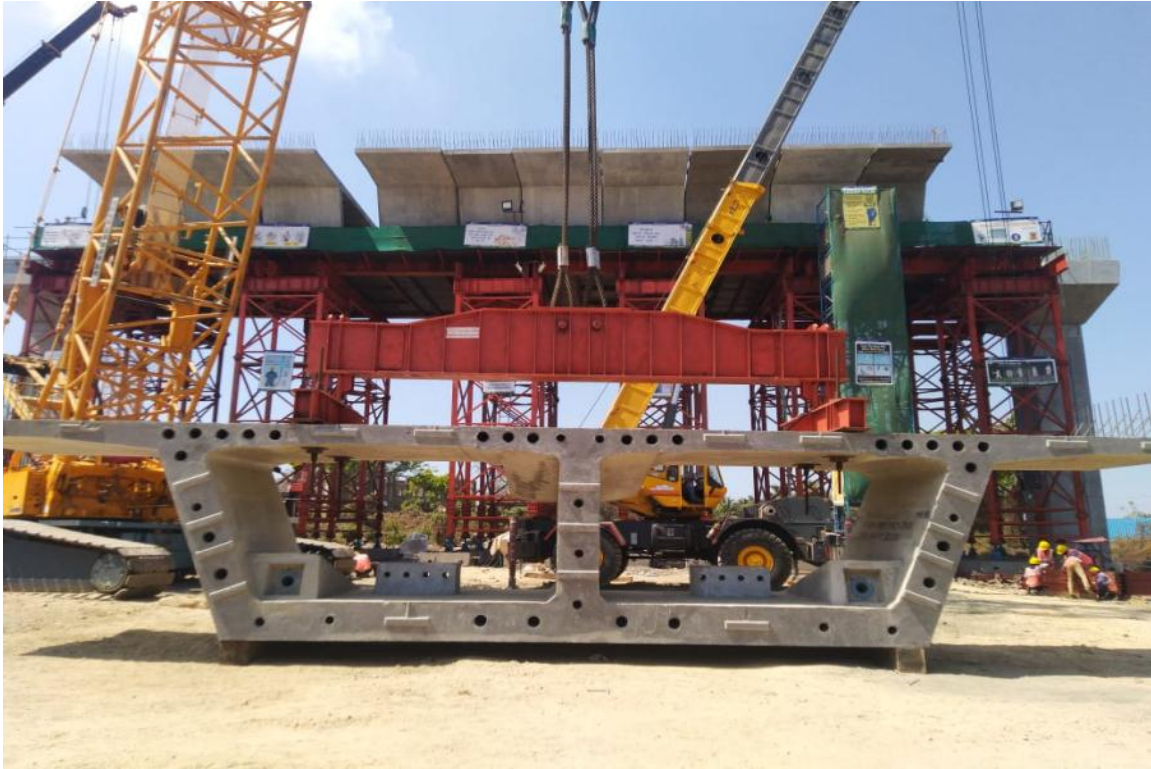
Photo No. 11: Segment erection at span RMP 268-269 in progress
