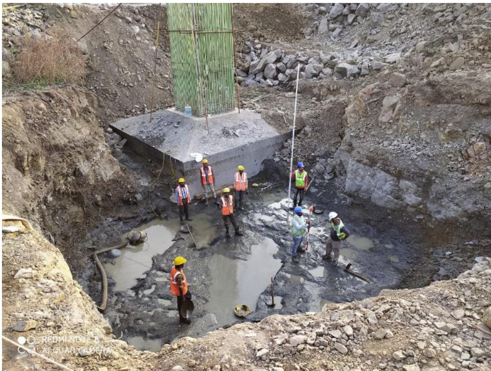
Photo No. 8: PCC Pre-pour checking at LMP 279 P1
