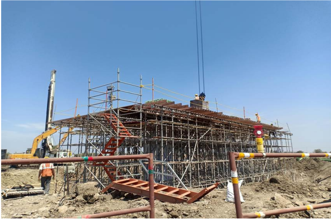
Photo No. 9: Scaffolding and Bottom formwork for Portal Beam at MP 245 LHS in progress
