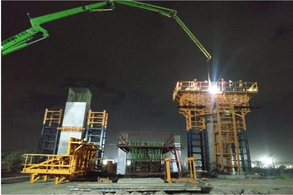
Photo No. 9: Pier Cap casting at location LMP283 in progress
