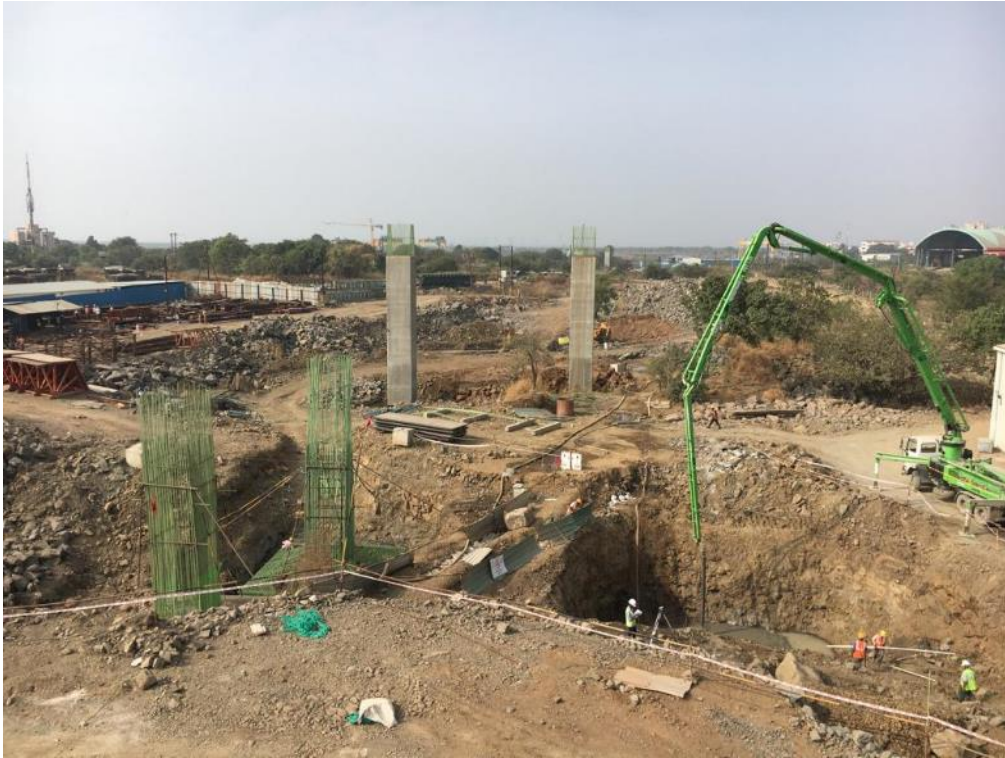
Photo No. 9: PCC Concrete pouring at LMP 279 LHS
