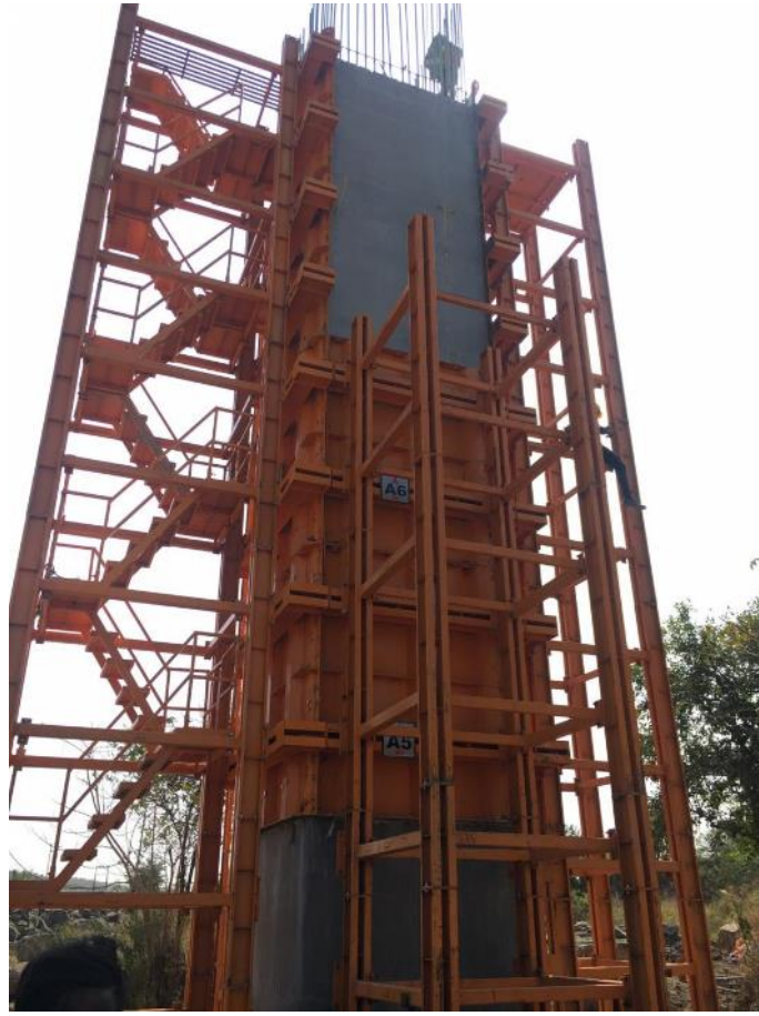
Photo No. 5: Pier casting completed at LMP 269 location
