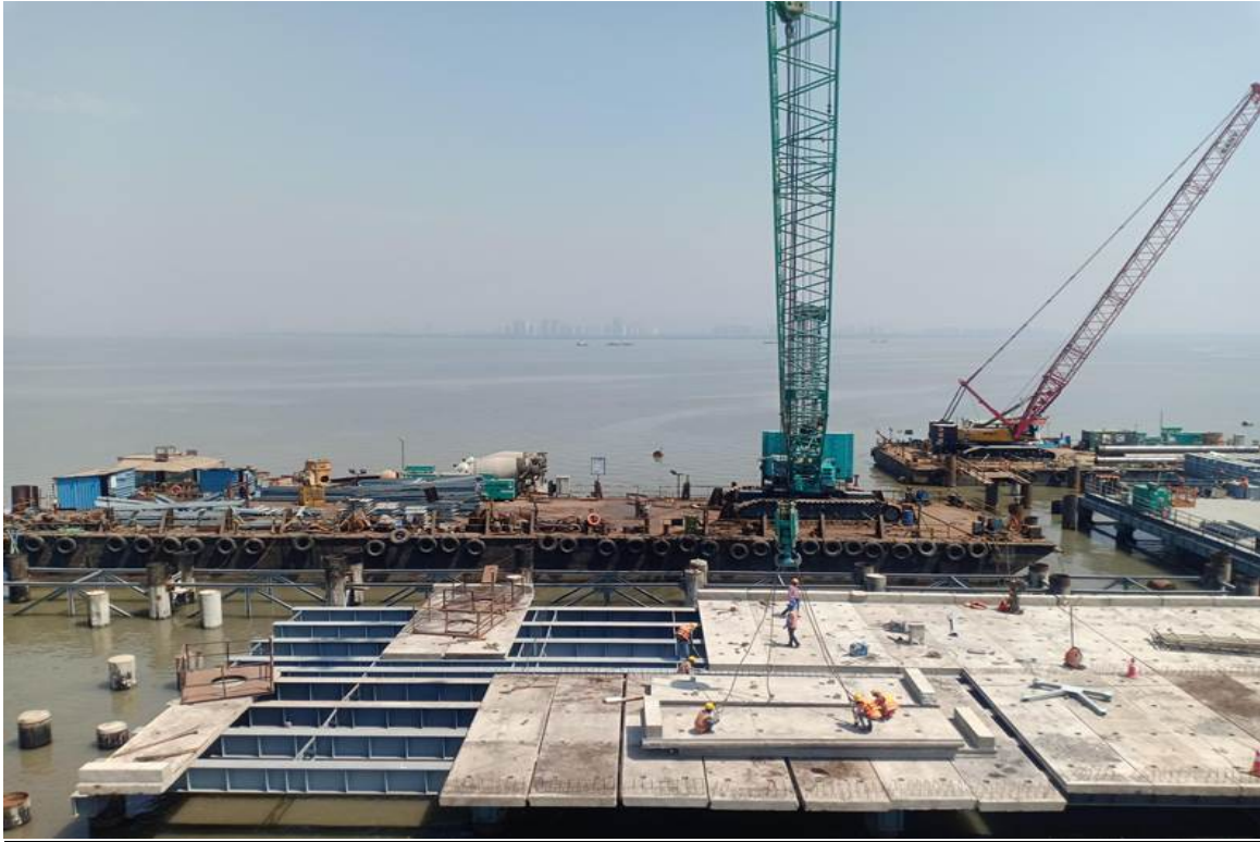
Photo No. 1: Precast Slab erection at TAB/Loading Jetty platform in progress
