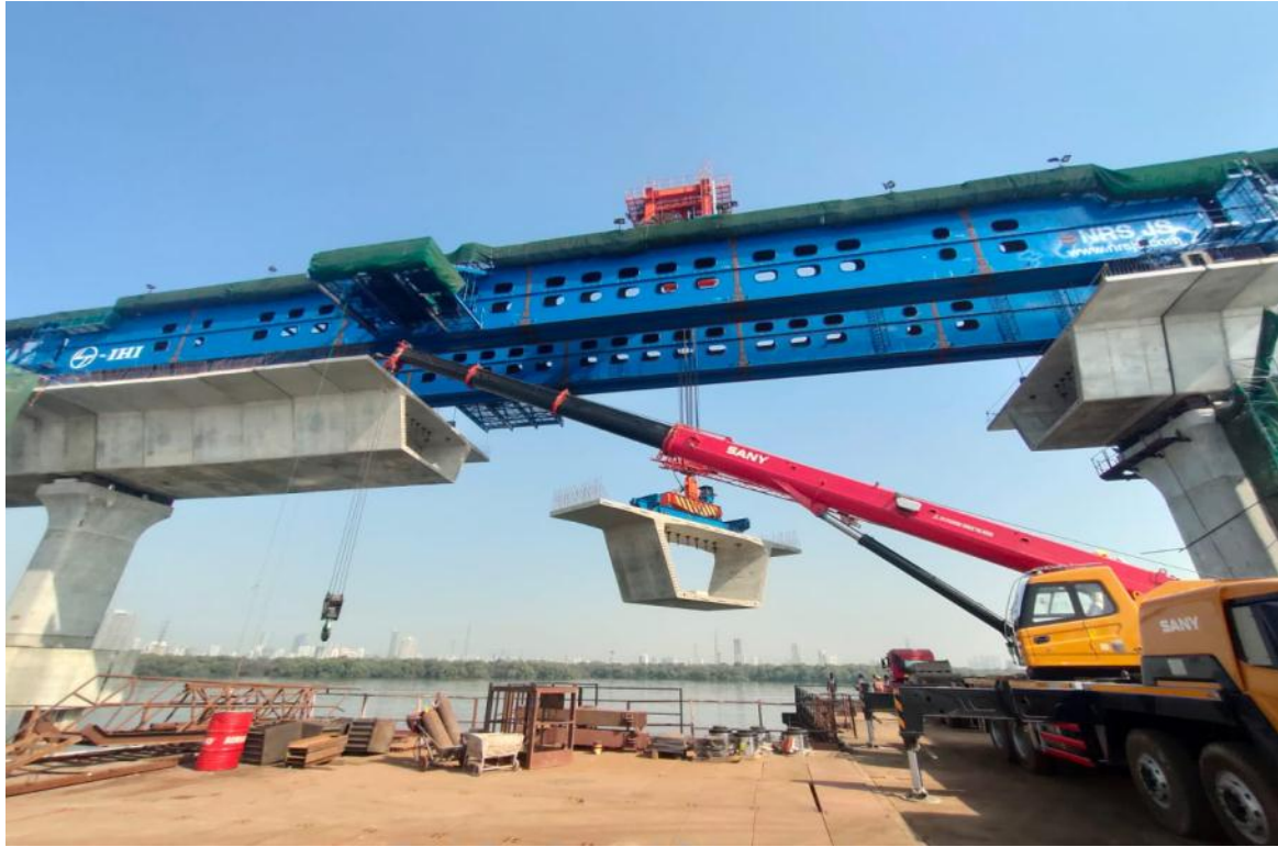
Photo No. 11: MP 14-15 Erection is in progress
