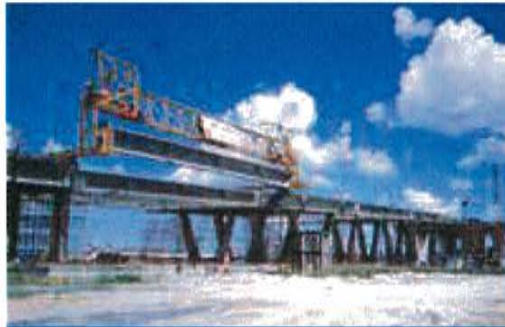
East Coast Parkway - Singapore (1981) 68,250m 2 of deck, 180 beams
