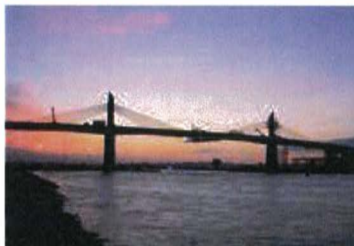
Radès La Goulette Bridge - Tunisia (2007) Main span length 120m
