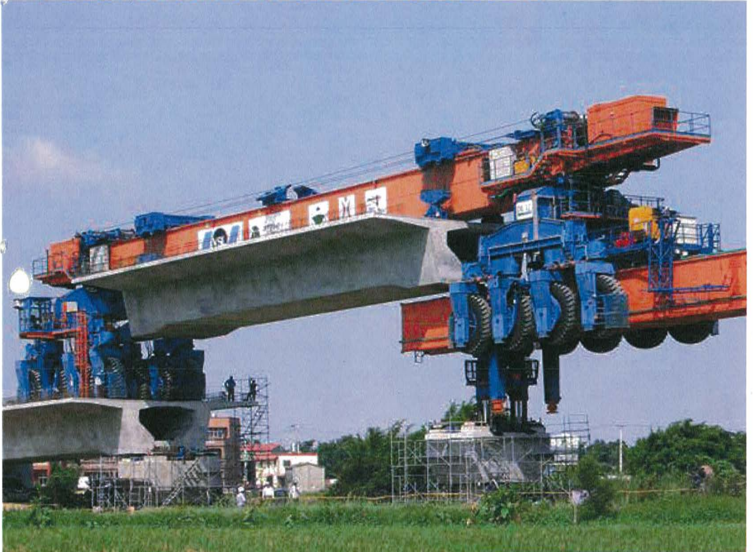
Taiwan High Speed Rail C215- Taiwan (2000-2004) 260,000m 2 of deck, 602 spans
