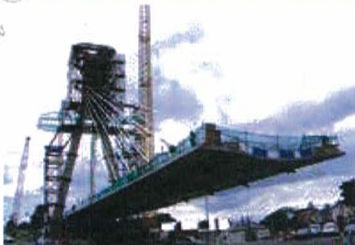
Taney Bridge - Ireland (2002) Main span length: 109m
