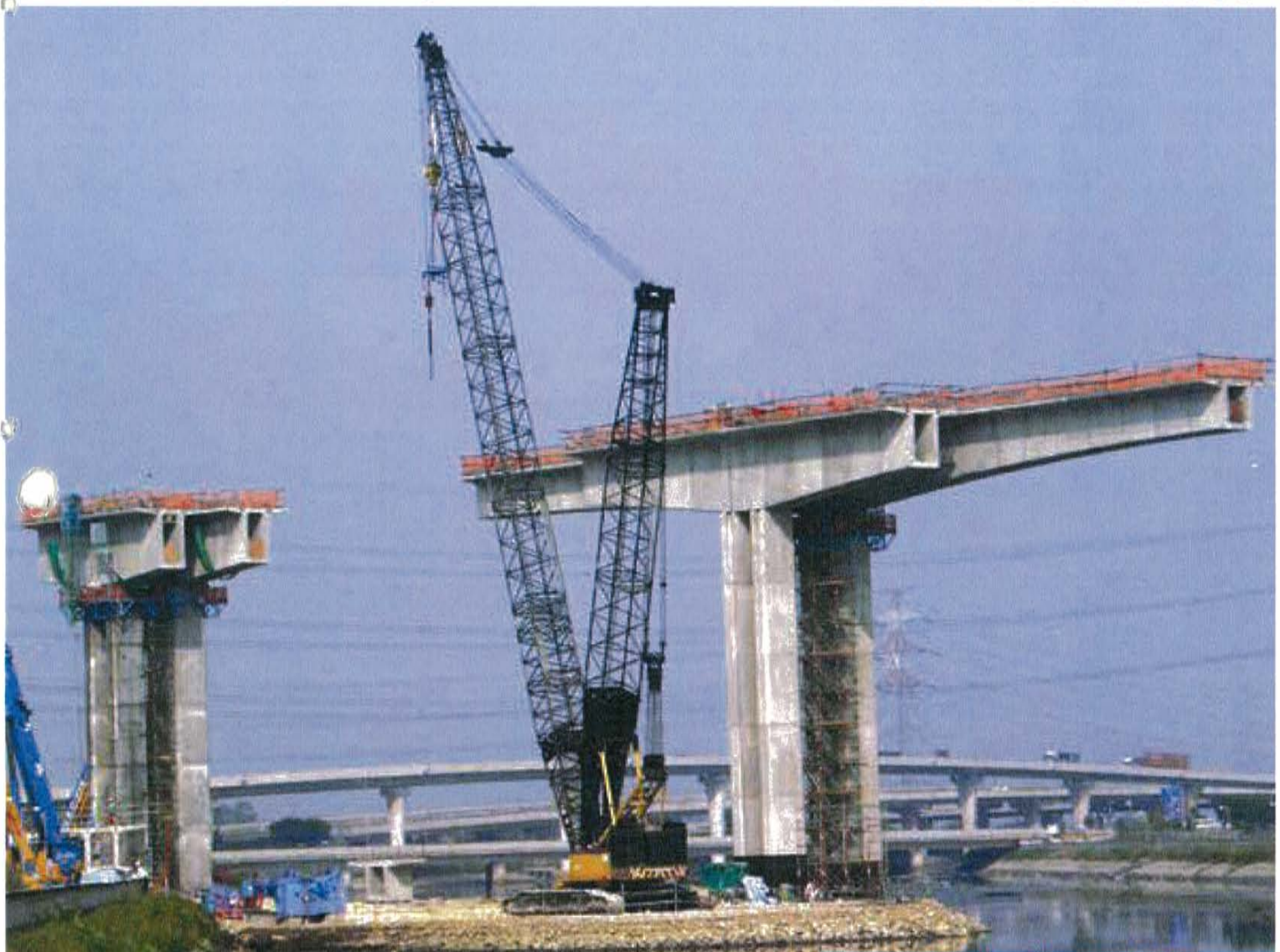
West Rail - Hong Kong (1999-2002) 8,330m 2 of deck, 617 segments
