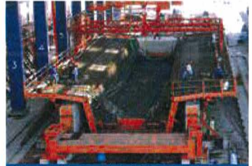
Taiwan High Speed Rail C215 - Taiwan Pretensioning bed and form
