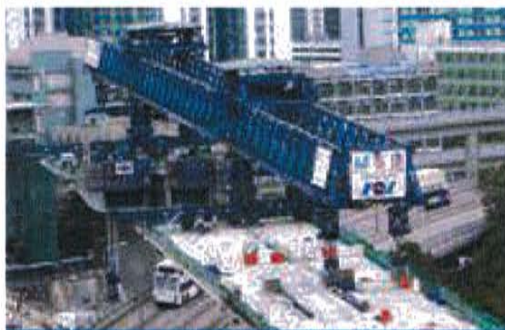
Shatin T3 - Hong Kong (2004-2007) 800m 2 of deck, 1,806 segments
