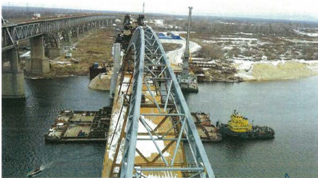
Positioning of span for lift off
