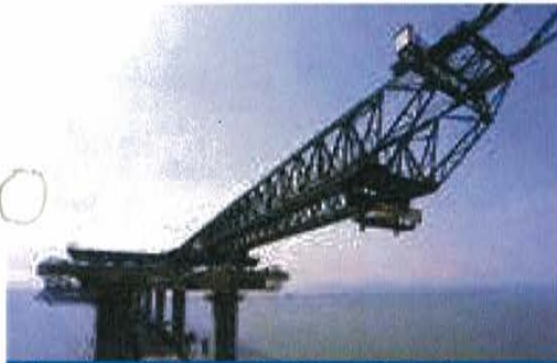
Shenzhen Western Corridor - Hong Kong (2004-2005) 90,800m 2 of deck, 1,879 segments
