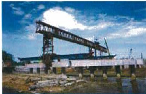
Tutong Lumut Coastal Highway - Brunei (2001-2003) 6,100m 2 of deck, 210 beams
