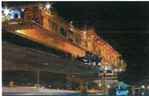
Light Rail Transit Dubai - UAE (2007-2009) 430,000m 2 , 16,450 segments
