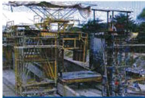
Pakse Bridge - Laos Match cast long line
