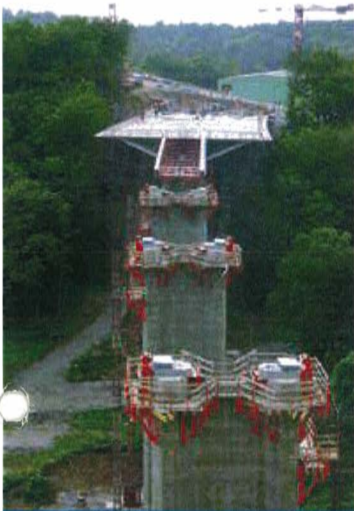
Rybný Potok - Czech Republic (2005) 58m of span length, 10,858m 2 of surface
