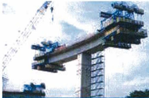
Ma Wan - Hong Kong (1999) 48m main span length, 15 cantilevers
