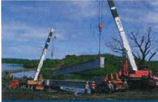
Palau Island Bridge - Palau (2003-2005) 4,000m 2 of deck, 52 beams
