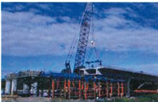
West Link - Australia (2004-2005) 108,000m 2 of deck, 3,013 segments
