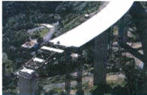
Caguas River Bridge - Puerto Rico (1981) 385m of bridge length
