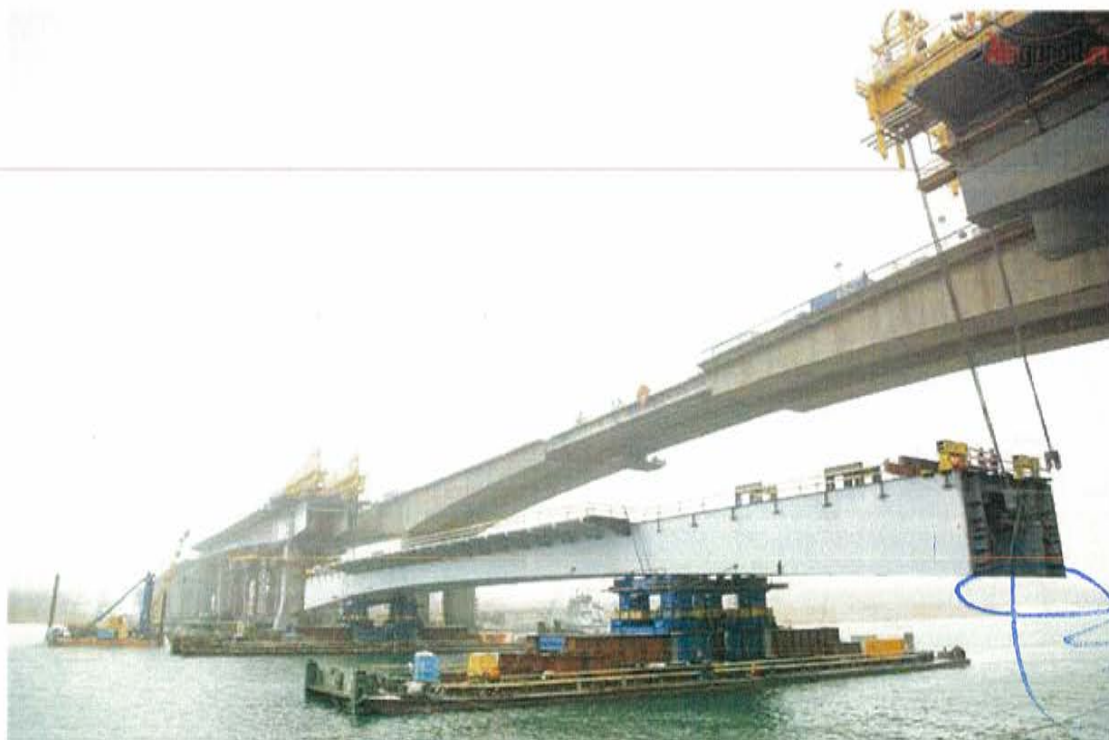
Preparation to connect the lifting cables to the span
