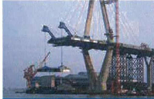
Industrial Ring Road - Thailand (2005-2006) Lifting of 500t bridge deck segment
