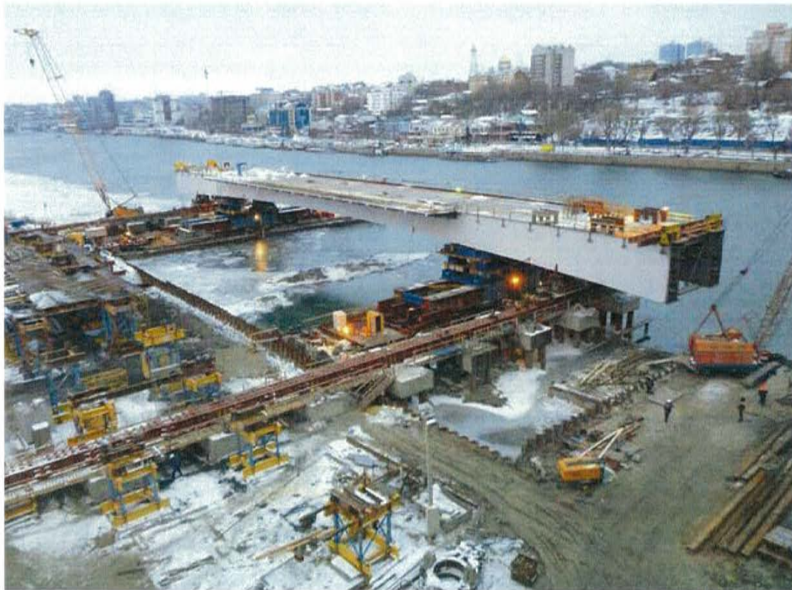
Load out preparation of the span onto the barges
