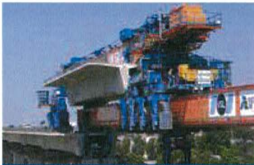
Taiwan High Speed Rail C215 - Taiwan (2000-2004) 260,000m 2 of deck, 602 spans
