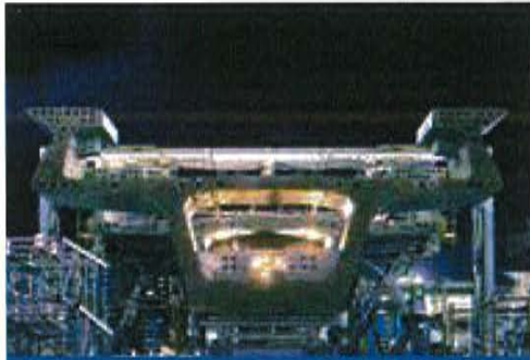
Light Rail Transit - Dubai (2007-2009) Casting Yard
