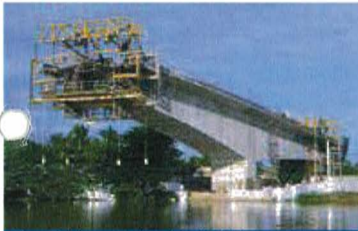
Sinu Bridge - Columbia (2005) 150m main span length, 2 cantilevers
