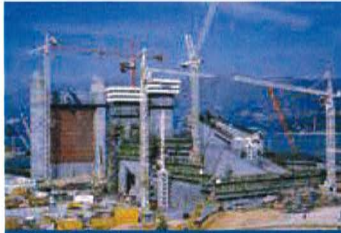
Tsing Ma Bridge - Hong Kong Pier climbform
