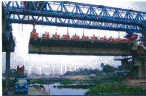
Deep Bay Link - Hong Kong (2004-2005) 108,000m 2 of deck, 3,014 segments
