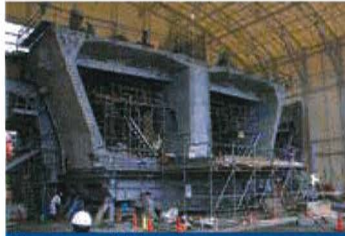
Kisosansen Bridge - Japan Match cast short line cells
