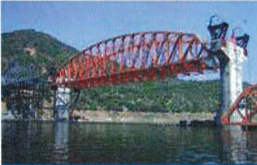
Infiernillo II Bridge - Mexico (2000) Lifting of 3 arched steel trusses (600t each)
