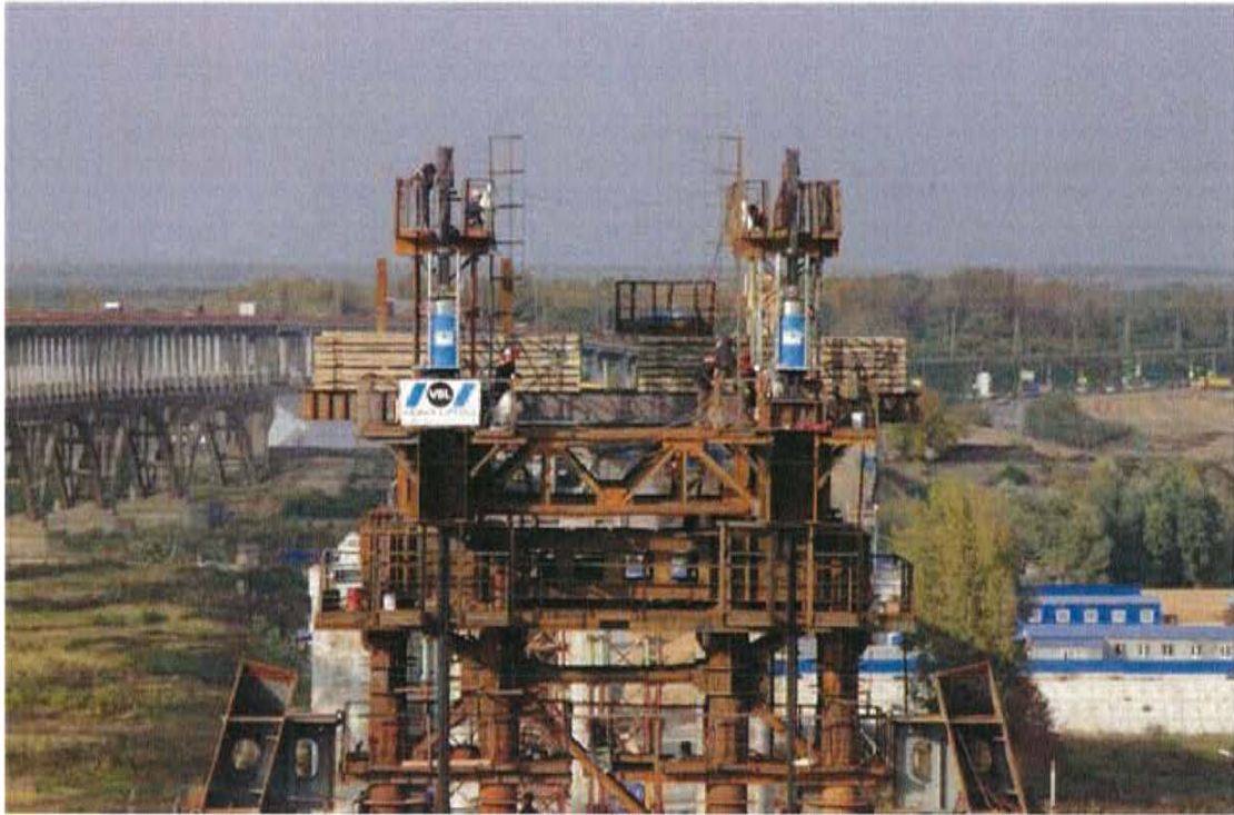
VSL equipment ready for lift off
