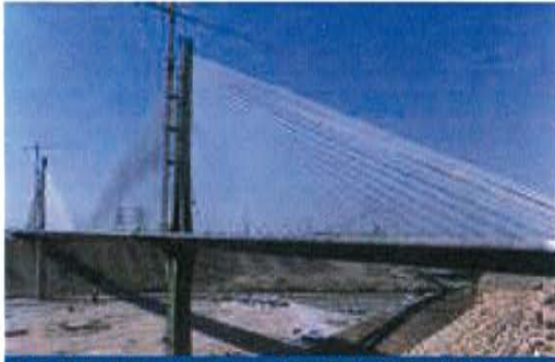
Wadi Leban Bridge - Saudi Arabia (1997) Main span length: 405m
