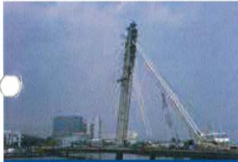
Keppel Bay Bridge - Singapore (2007) 4,132m 2 of deck, 77 bridge segments
