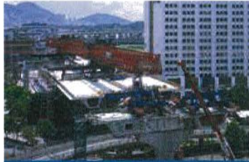
Lai Chi Kok - Hong Kong (2004-2006) 63,000m 2 of deck, 1,771 segments
