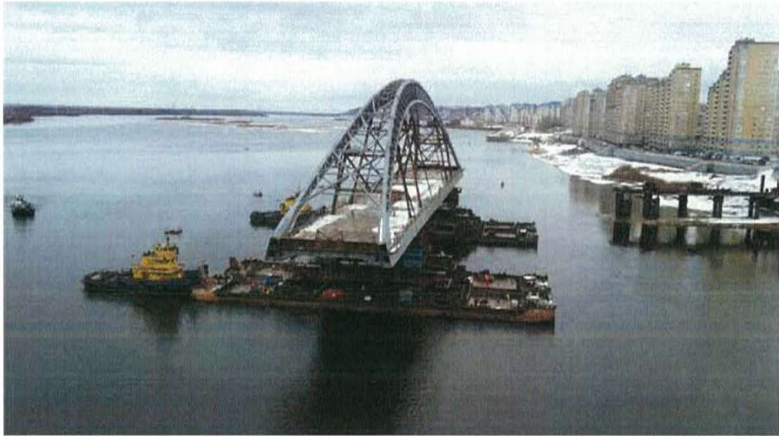
Transfer of span to bridge location
