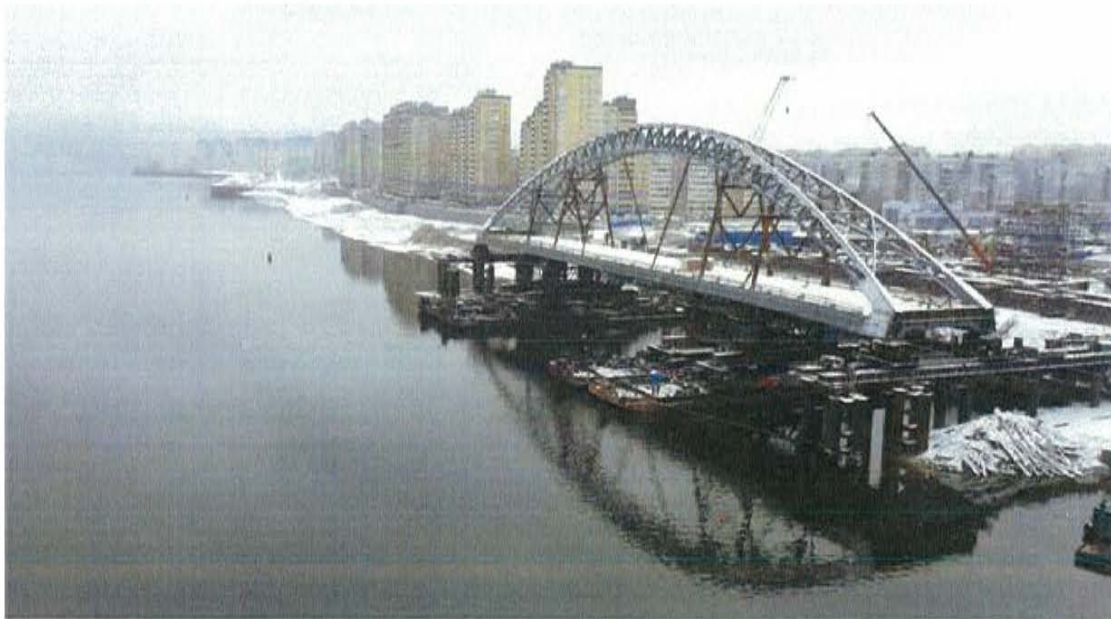
Transfer of span onto barges
