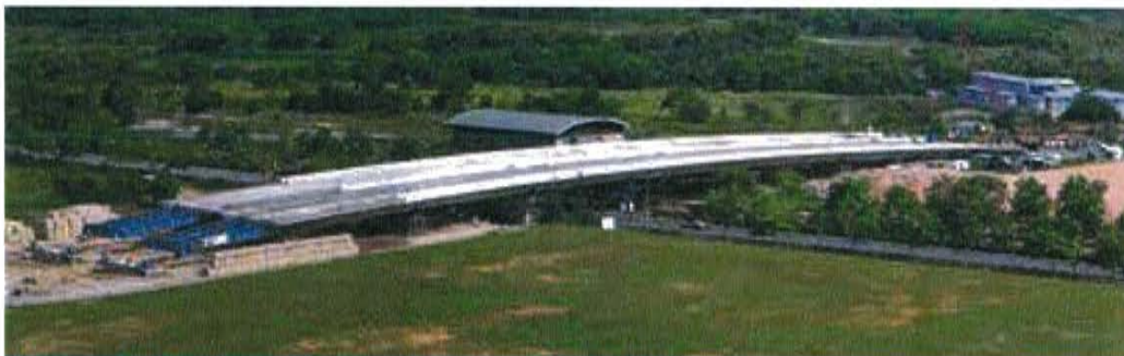
Tampines Sengkang Flyover - Singapore (2002-2003) 5-63m of span length, 10,623.85m 2 of surface
