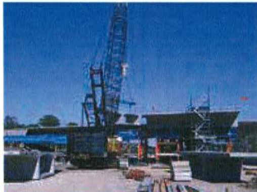
West Link - Australia (2004-2005) 63,000m 2 of deck, 3,013 segments
