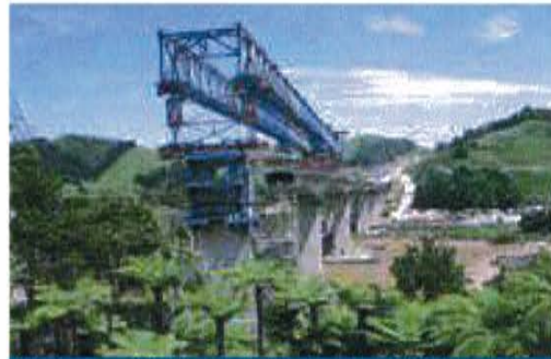
Waiwera Viaduct - New Zealand (2007-2008) 12,130m 2 of deck, 356 pre-cast segments
