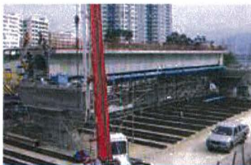
East Rail - Hong Kong (2000-2003) 58,320m 2 of deck, 4,449 segments
