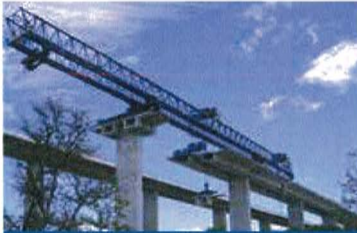
Second Gateway Bridge - Australia (2008-2010) 29,526m 2 of deck, 700 precast elements
