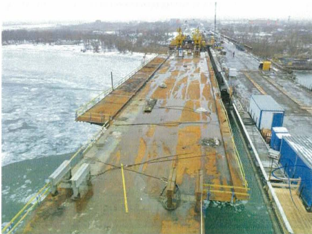
Span at final level
