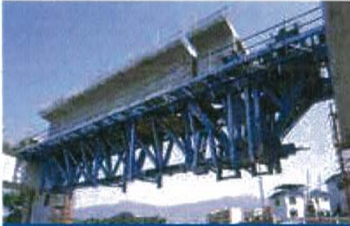
West Rail - Hong Kong (1999-2002) 116,667m 2 of deck, 8,642 segments
