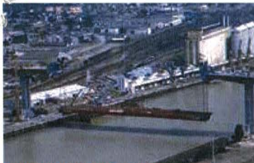
Loire River Bridge - France Lifting of centre span (2,400t)
