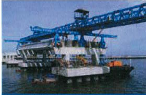
Cebu Coastal Road - Philippines (2001-2002) 24,000m 2 of deck, 320 beams
