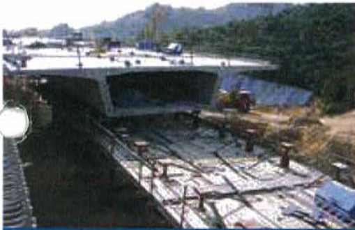
Deep Bay Link - Hong Kong (2004-2005) 108,000m 2 of deck, 3,014 segments
