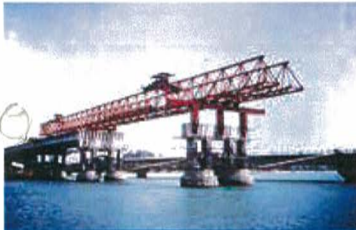
Sarasin Bridge - Phuket, Thailand (1991-1992) 7,800m 2 of deck, 182 beams
