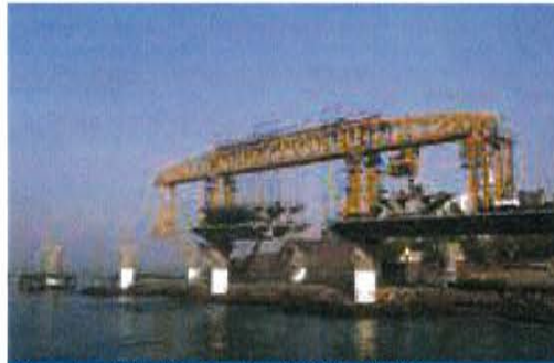
Bandra Worli - India (2002-2006) 132,130m 2 of deck, 2,332 segments
