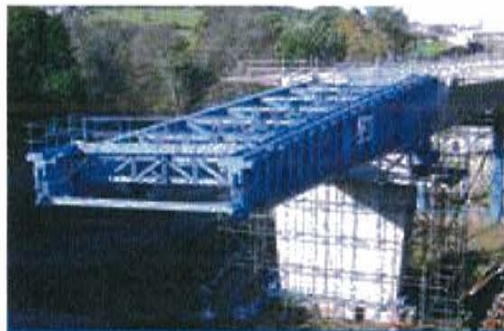
Brides Glens Bridge - Ireland (2003-2004) 45.9-65m of span length, 3,200m 2 of surface
