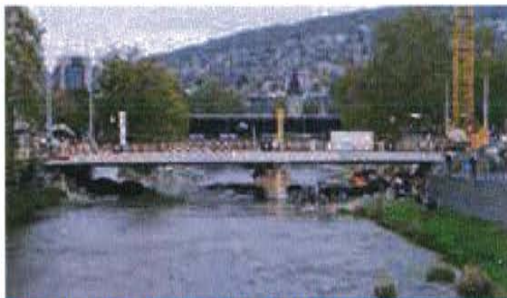
Gessnerbrück - Switzerland (2006) Lifting of Bridge 3'500t for 23m
