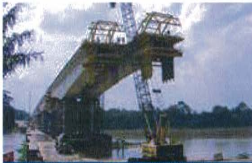
Chenur Bridge - Malaysia (2002-2004) 100m main span length, 7 cantilevers
