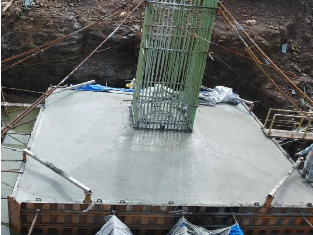
Photo No. 1: Foundation RP-38 (Chirle) concrete pouring completed
