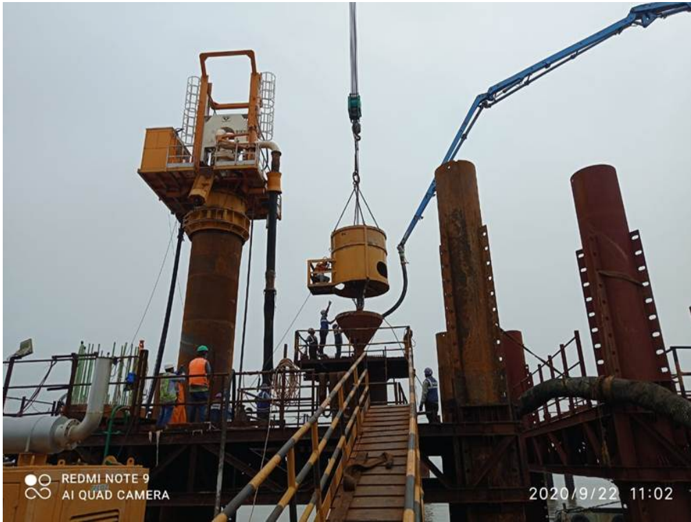
Photo No. 3: Pile concreting at MP 181 LHS in progress
