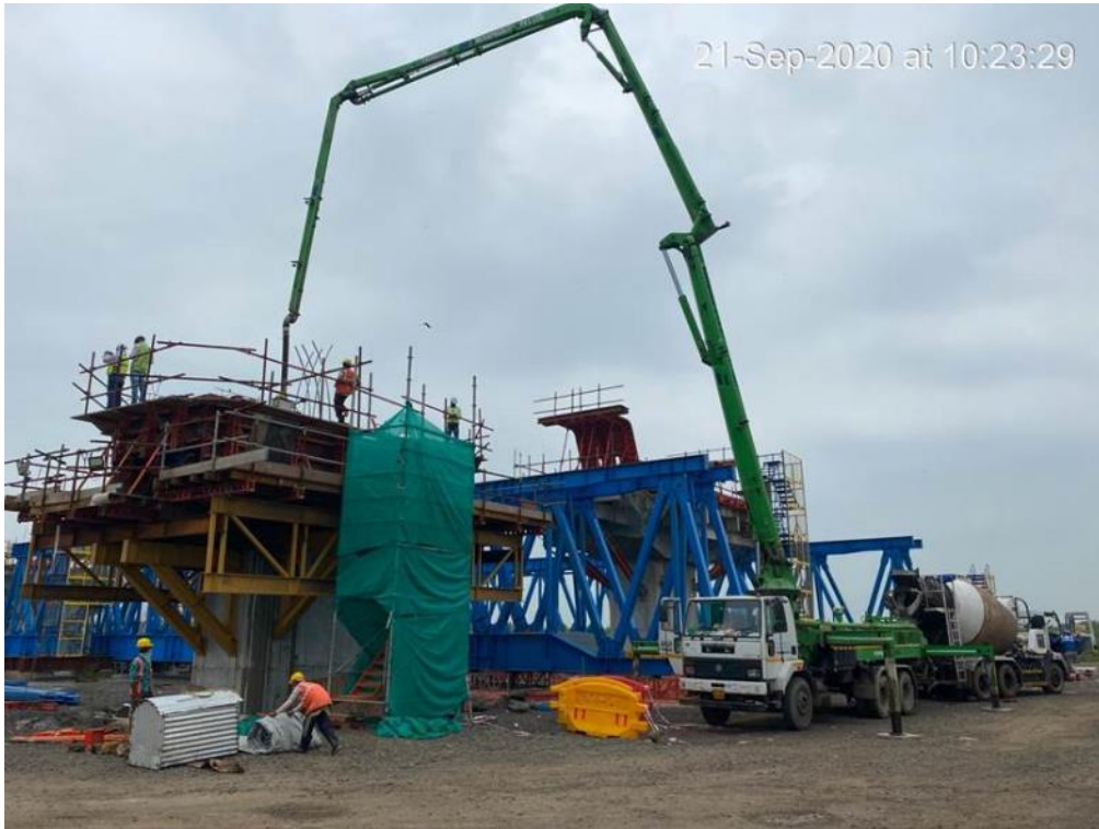
Photo No. 7: Pier Cap concreting at MP 243 LHS in progress
