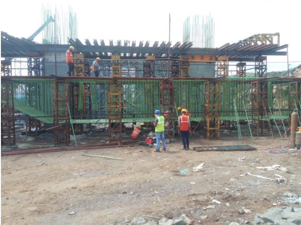
Photo No. 10: RP 03 Portal Pier Cap reinforcement in progress
