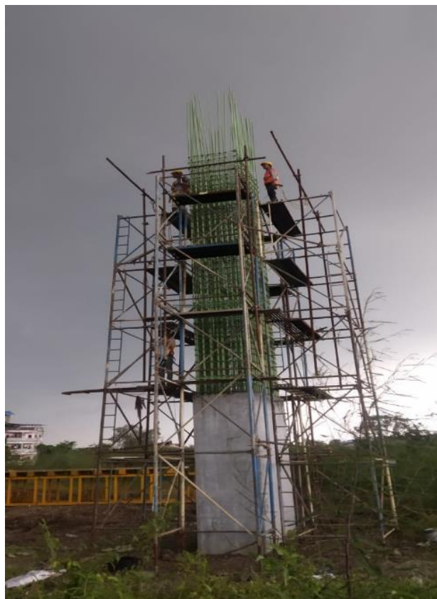
Photo No. 2: JMP-10 (Chirle) Pier reinforcement inspection completed
