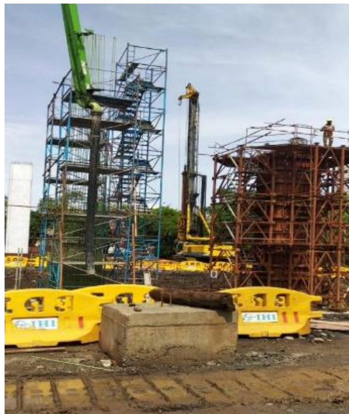
Photo No. 2: EP-15 Pier Concreting – Interchange Area in progress
