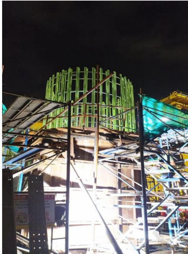
Photo No. 4: AP 39 Pile Cap Concreting in progress
