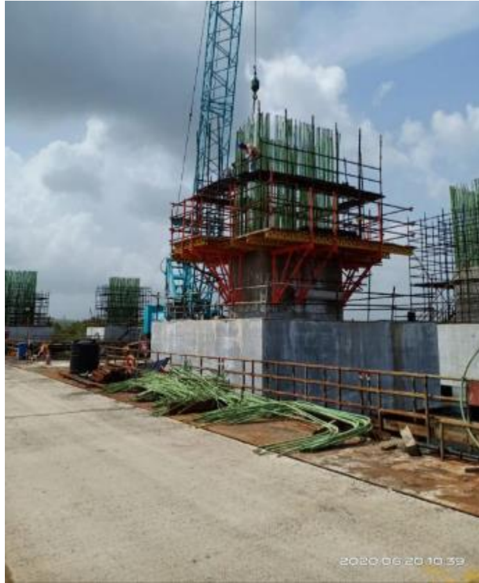
Photo No. 11: Pier reinforcement tying at MP 233 LHS in progress
