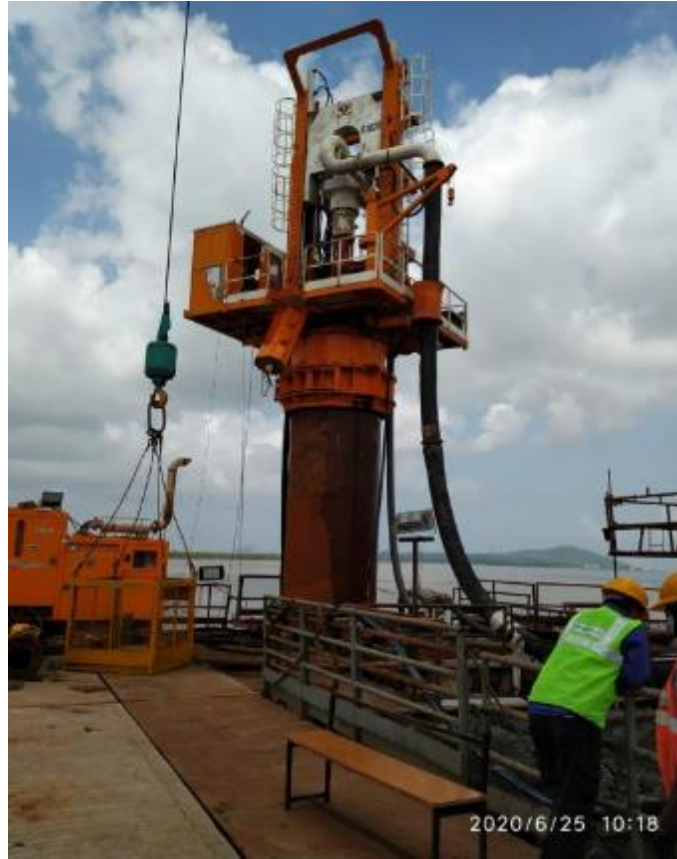
Photo No. 7: Pile drilling at MP 219 RHS in progress
