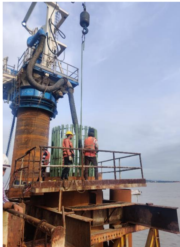
Photo No. 10: MP 126 N2 Top Cage Welding - Marine Area in progress
