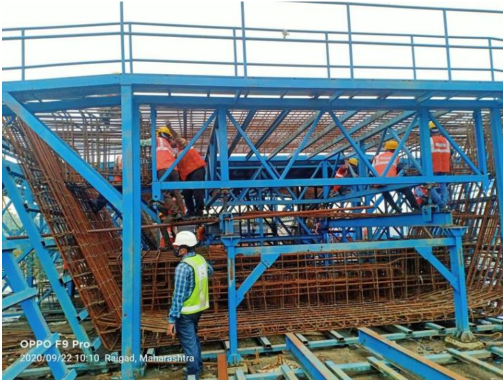
Photo No. 5: Segment Reinforcement Cage Works at Bay-1 in progress
