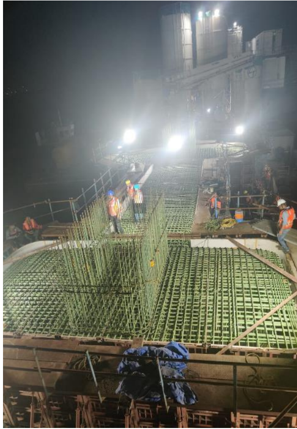
Photo No. 5: MP 108 Pile Cap pre-pour inspection in progress
