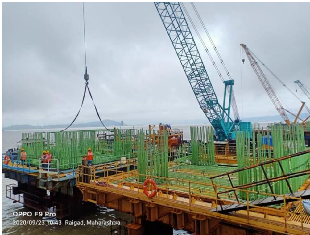
Photo No. 2: Pile Cap Reinforcement Works at MP 216 RHS in progress
