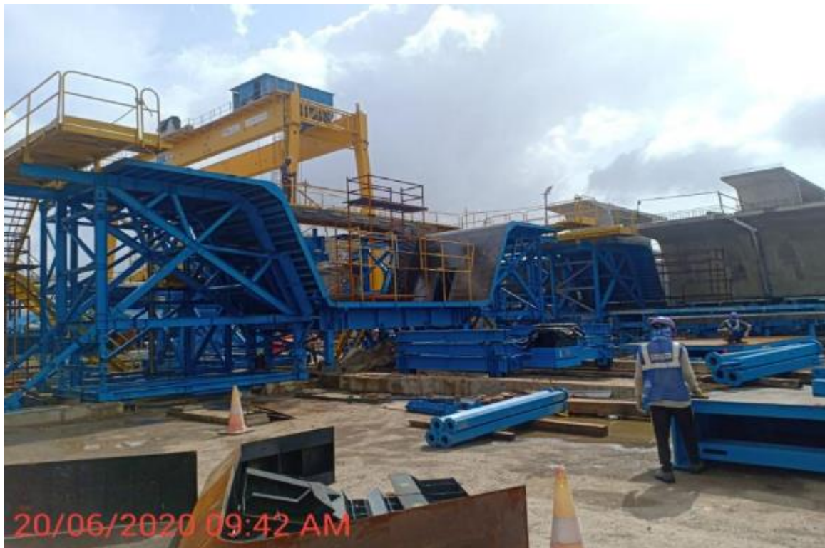
Photo No. 12: Segment Mould erection at Bay-3 in progress
