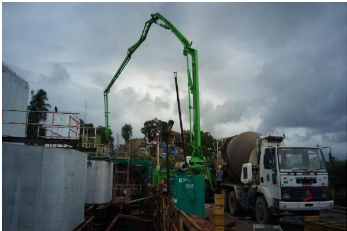
Photo No. 8: MP 02 N Pile Cap Concreting in progress
