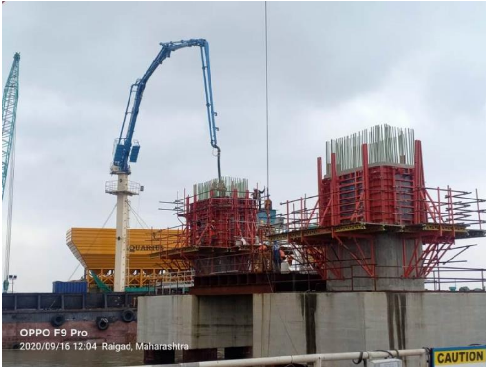
Photo No. 9: Pier final lift concreting at MP 206 RHS in progress
