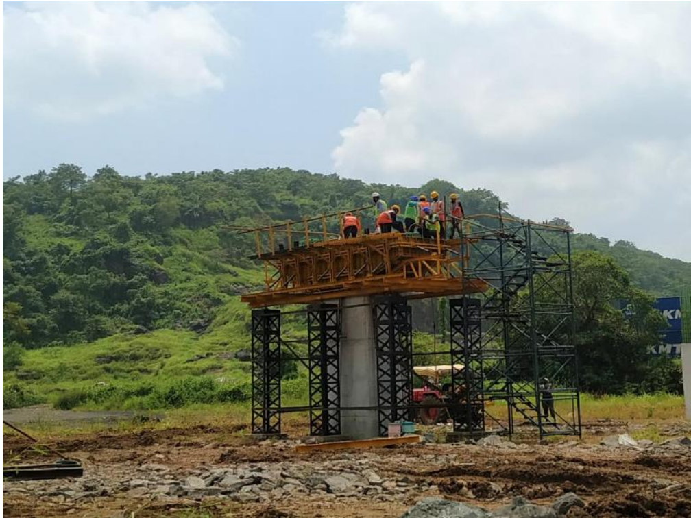
Photo No. 7: Pier Cap PMP-08 (Chirle) Pre-pour inspection completed
