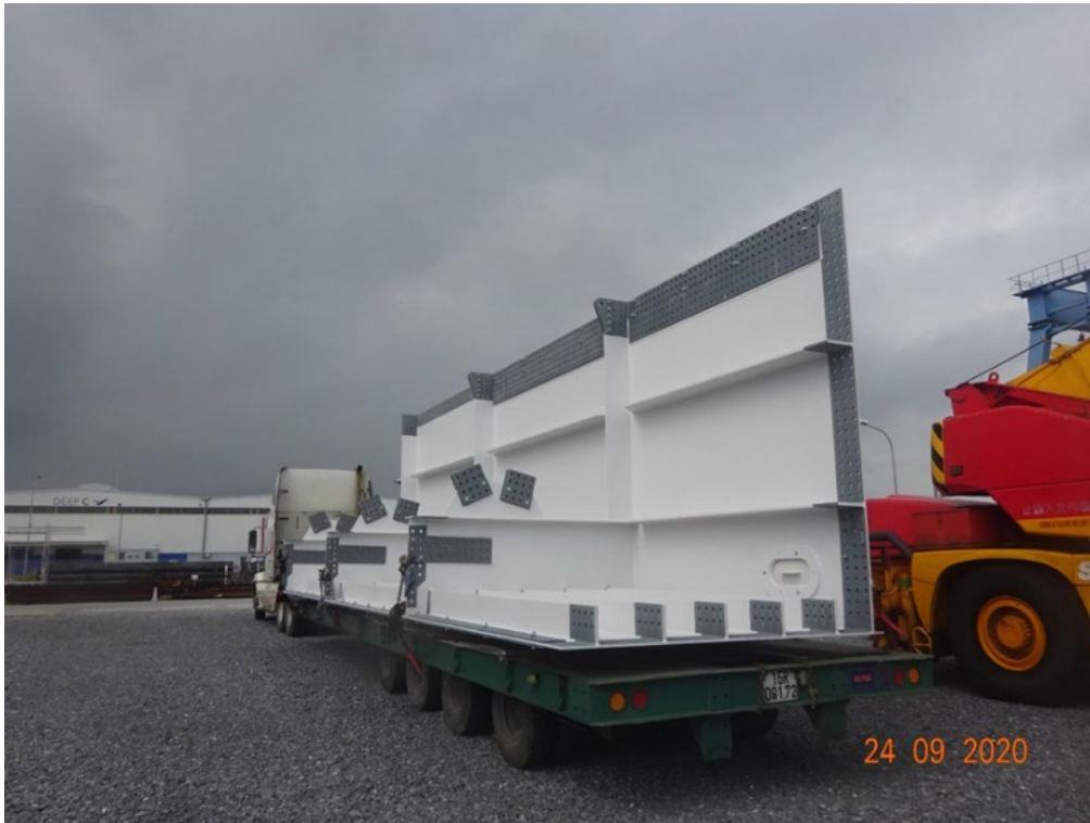
Photo No. 7: Transportation of OSD Girder Bridge P1-OS01-NG Package to Port for Shipment-3 in progress
