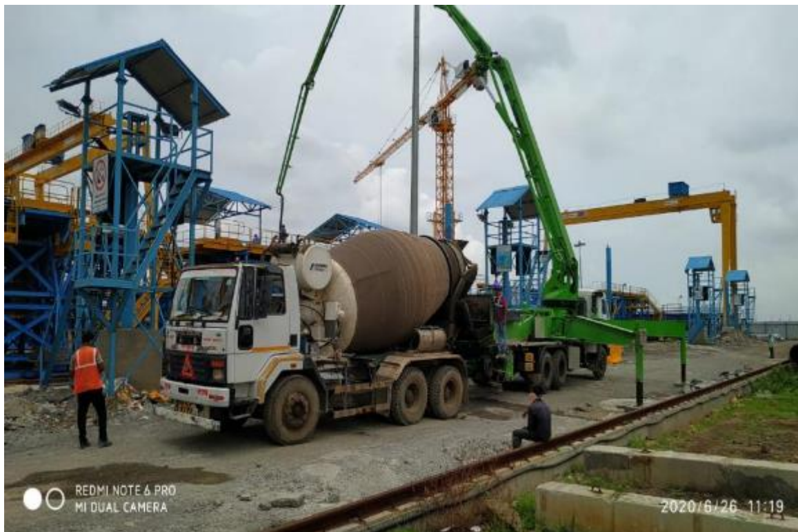
Photo No. 6: Segment concreting at Bay-2 in progress
