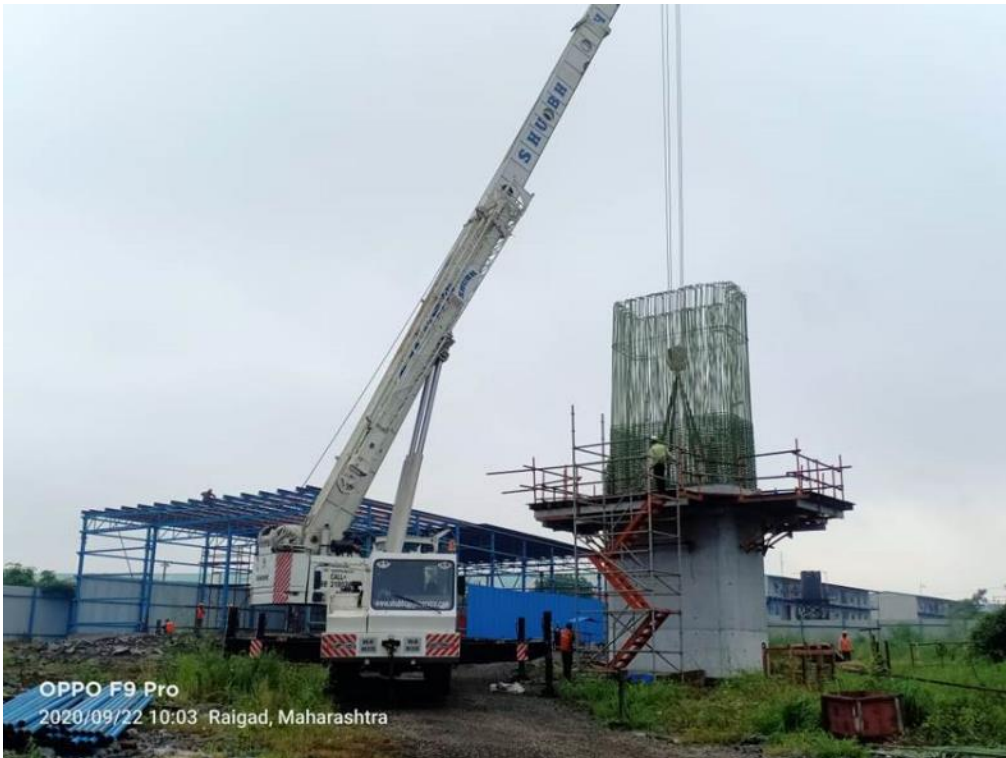
Photo No. 6: Pier Formwork fixing at MP 265 LHS in progress
