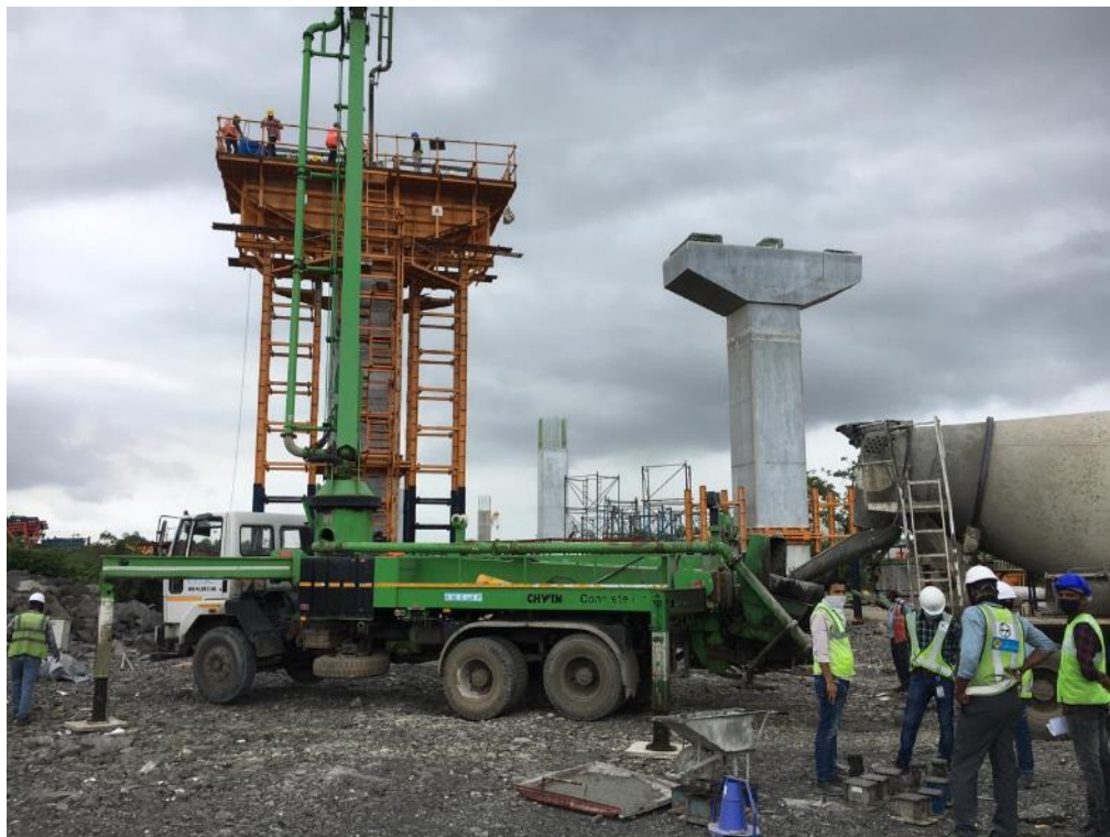
Photo No. 8: RMP 281 Pier Cap concrete pouring in progress
