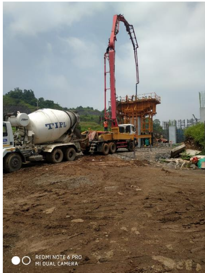
Photo No. 6: JMP02 (Jasai) Pier Cap concreting in progress
