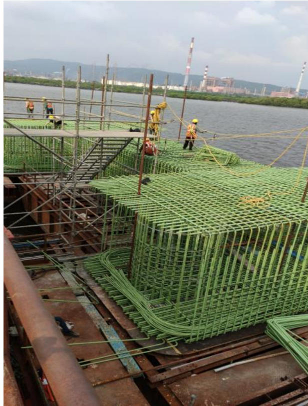
Photo No. 3: MP 43 Pile Cap Bottom Reinforcement Inspections - Intertidal in progress
