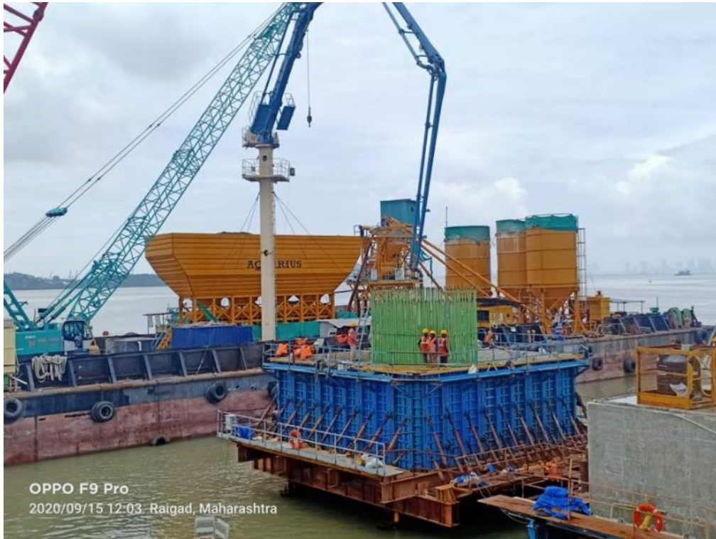
Photo No. 11: Pile Cap concreting at MP 212 RHS in progress
