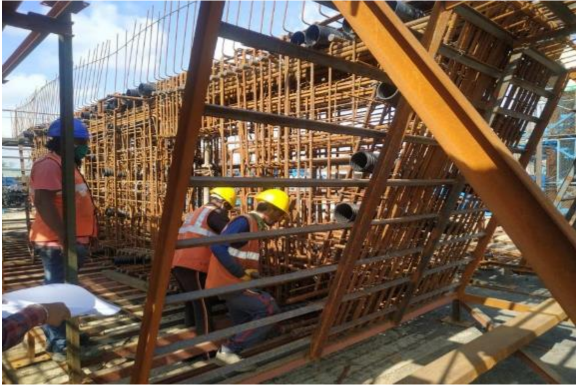
Photo No. 9: Reinforcement inspection for Segment N (15) in progress
