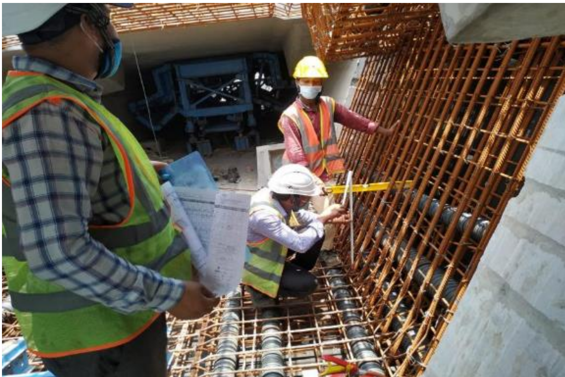
Photo No. 10: Segment Profile checking in progress
