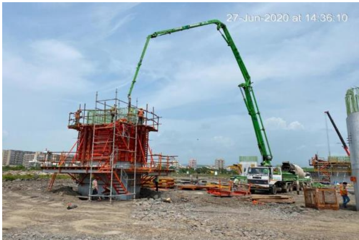
Photo No. 2: Pier final lift concreting at MP 242 LHS in progress
