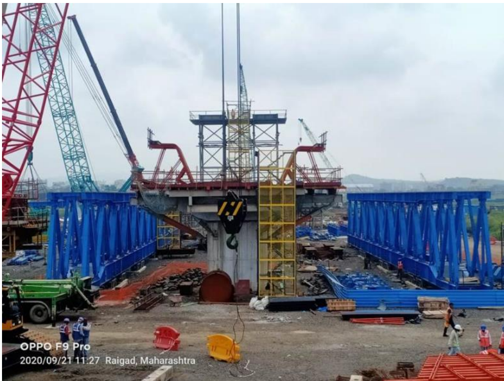
Photo No. 8: LG assembling works in progress
