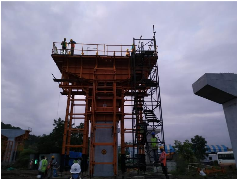
Photo No. 4: LP-06 (Jasai) Pier Cap Pre-pour inspection completed
