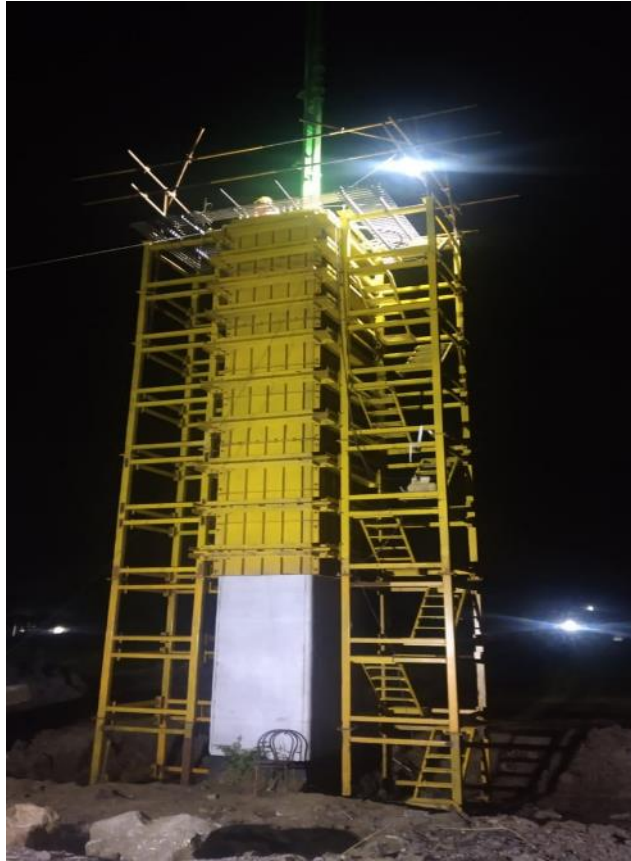
Photo No. 3: MPP12 Pier concrete pouring in progress
