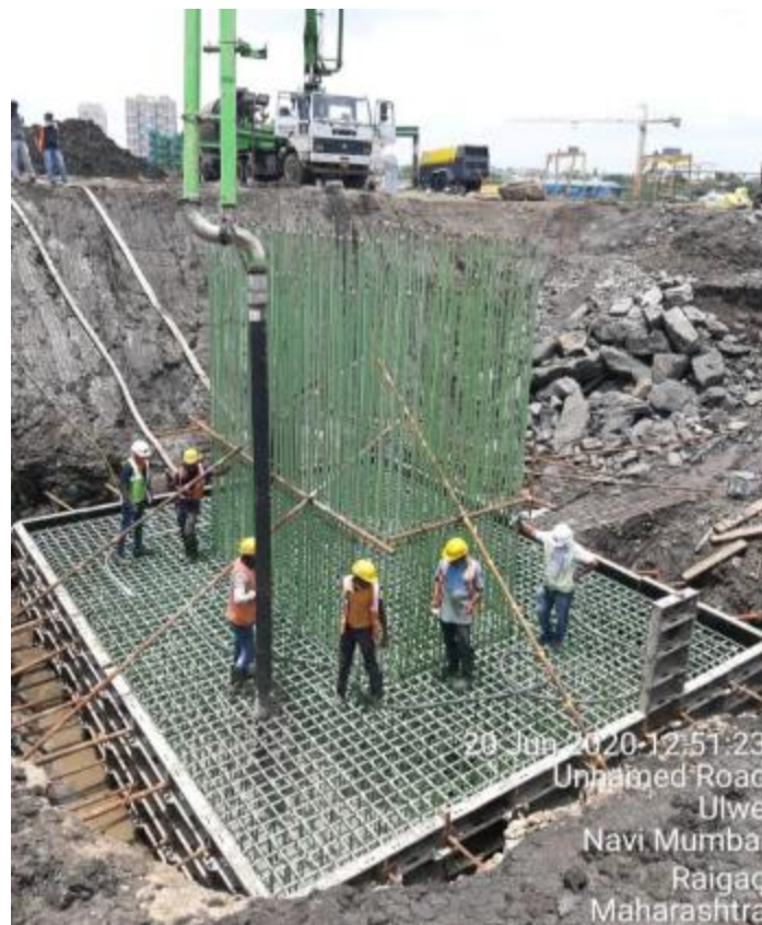
Photo No. 10: Open foundation concreting at MP 251 RHS in progress
