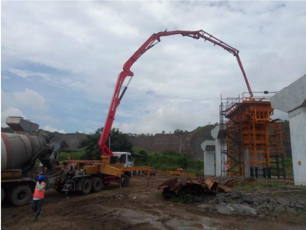
Photo No. 5: LP06 Pier cap concrete pouring in progress
