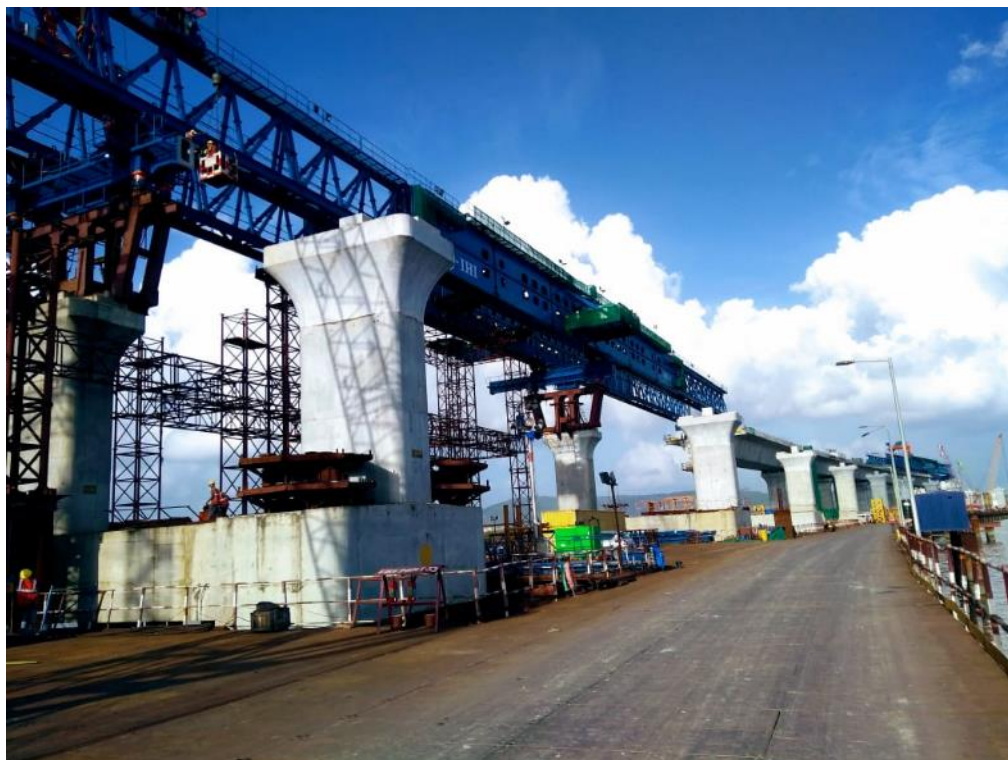
Photo No. 2: LG-2 Erection - Intertidal Section in progress
