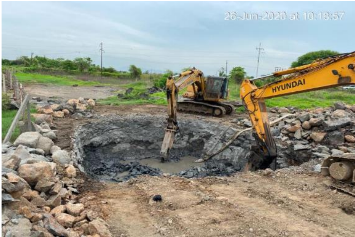
Photo No. 5: Excavation at Open Foundation MAA2 in progress
