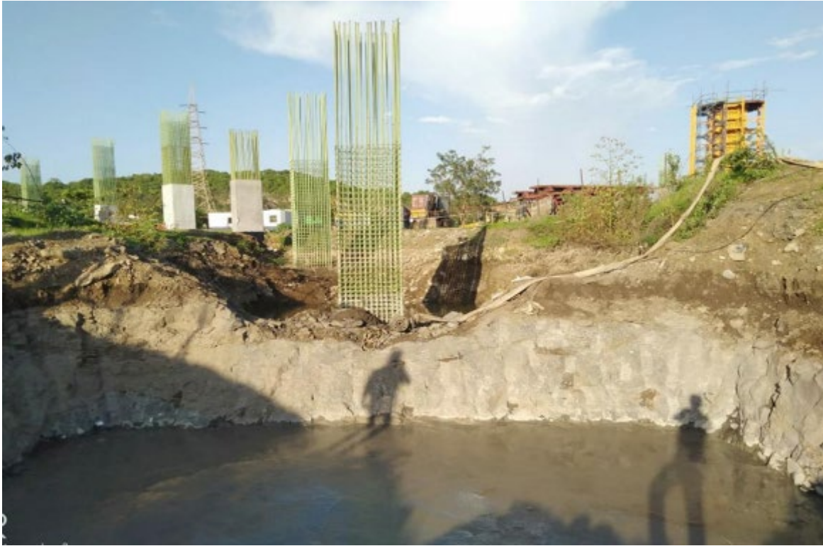
Photo No. 1: PCC for Foundation No. MPP-05 (Chirle) completed
