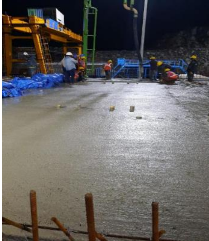
Photo No. 11: Segment concrete pouring at bay 2, precast yard in progress
