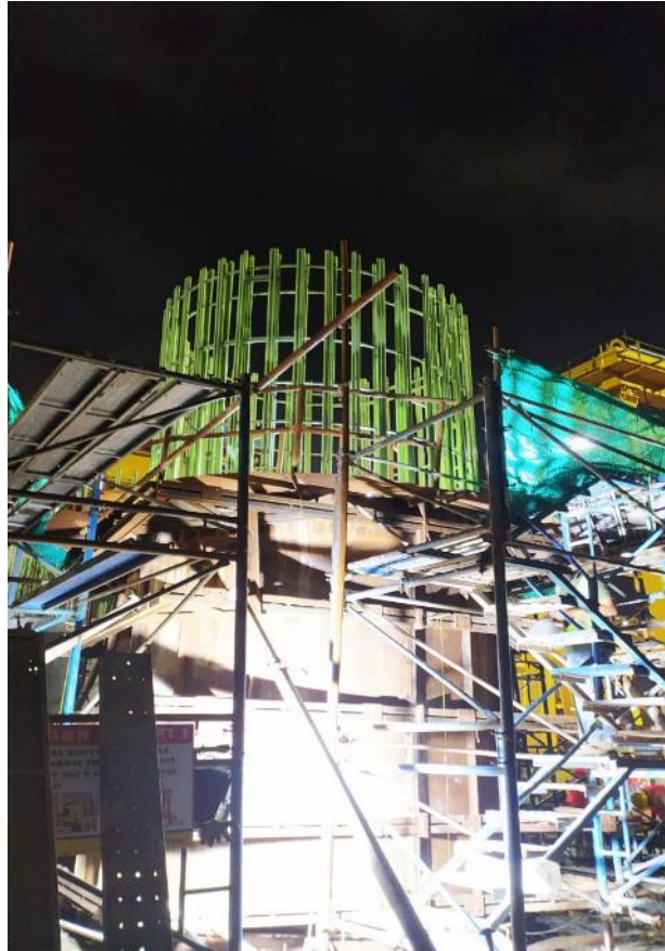
Photo No. 11: AP 39 Pile Cap concreting in progress
