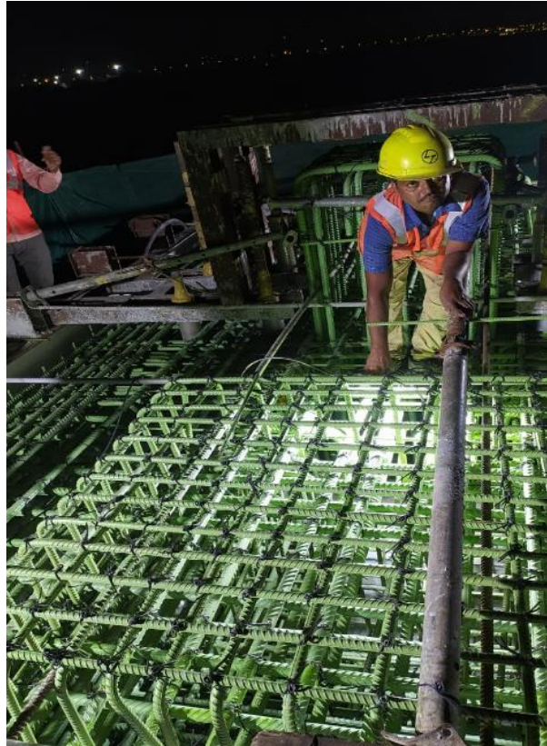
Photo No. 9: MP 19 N Pier Cap Pre-Pour checking in progress
