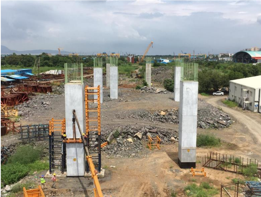
Photo No. 9: A View taken from RMP 281 Pier
