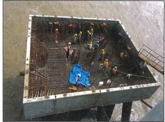
Figure 19: Typical Pile Cap Shell
