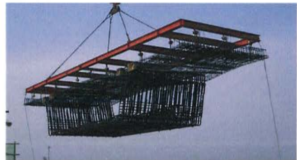
Figure 8: Rebar Cage Handling
