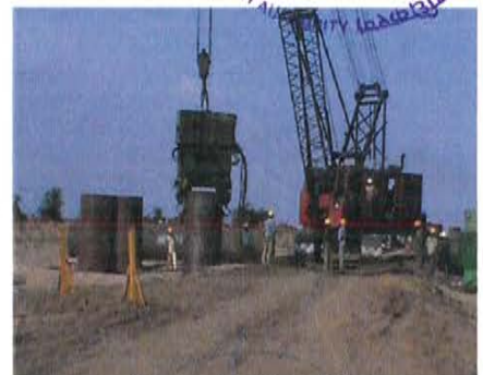
Figure 13: Liner Driving
