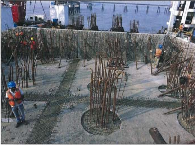
Figure 19: Typical Pile Cap Shell
