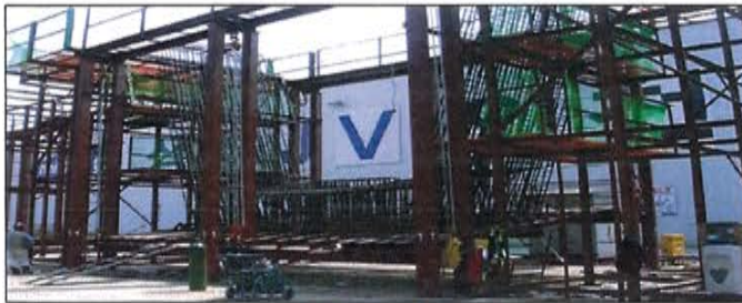
Figure 7: Typical Rebar Jig
