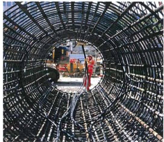
Figure 15: Typical Pile Reinforcement Cage
