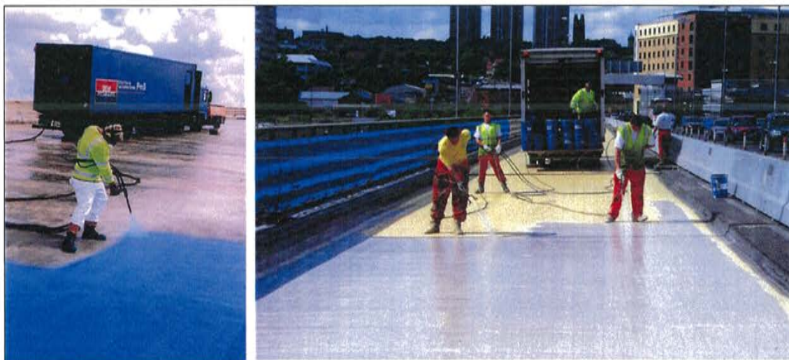
Figure 31: Waterproofing Application
