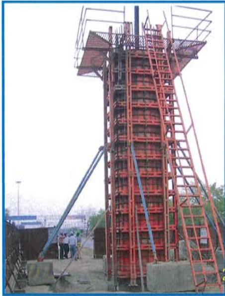
Figure 20 Pier Formwork
