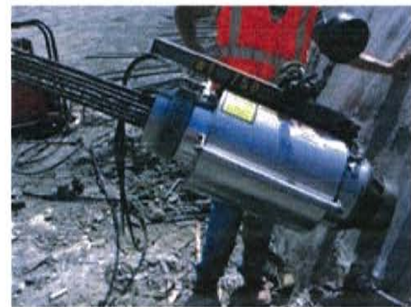
Figure 26: Stressing of Tendon
