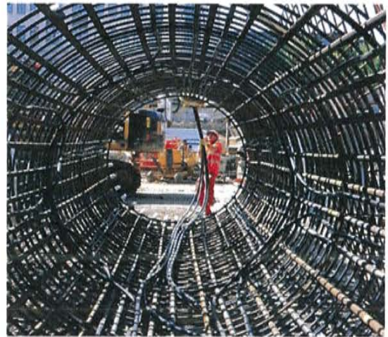
Figure 16 : Pile Reinforcement Cage
