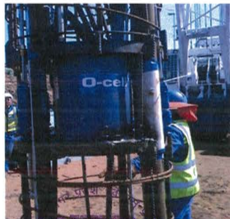
Figure 17: Typical O-cell pile Load test arrangement
