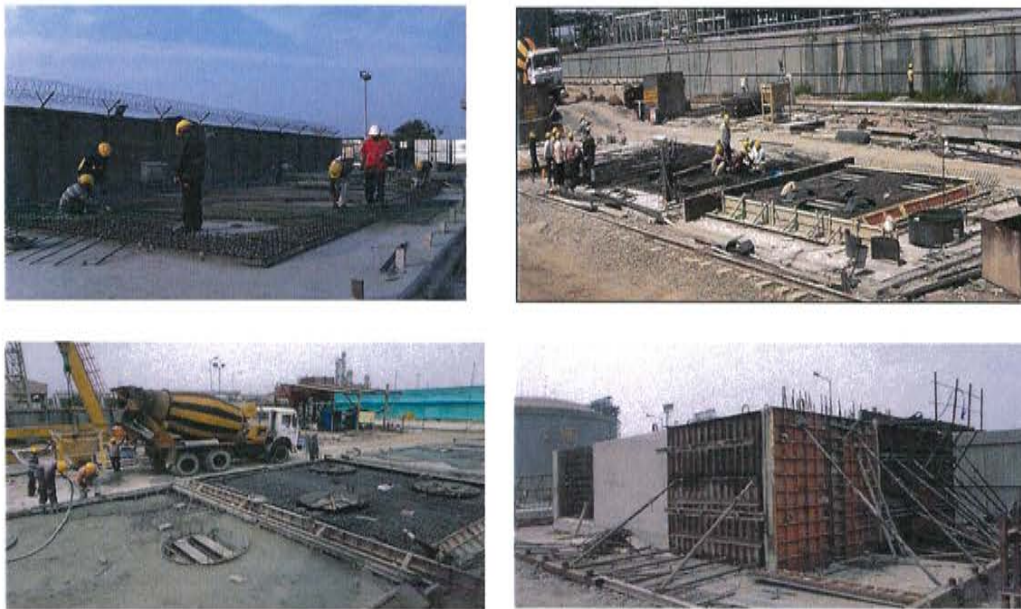
Figure 18: Photographs of Pile Cap Shell Pre-casting Work
