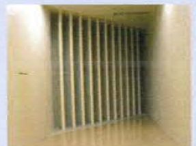
• Corner Vane flow deflector at corner
