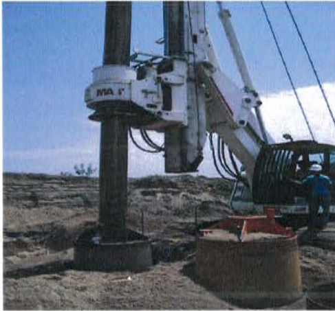
Figure 14: Boring with Hydraulic Rig
