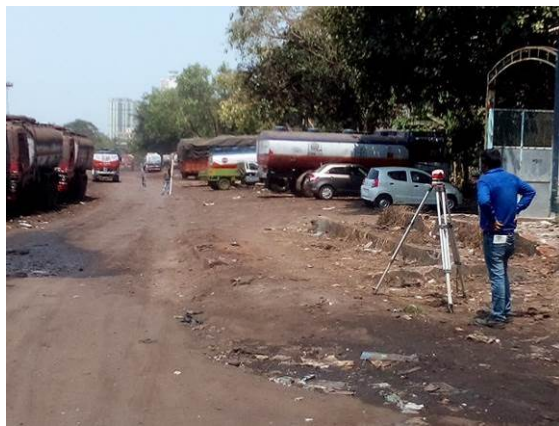
Topographic survey work at Seweri site
