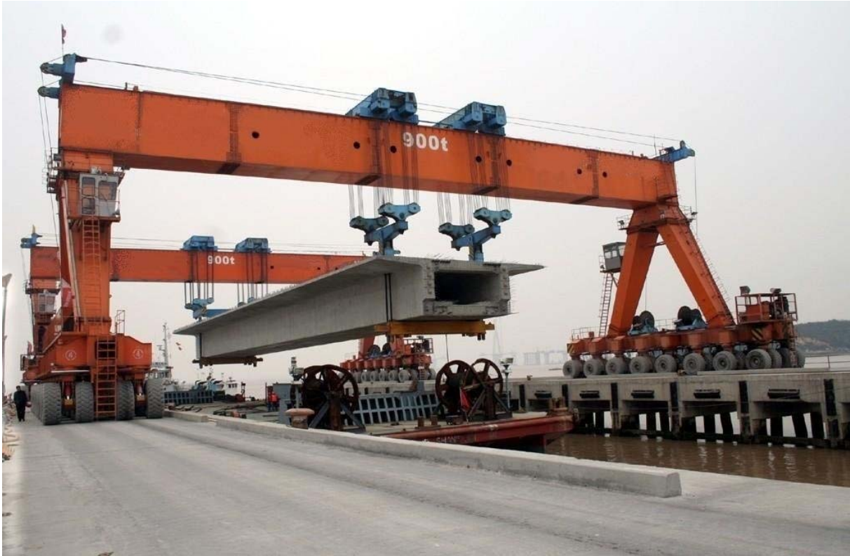
Figure 7.2.17 Full Span Erection Method (Using Gantry Crane)
