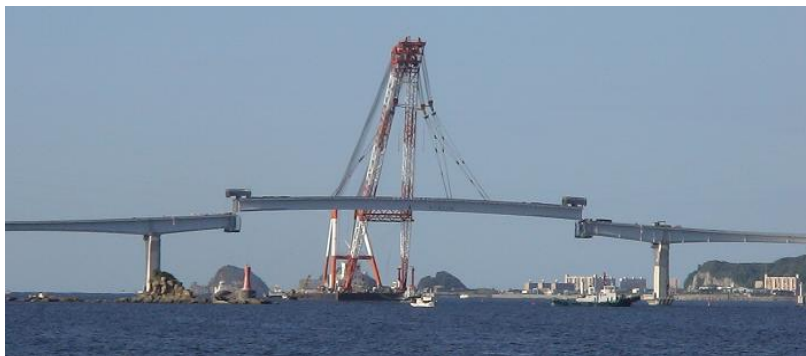
Figure 7.2.15 Large Block Erection Method Using Floating Crane
