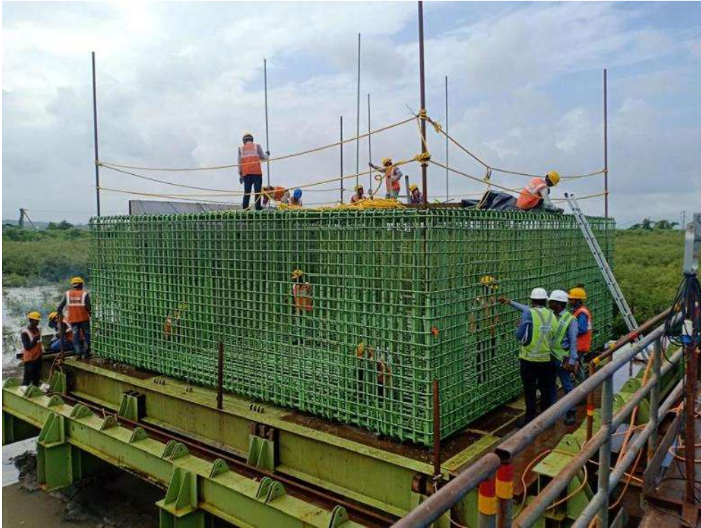
Photo No. 3: Pile Cap Reinforcement Works at MP 238 RHS in progress
