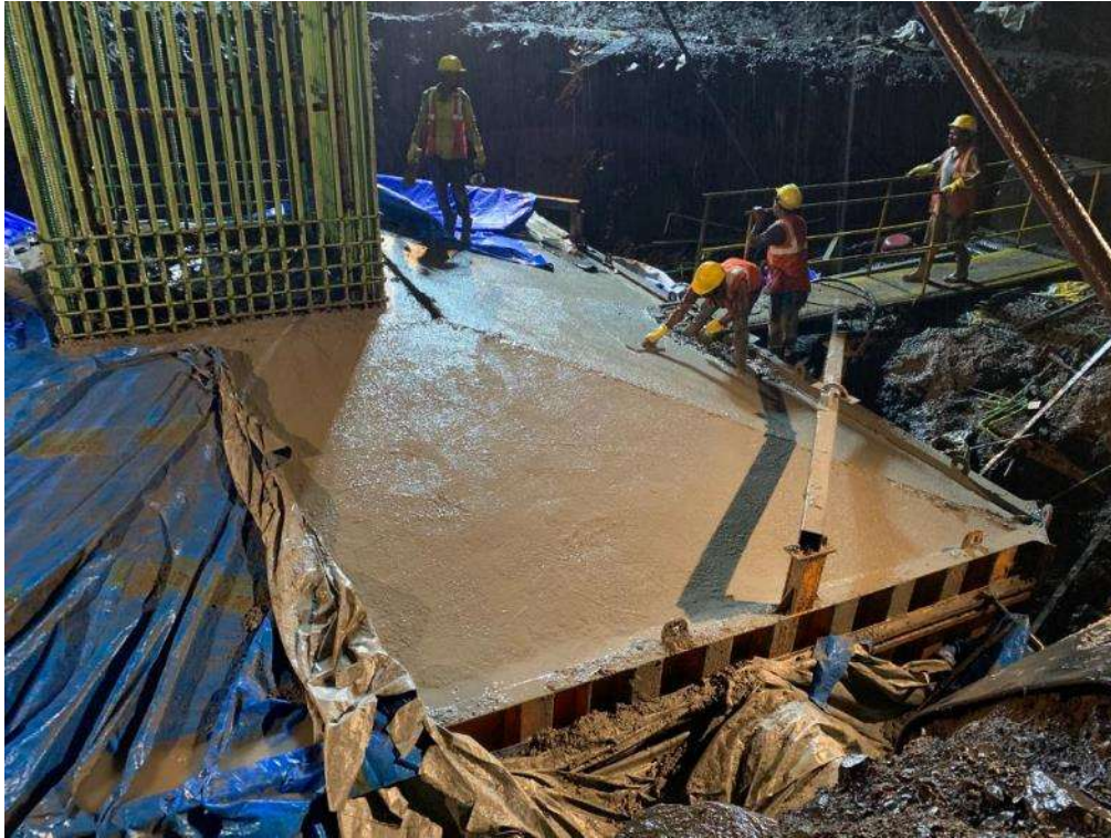
Photo No. 3: Foundation casting at JMP 13 Chirle location is in progress
