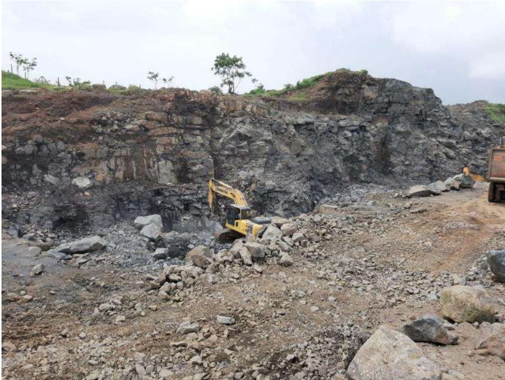
Photo No. 7: Excavation at At-Grade area at CH 19+750 is in progress
