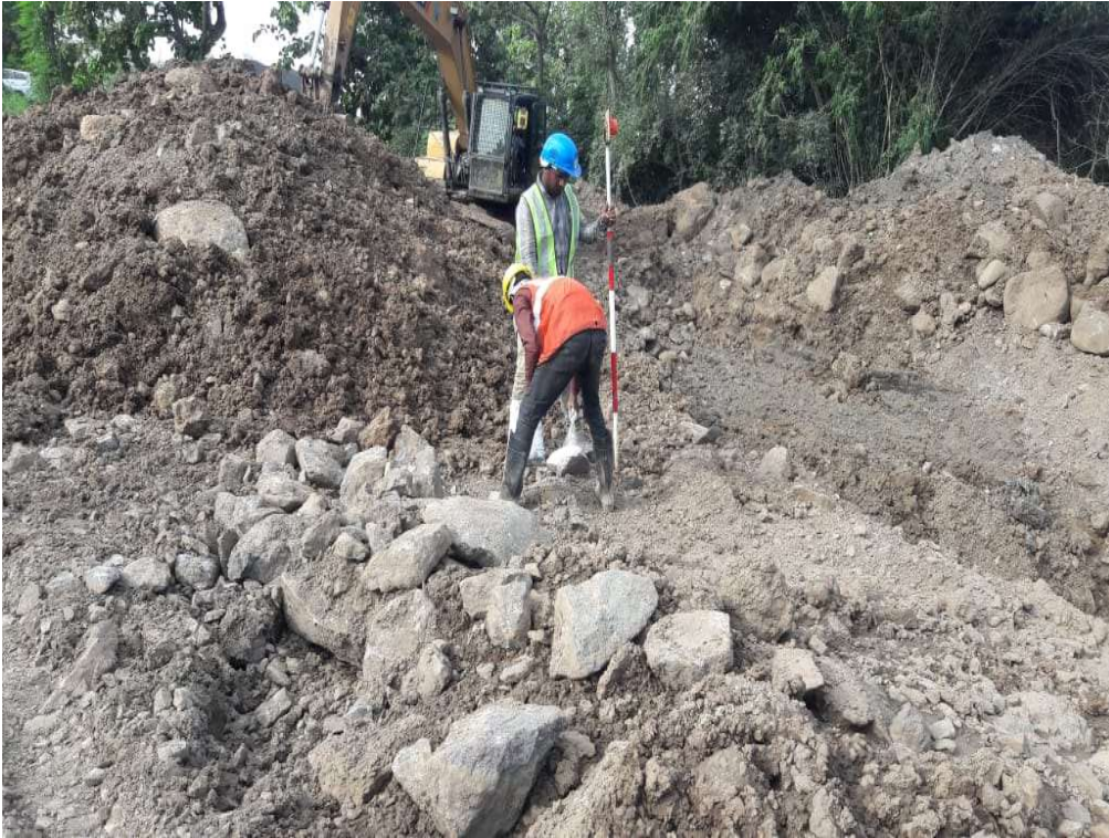
Photo No. 5: OGL Survey at LP02 RHS location is in progress
