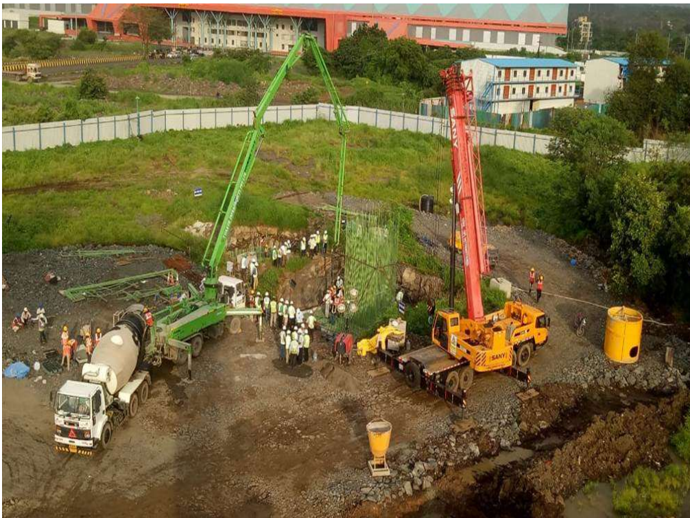
Photo No. 10: Open foundation Concreting at MP 266 RHS in progress
