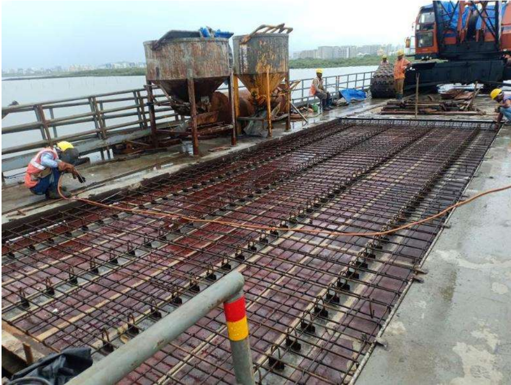
Photo No. 9: Composite Slab formwork for Span 78 in progress
