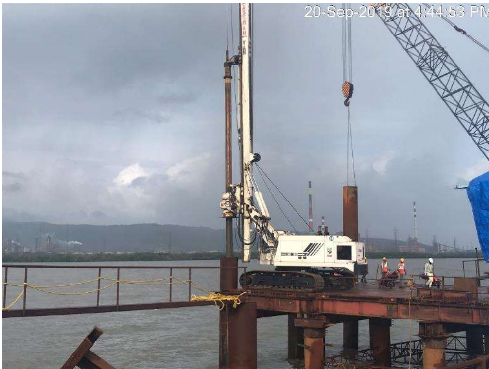
Photo No. 10: Pile Boring at Finger MP-25 is in progress
