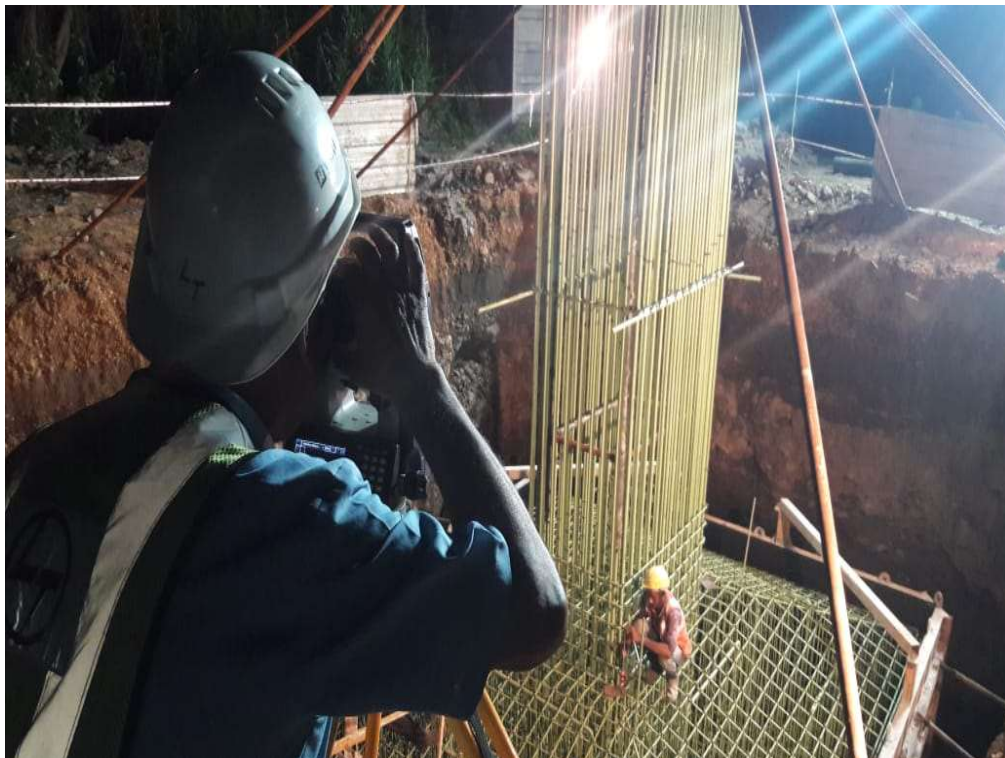
Photo No. 4: Survey for Pre-pour checking at PMP 07 in progress
