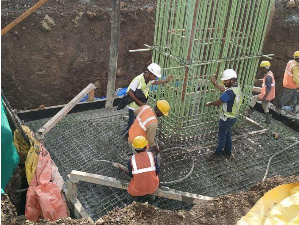
Photo No. 1: Foundation casting at PMP 11 Chirle location is in progress
