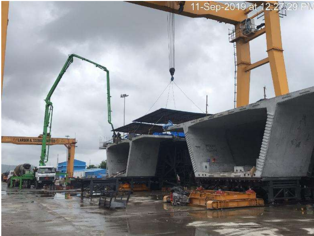
Photo No. 7: Casting of Segment No. 82-83 NS3
