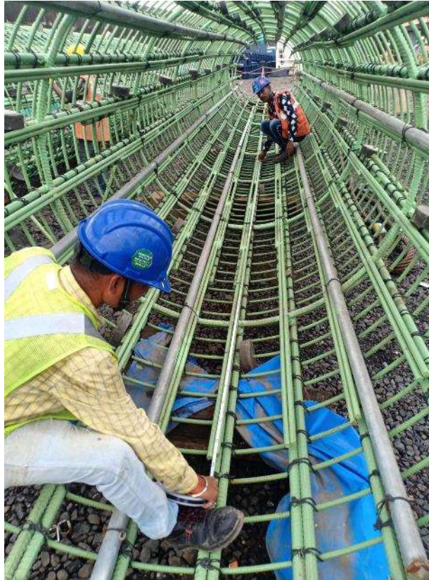
Photo No. 11: Pile Reinforcement Cage inspection at MP 239/01 LHS in progress
