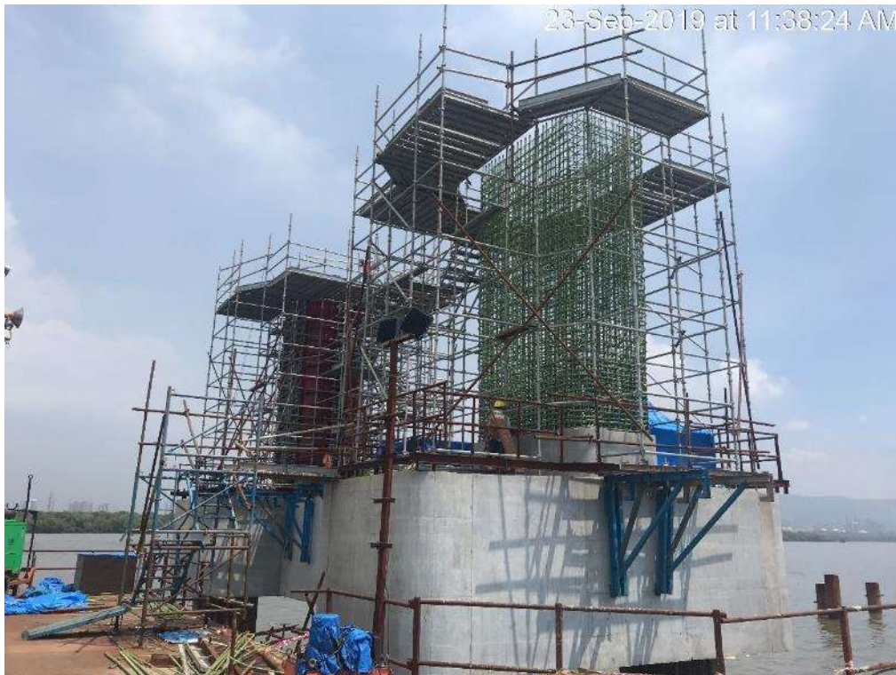
Photo No. 1: Pier Reinforcement at MP-17 N is in progress
