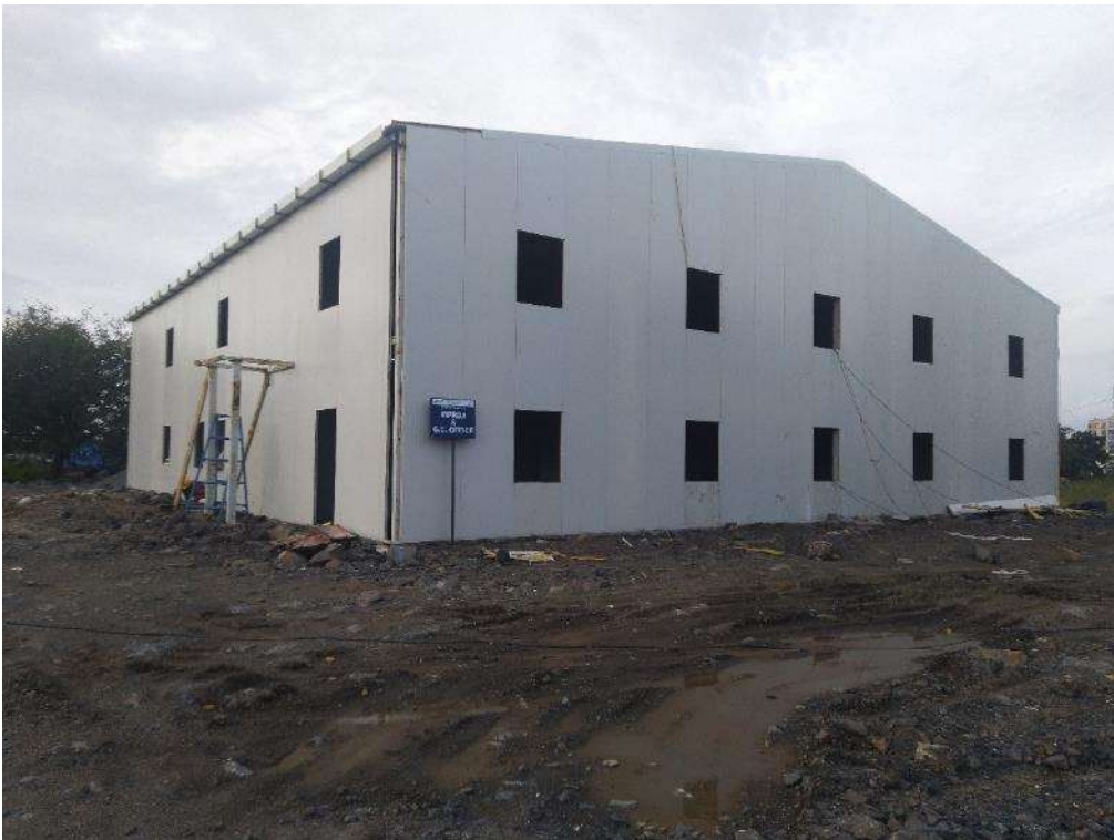
Photo No. 12: Employer's Office construction works in progress
