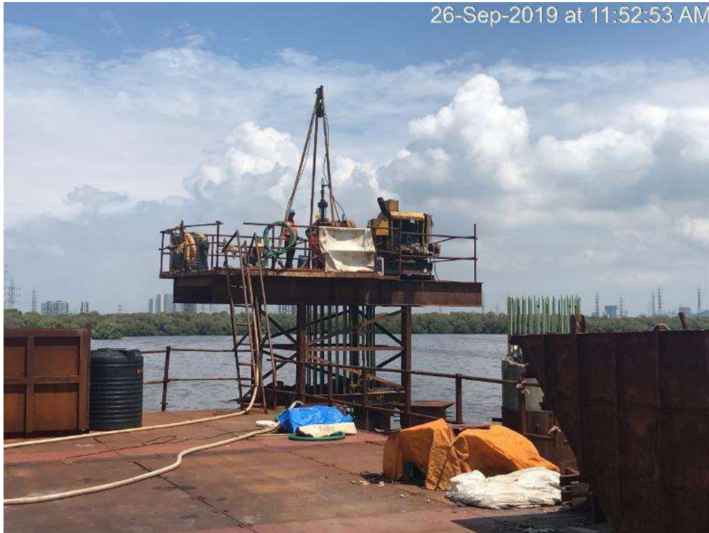
Photo No. 11: Core drilling at MP 19 location is in progress
