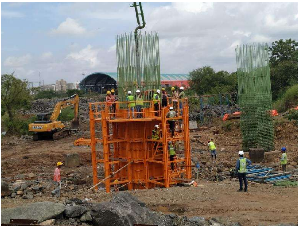
Photo No. 2: Pier casting at RMP 278 location is in progress
