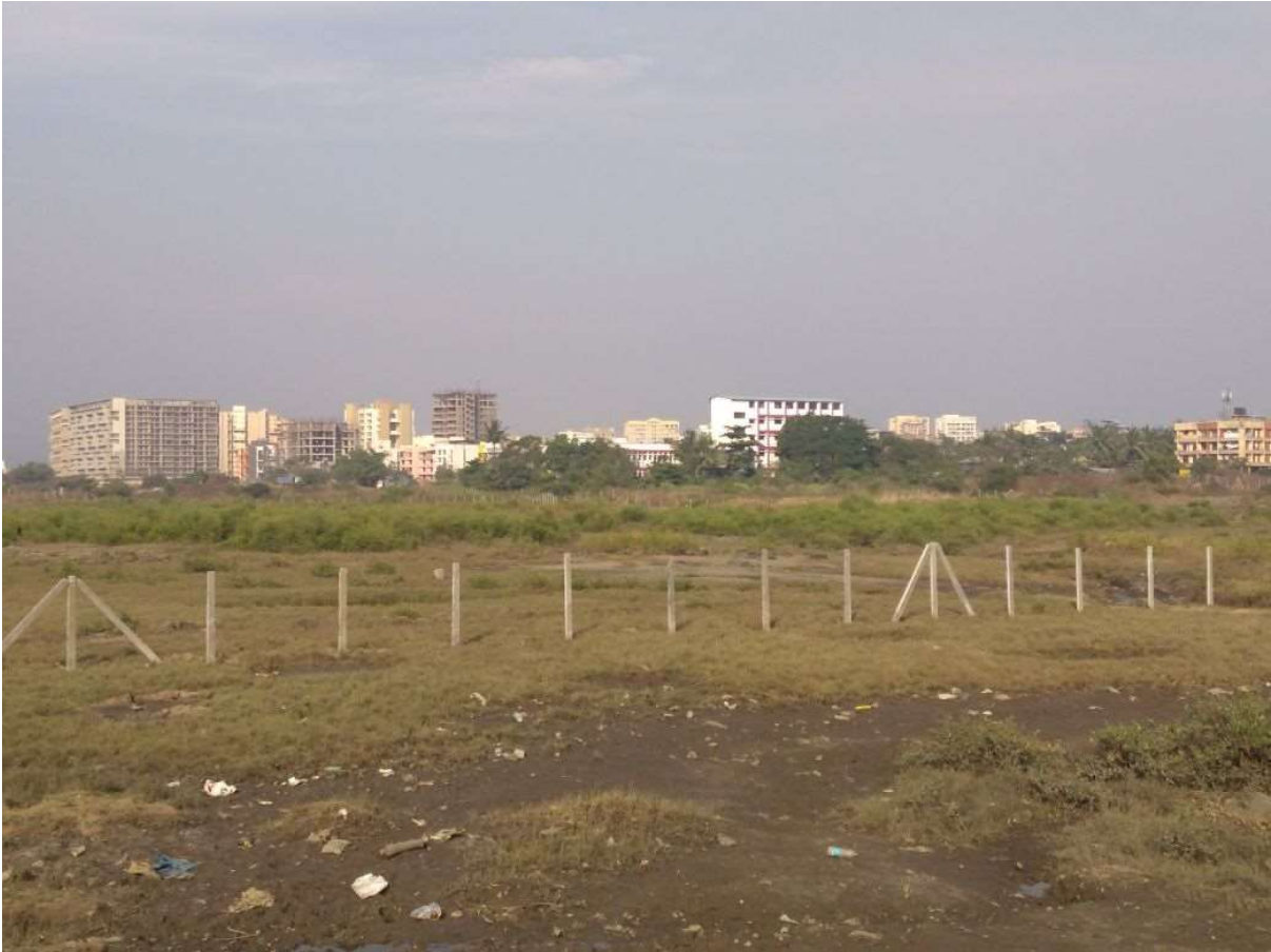
Material for Package 2 Casting Yard Fencing Site 24/11/2017
