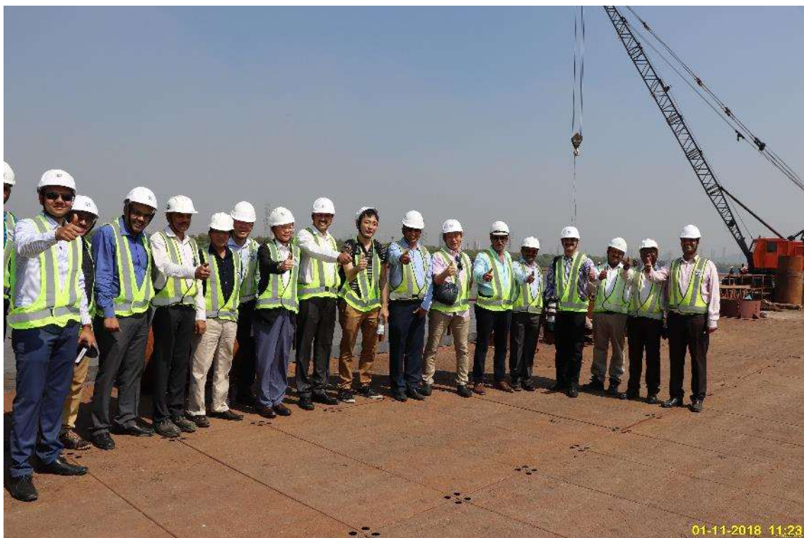
Photo No. 2: JICA Site visit – Package 1 dated 1 st November 2018
