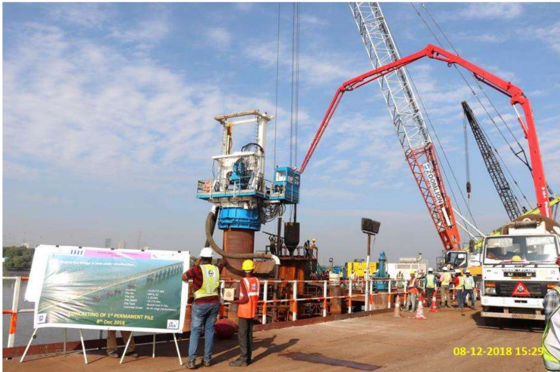
Photo No. 1: Permanent Pile Casting at MP6 Location in progress
