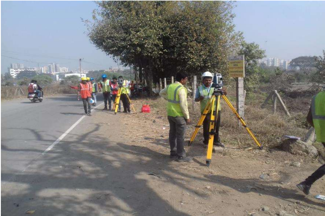
Photo No. 25: OGL Survey at CH 18+200 in progress
