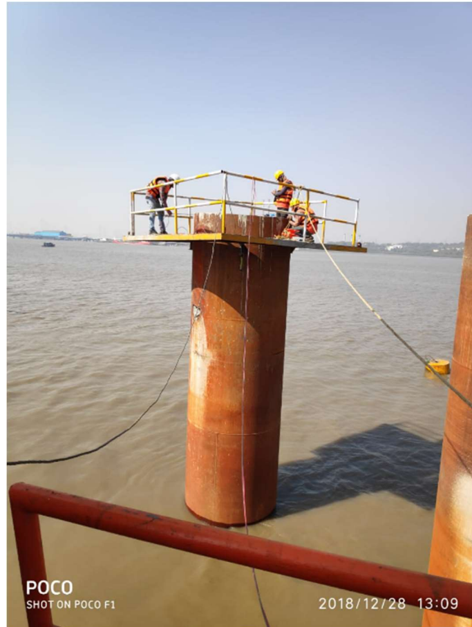
Photo No. 11: Cross-hole Sonic Test at MP 95 Location in progress
