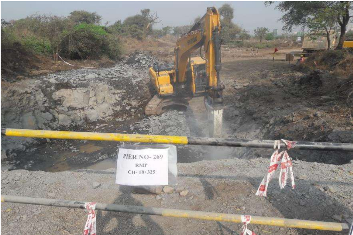
Photo No. 28: Excavation work at Pier No 269 RMP (CH 18+325) in progress
