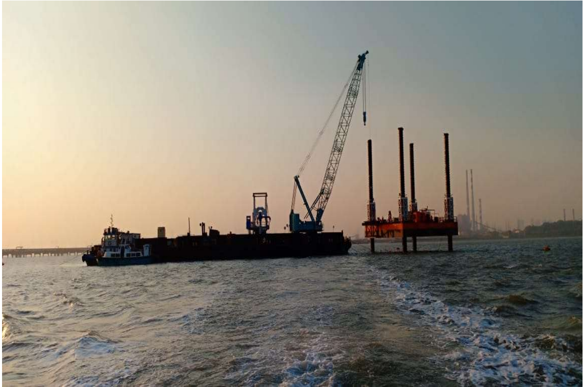
Photo No. 9: Jack-up Barge installation at MP 95 location in progress
