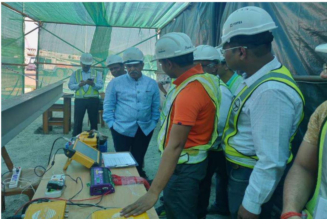
Photo No. 8: Bi-directional Pile Load test monitoring at AP 42 B location
