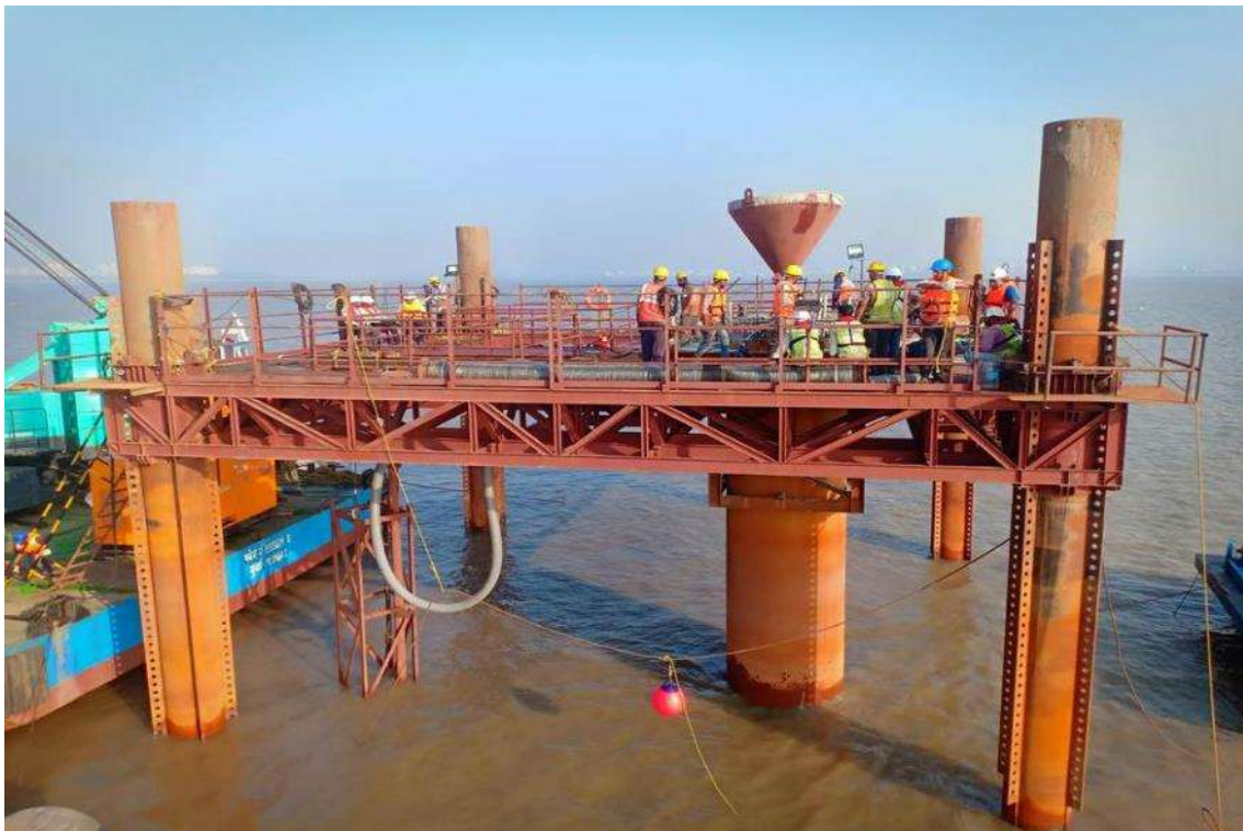
Photo No. 22: Test Pile Concreting Works in progress
