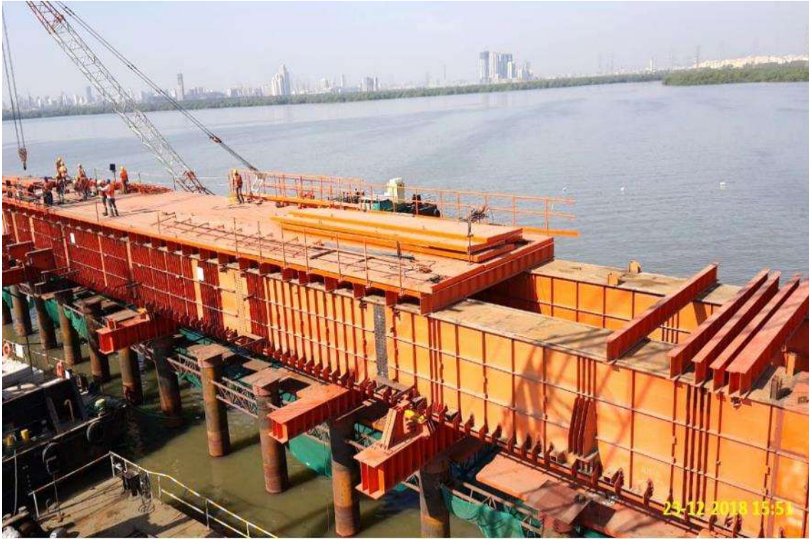
Photo No. 3: Piling Gantry Assembly Works at MP43 Location in progress
