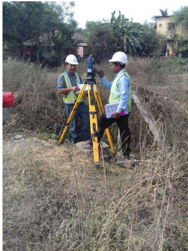
Photo No. 26: Survey Works (Traversing) at Point S1 in progress
