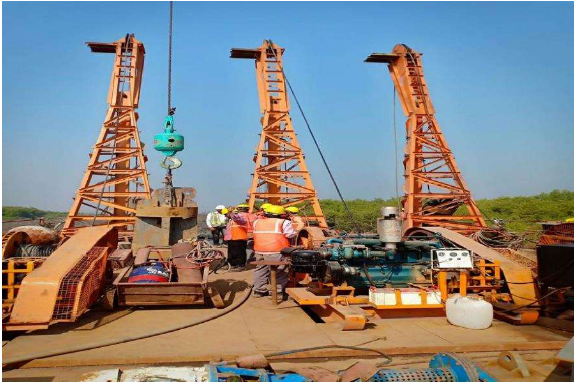
Photo No. 17: Temporary Access Bridge (TAB) Piling works in progress
