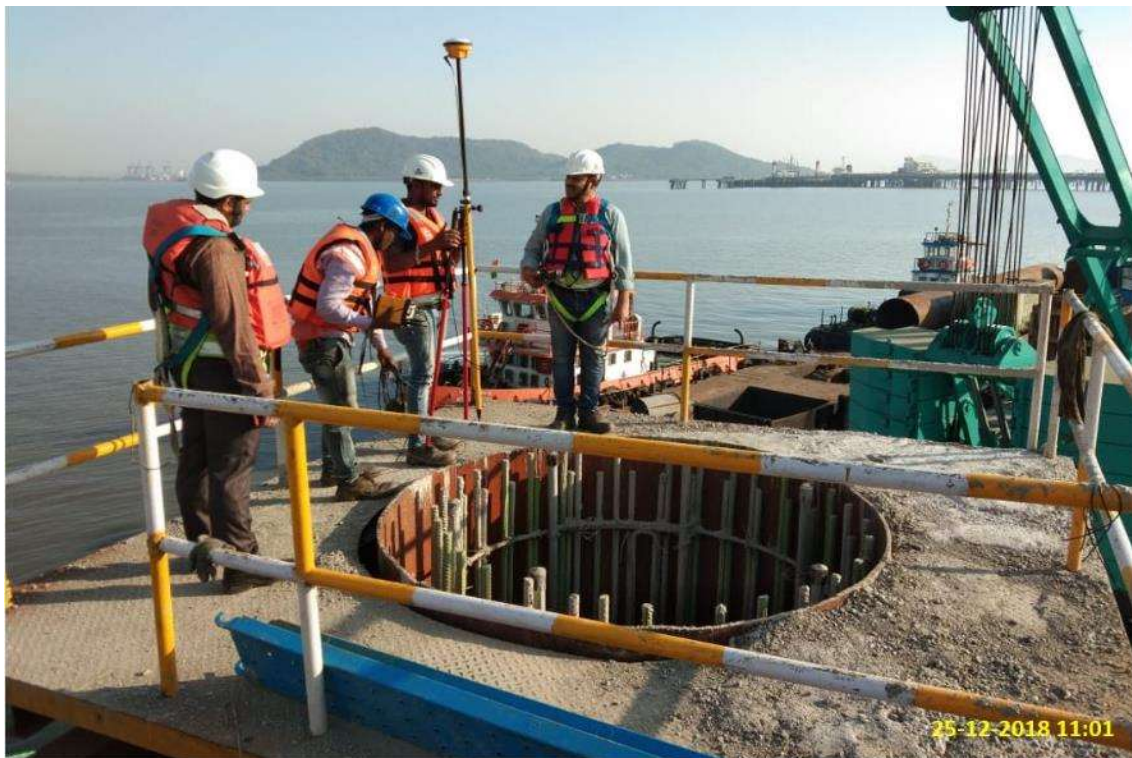
Photo No. 12: Marine Piling Survey Works in progress
