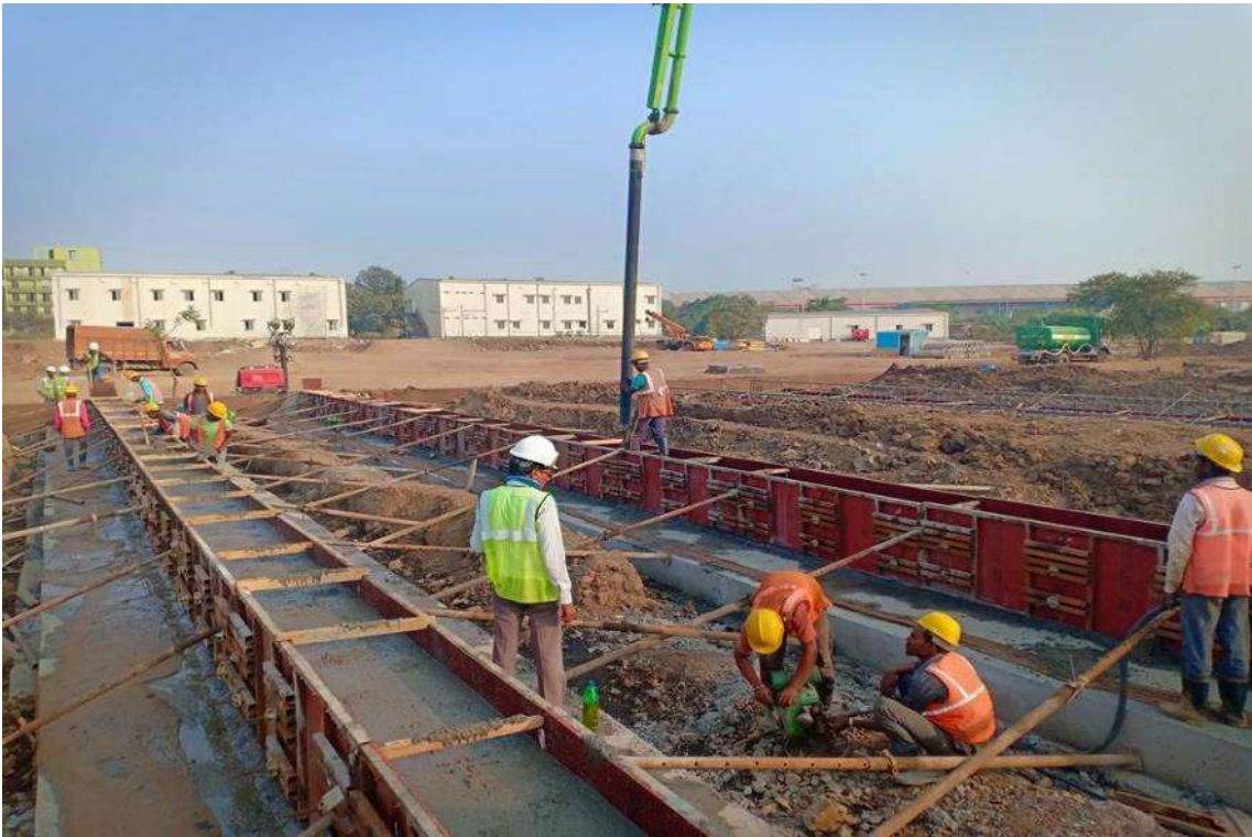
Photo No. 23: Bay-1 Segment Stacking Foundation concrete in progress
