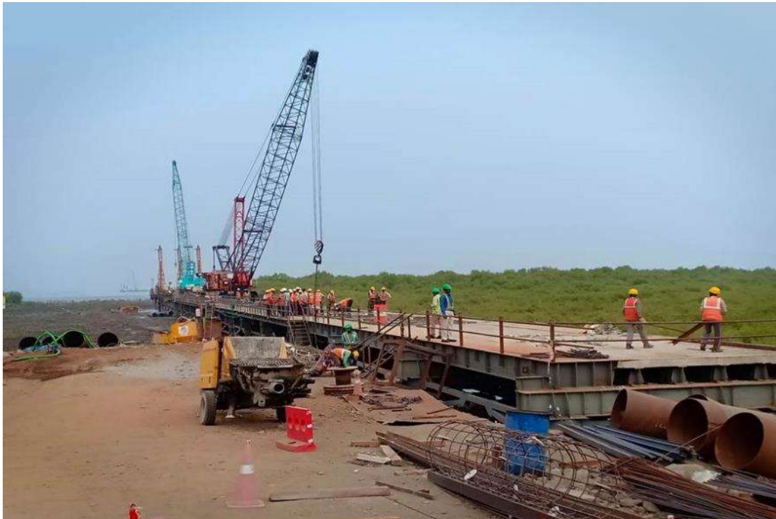
Photo No. 15: Temporary Access Bridge (TAB) Decking works in progress
