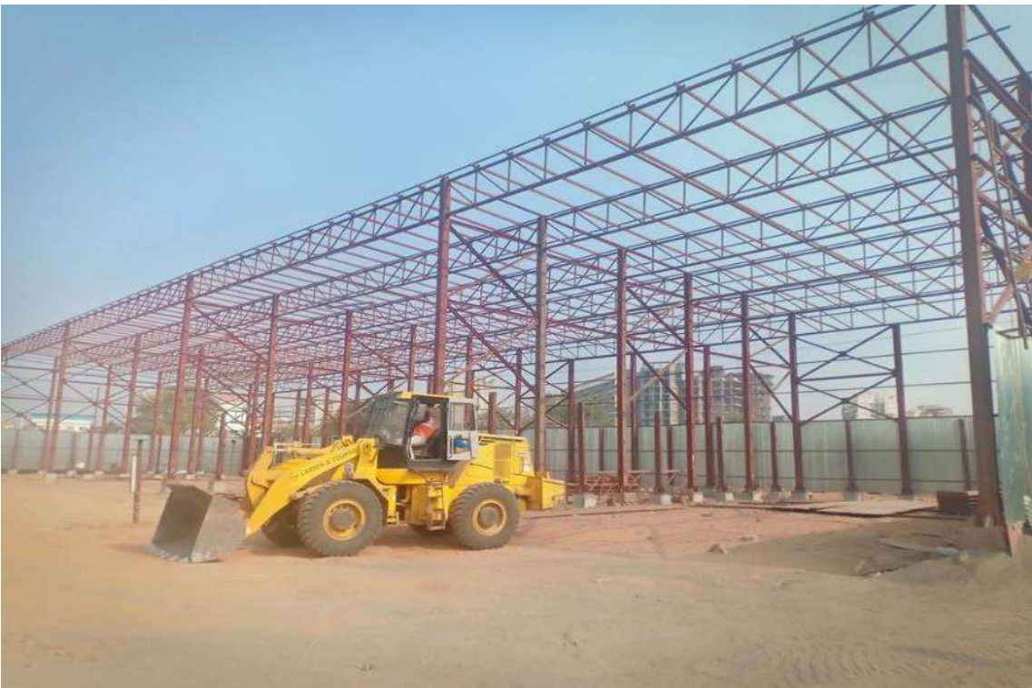
Photo No. 24: Aggregate Shed Construction Works in Progress
