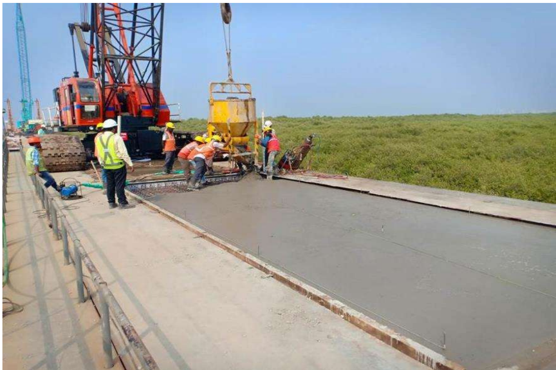
Photo No. 18: TAB - Composite Slab Concreting Works in progress
