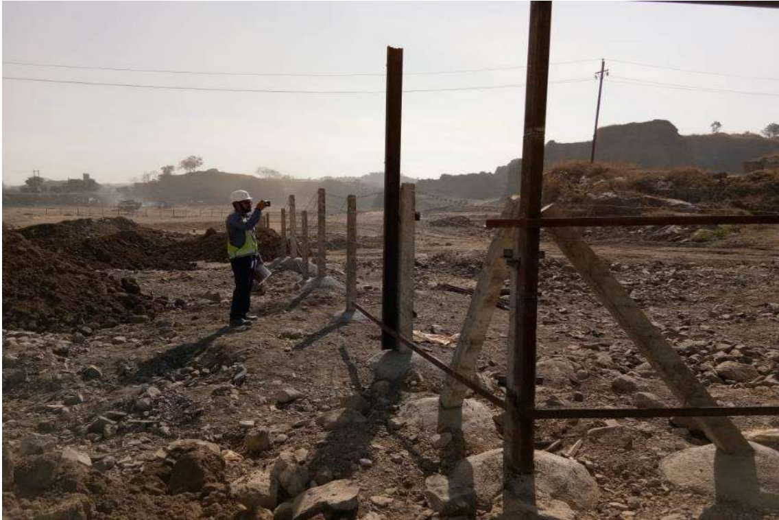
Photo No. 27: Fencing Works at Casting Yard in progress
