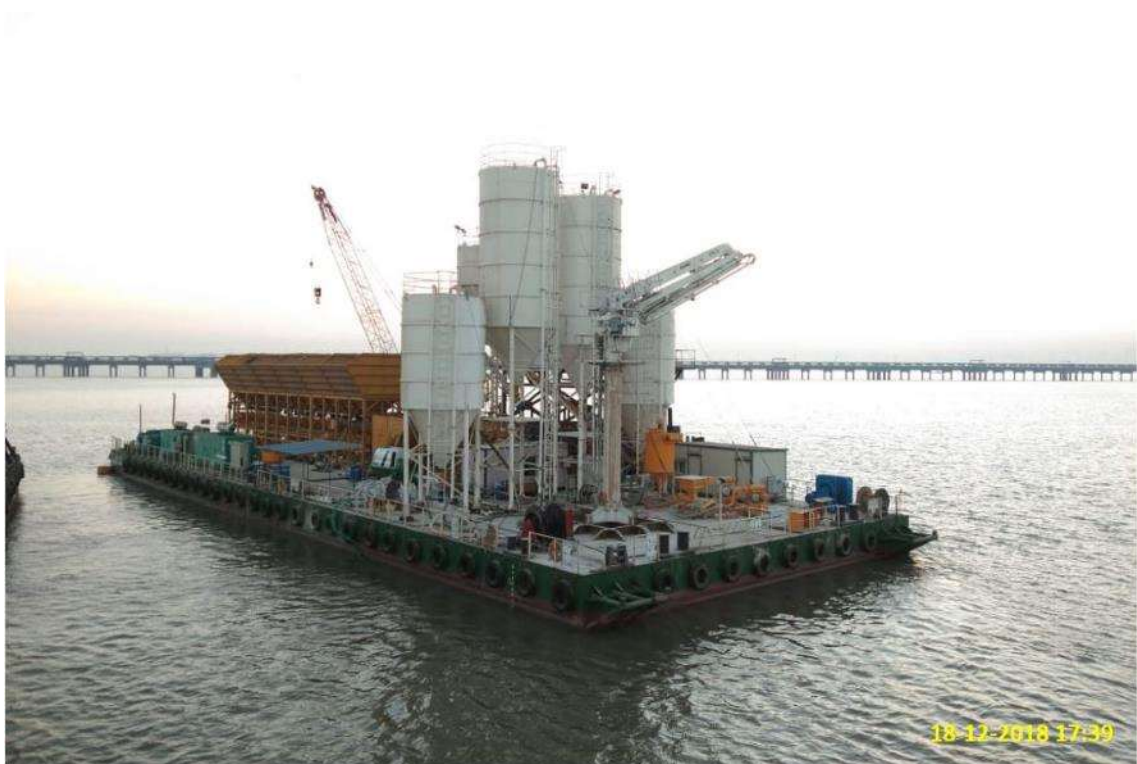
Photo No. 4: Floating Batching Plant is anchored at MP95 Location
