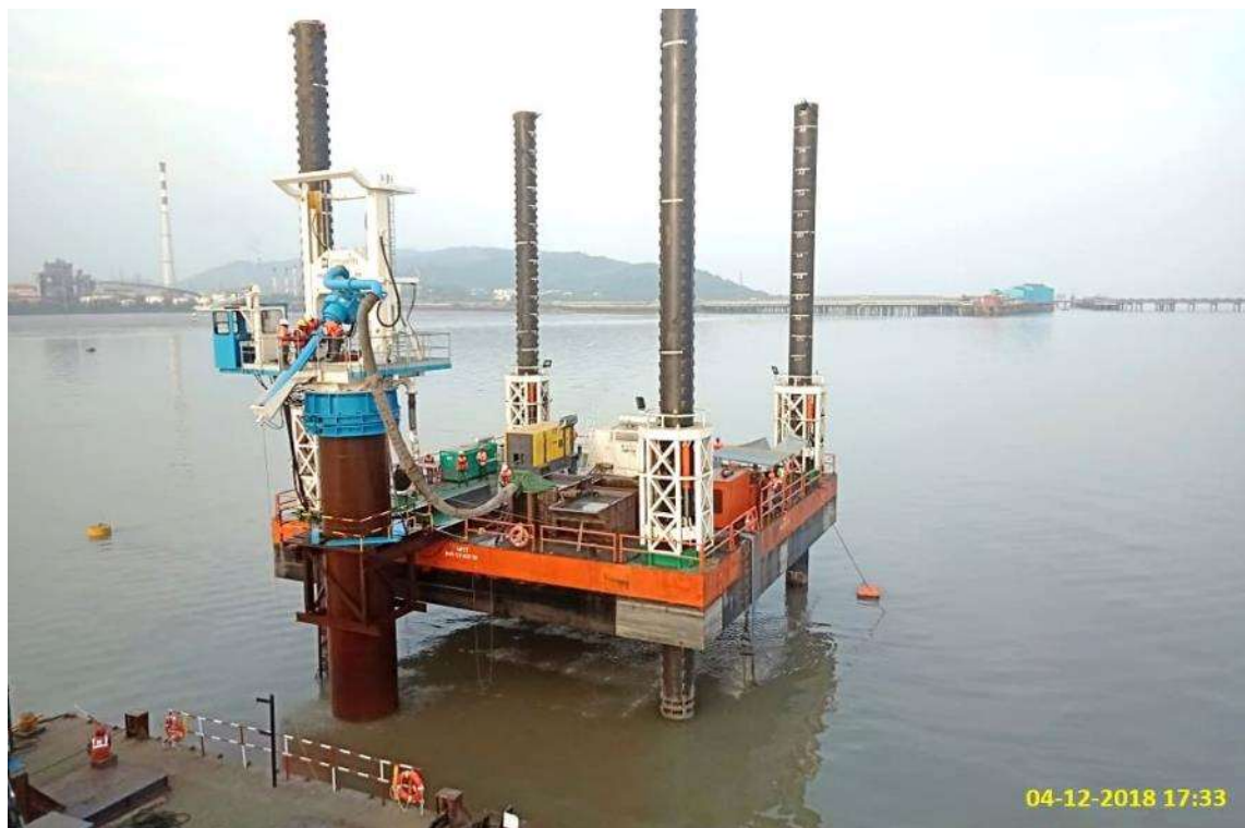
Photo No. 2: Marine Test Pile boring at MP72 Location in progress
