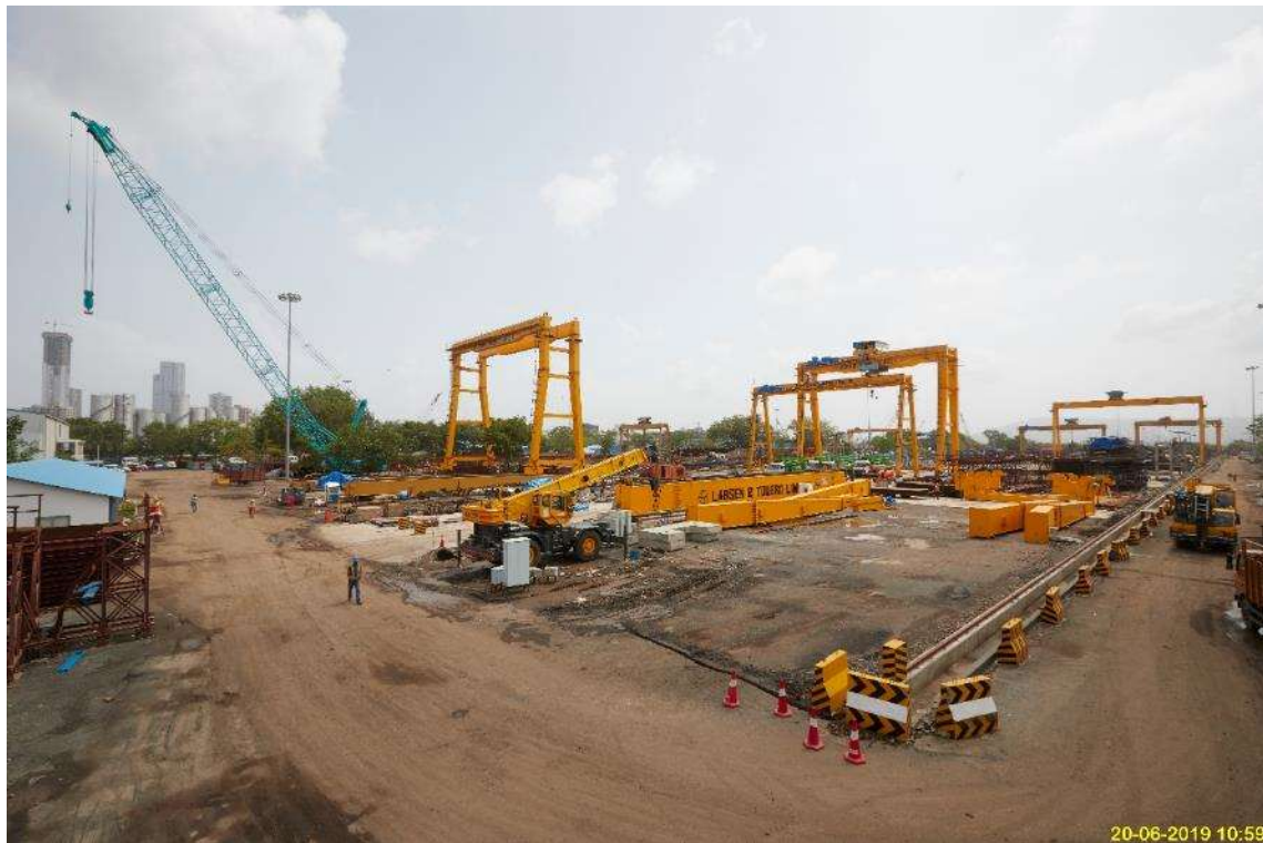
Photo No. 1: Casting Yard Development in progress
