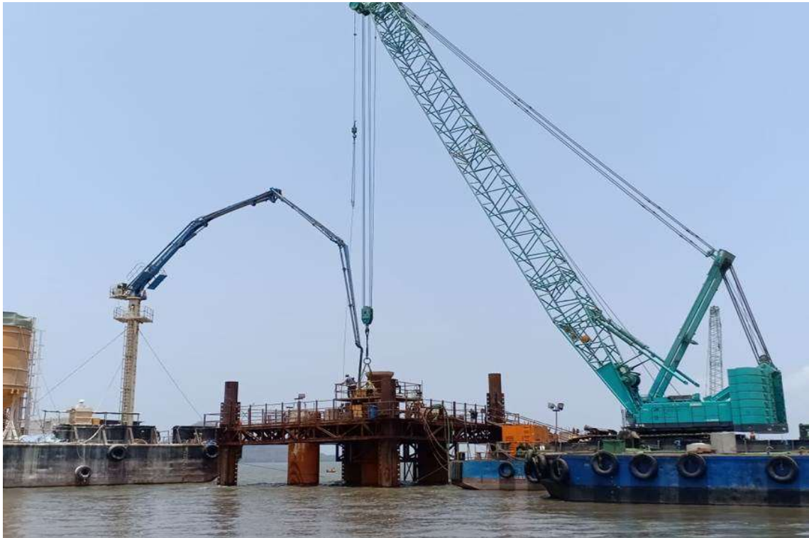
Photo No. 1: Pile Concreting at MP 164/01 LHS in progress
