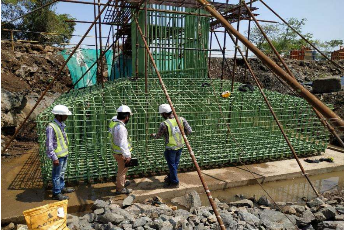
Photo No. 3: Reinforcement inspection for Foundation at RMP 282 in progress
