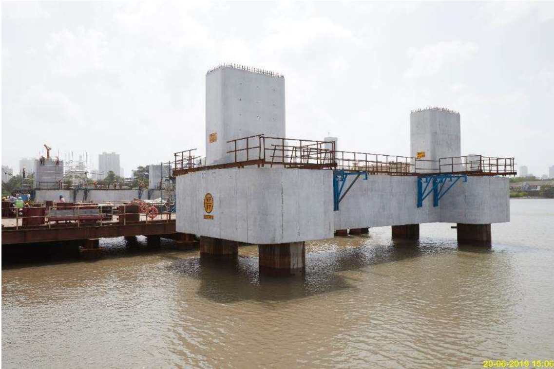
Photo No. 7: Pile Cap & Pier Works at MP7 in progress
