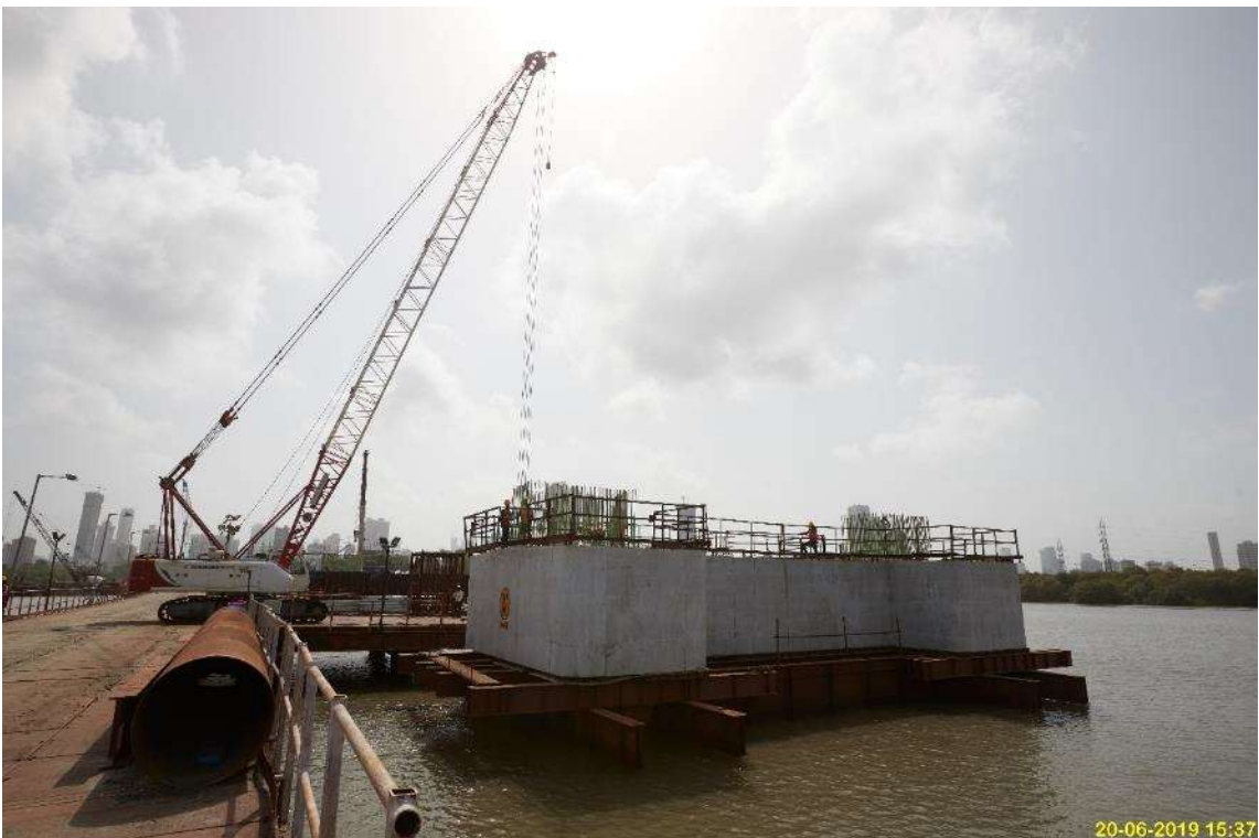
Photo No. 10: Pile Cap Works at MP10 in Progress
