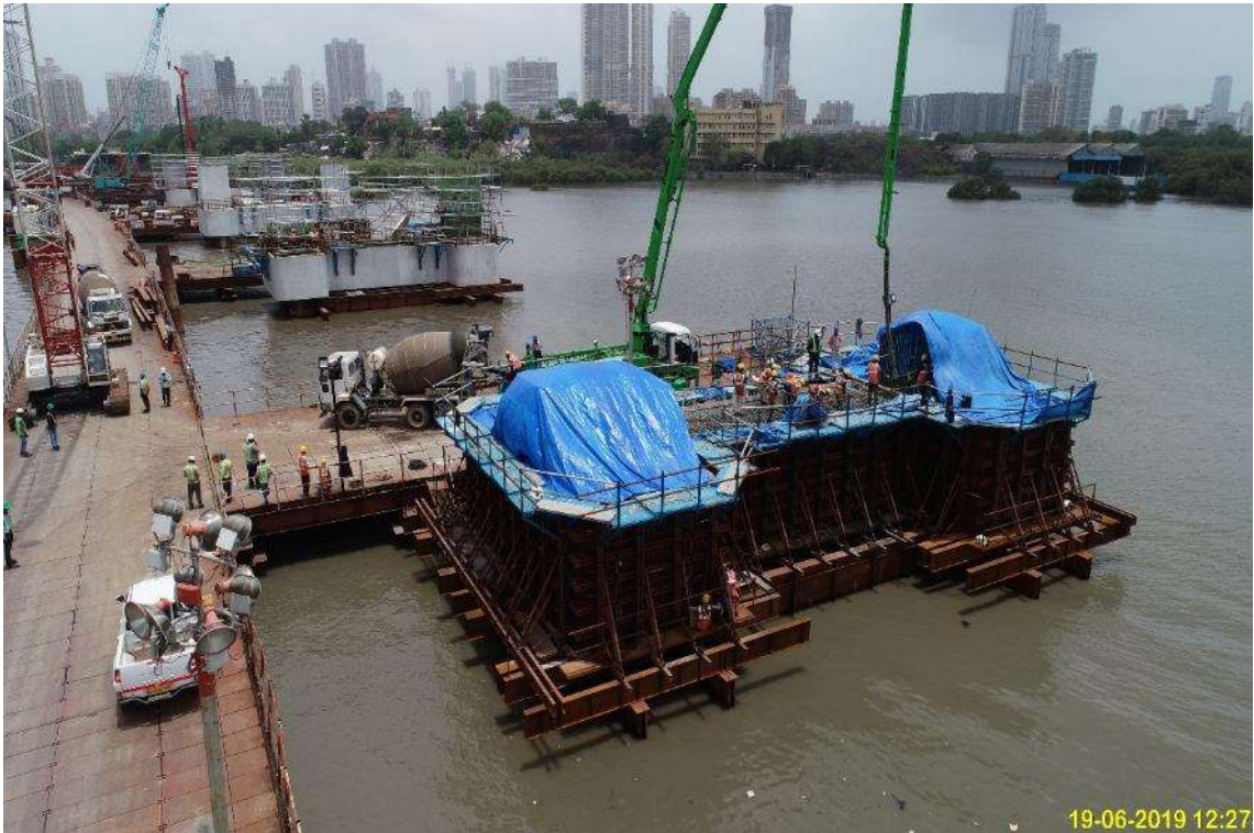
Photo No. 9: Pile Cap Concreting at MP9 in progress
