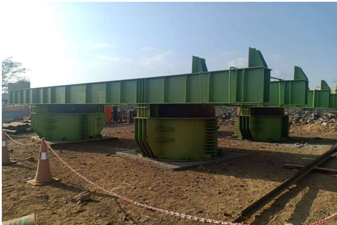
Photo No. 2: Pile Cap Bottom formwork mock-up at Belapur jetty location
