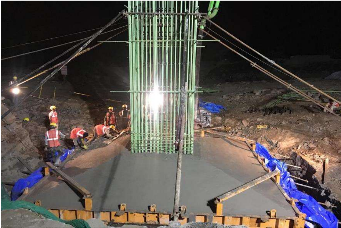
Photo No. 1: Casting of Foundation at location LP 16
