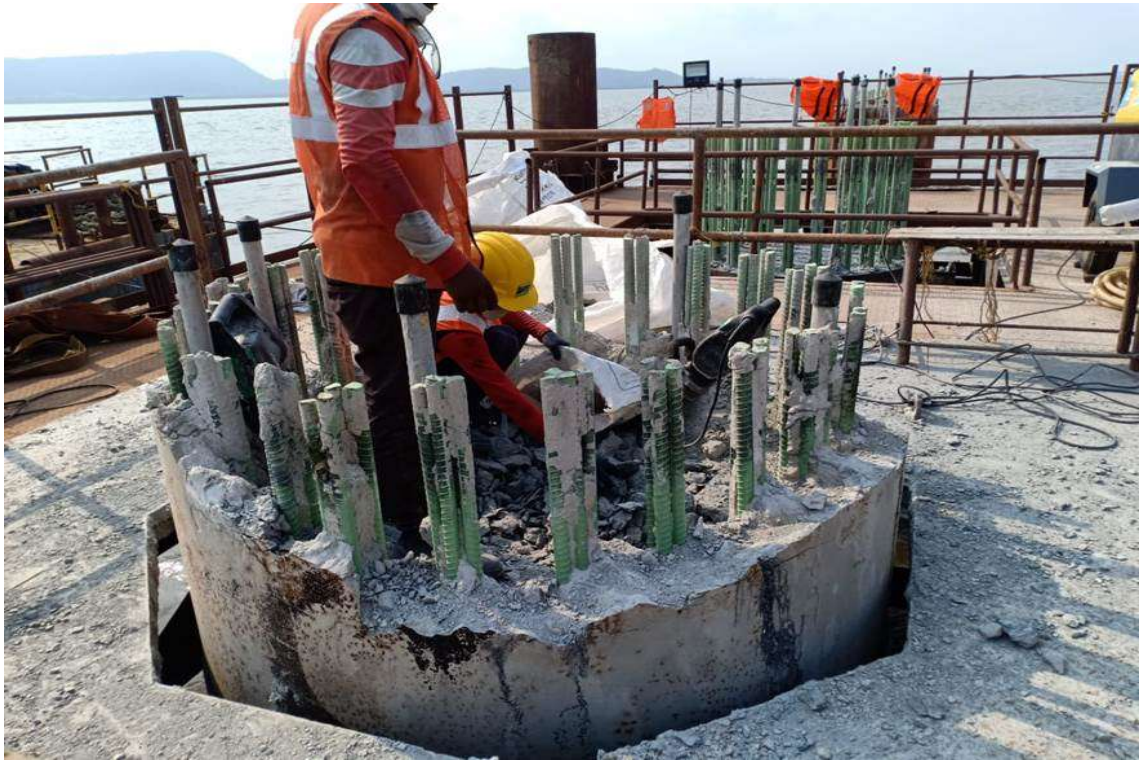
Photo No. 3: Pile head breaking at MP 162 LHS location in progress
