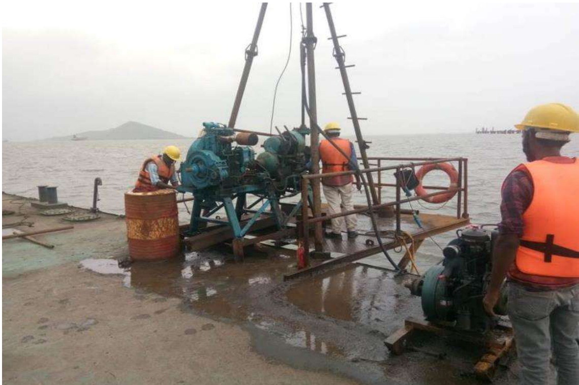
Photo No. 6: Geotechnical Investigation works at location 172A LHS in progress
