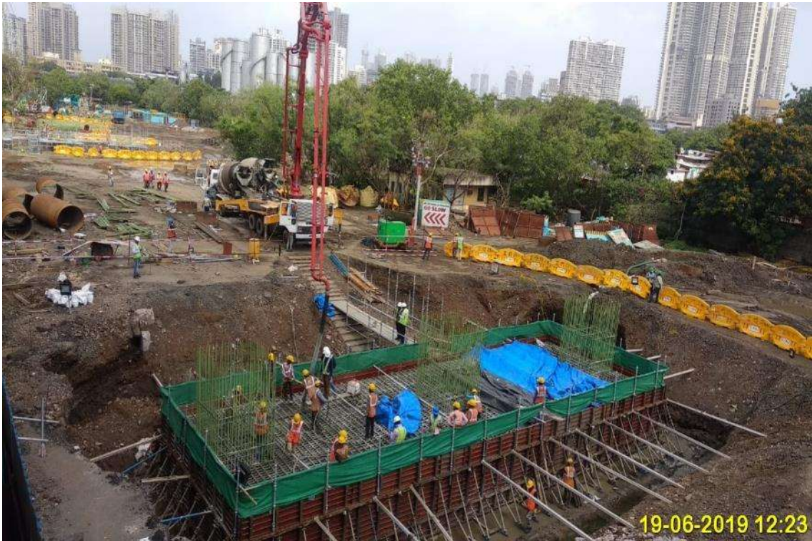
Photo No. 3: C2P8-C1P34-BP45 Pile Cap Concreting in progress
