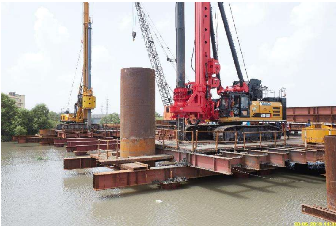
Photo No. 5: Piling Works at MP4 in progress
