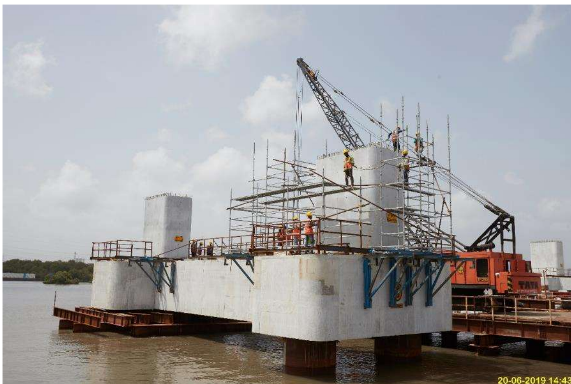
Photo No. 6: Pile Cap & Pier Works at MP6 in progress
