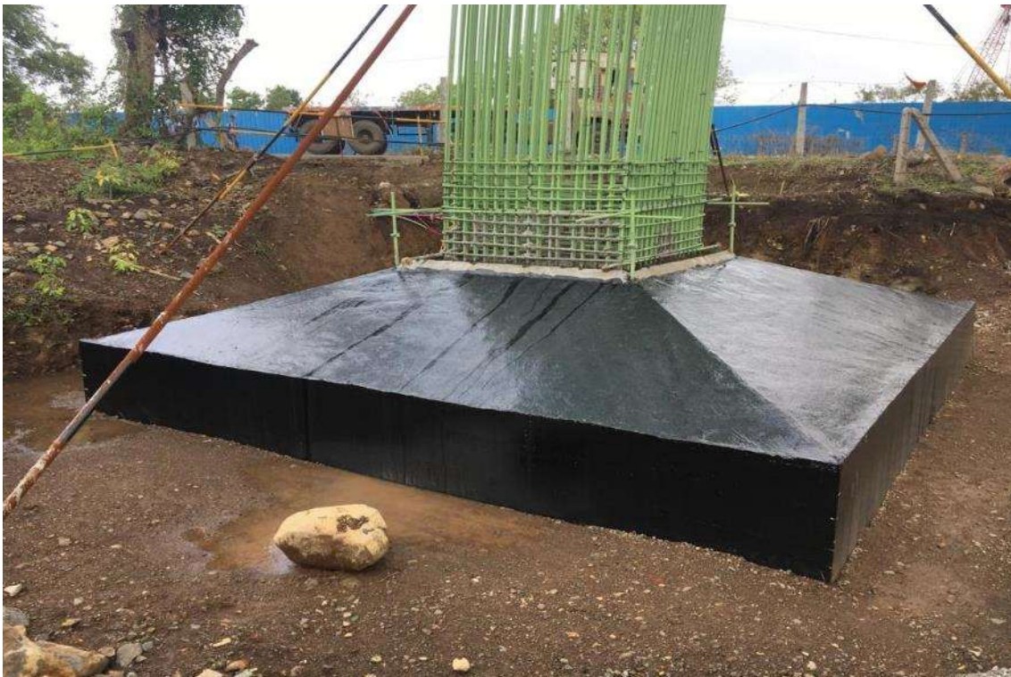
Photo No. 4: Coal Tar Epoxy coating and Foundation Backfilling at RMP 267
