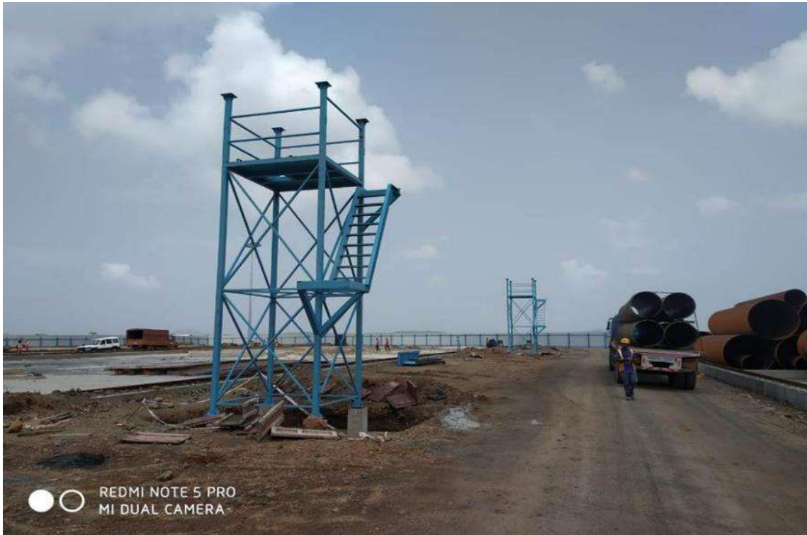
Photo No. 9: Survey Tower erection at Bay-2 in progress
