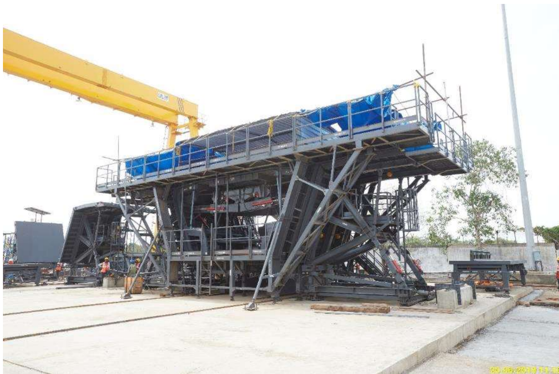
Photo No. 2: 1st Segment Mould Assembly in progress
