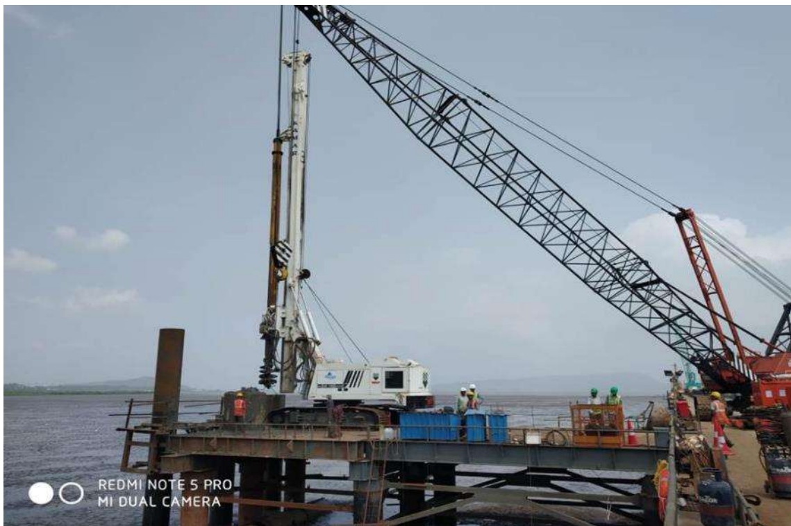
Photo No. 4: Pile Boring at Finger location MP 231 in progress
