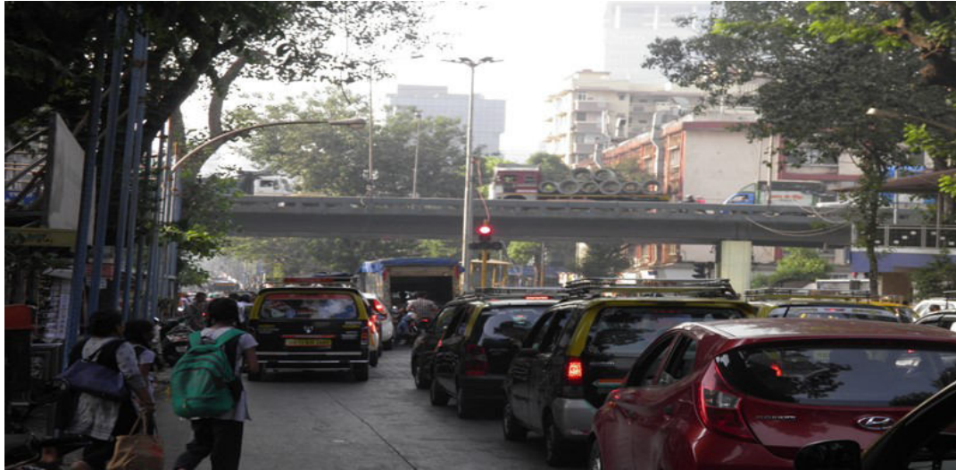
Hindmata Flyover (Parel Flyover)
