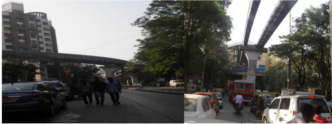
Monorail Enters in Alignment at GD Ambedkar Marg
