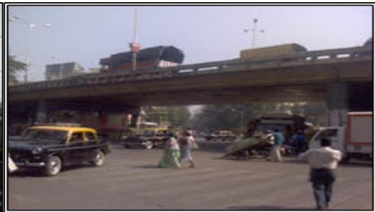
Elphinstone Station Flyover
