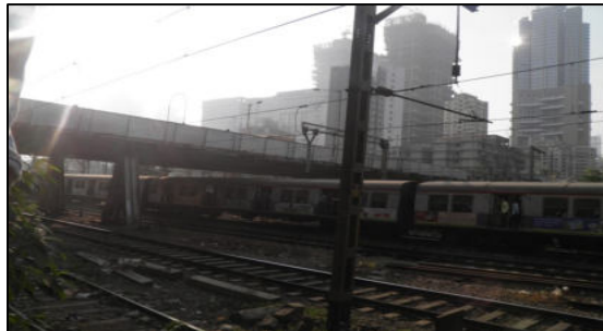
Elphinstone Station Flyover
