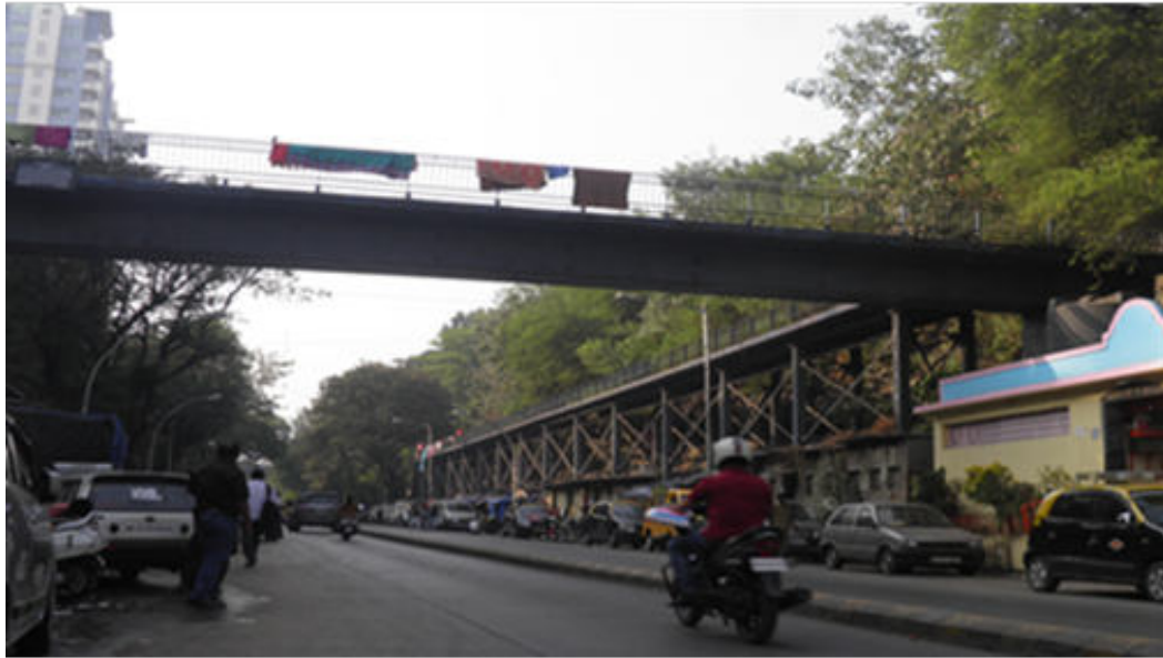
Foot Over Bridge
