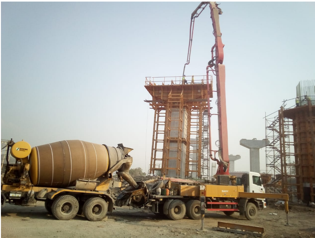
Photo No. 6: LP 14 pier cap concrete pouring in progress
