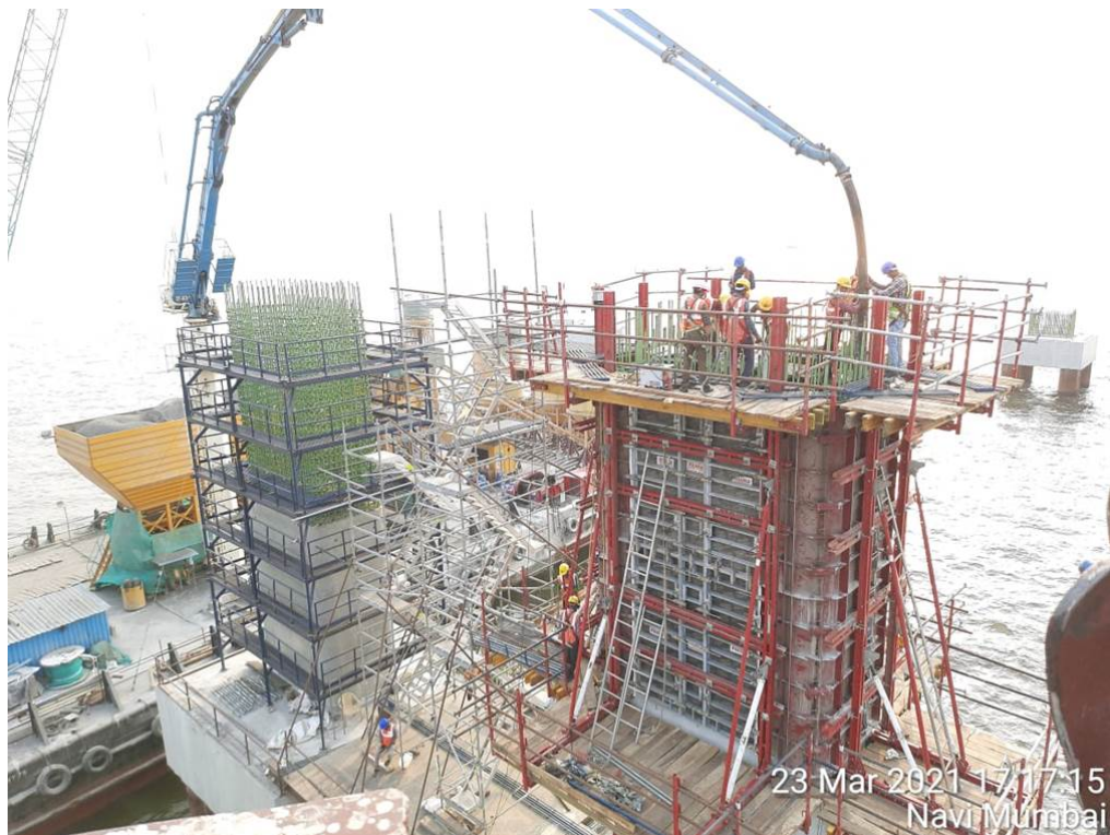
Photo No. 3: Pier 2nd lift concreting at MP 181 LHS in progress
