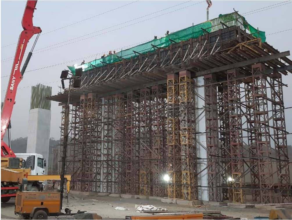
Photo No. 7: RP 33 Portal Concrete pouring work in progress
