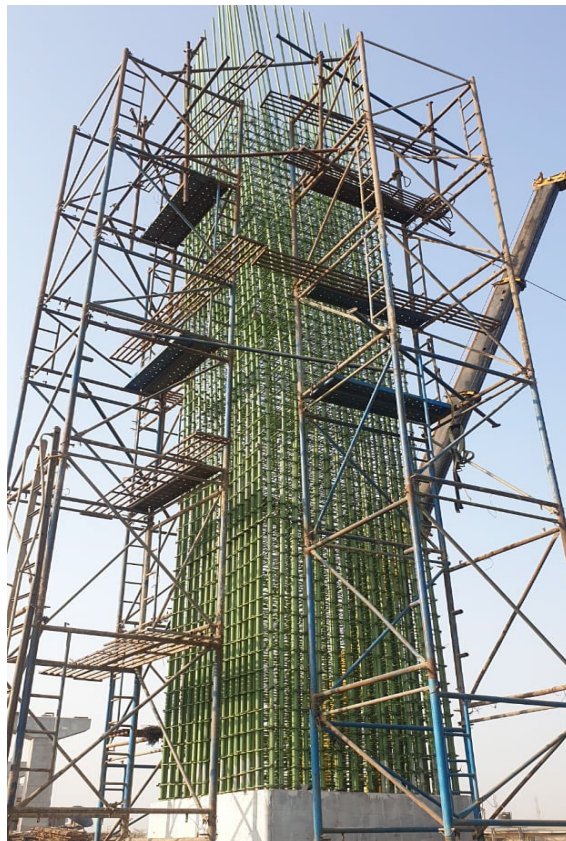
Photo No. 2: LP 18 pier reinforcement works in progress
