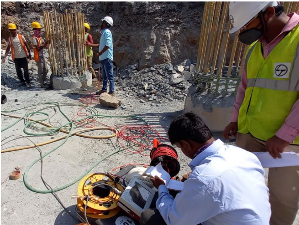
Photo No. 12: Cross hole sonic logging test at LP35 Chirle location
