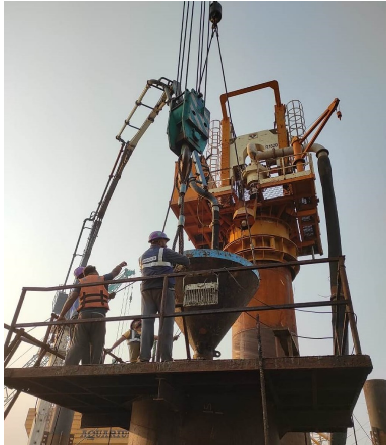
Photo No. 11: Pile concreting at MP 167 LHS in progress
