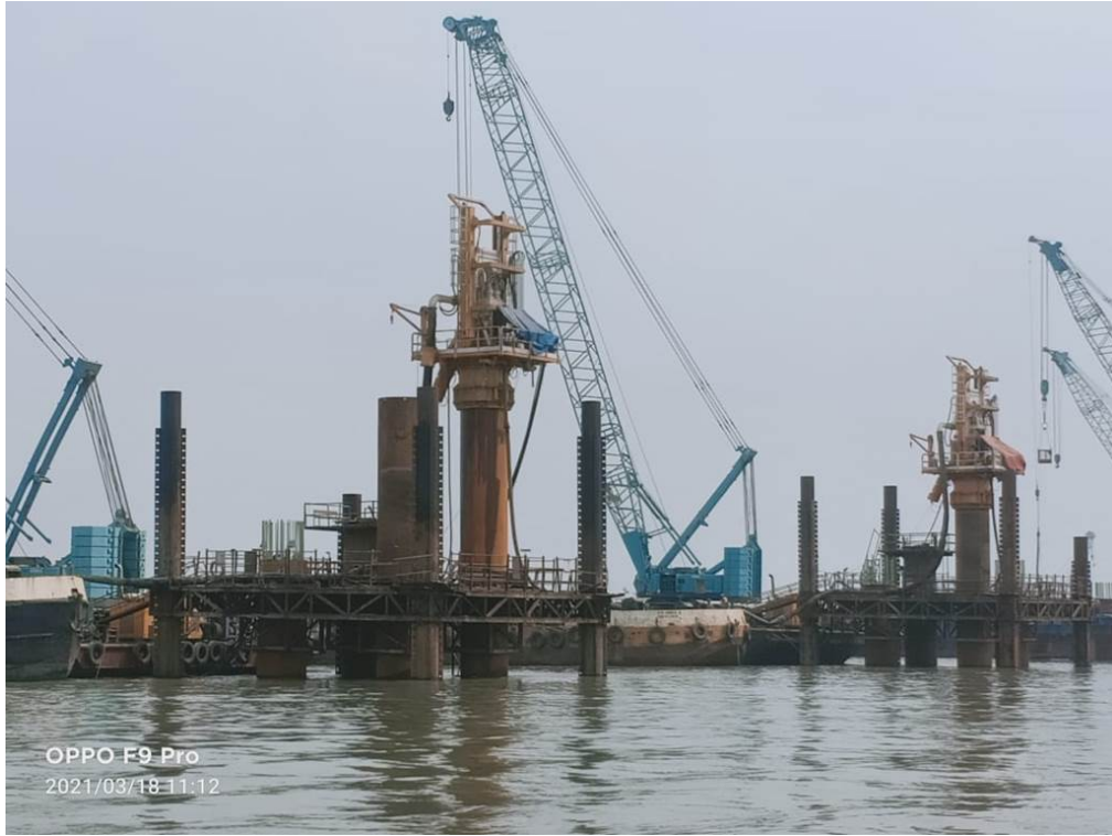
Photo No. 5: Pile drilling at MP 151 LHS in progress
