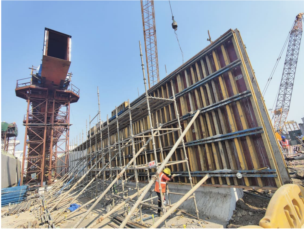
Photo No. 5: C2 Ramp Retaining wall in progress
