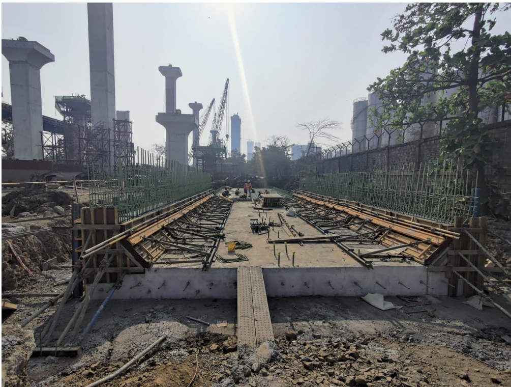
Photo No. 8: F2 Zone 2 Retaining Wall works in progress
