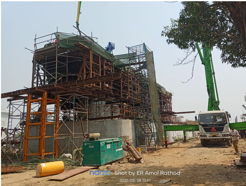
Photo No. 10: Casting of Pier cap MP01 North in progress
