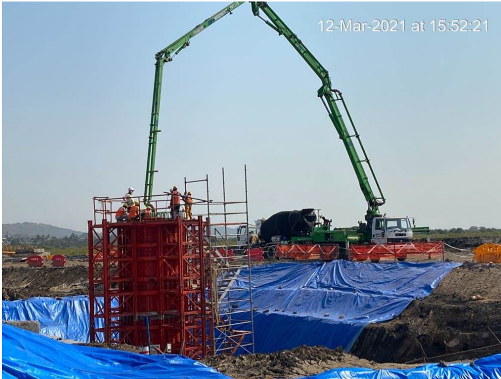
Photo No. 9: Pier concreting at CAP-10 in progress
