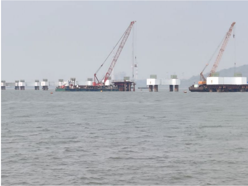
Photo No. 11: Pier Cap Works at the Marine Section in progress
