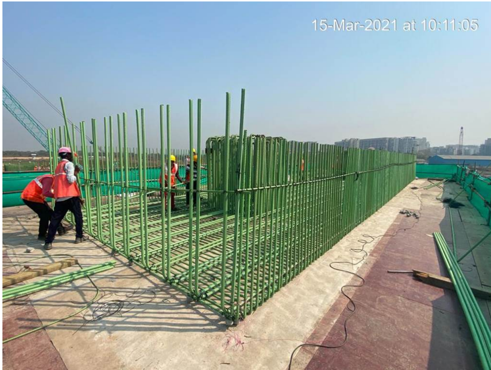
Photo No. 7: Portal Beam reinforcement works at MP 252 LHS in progress
