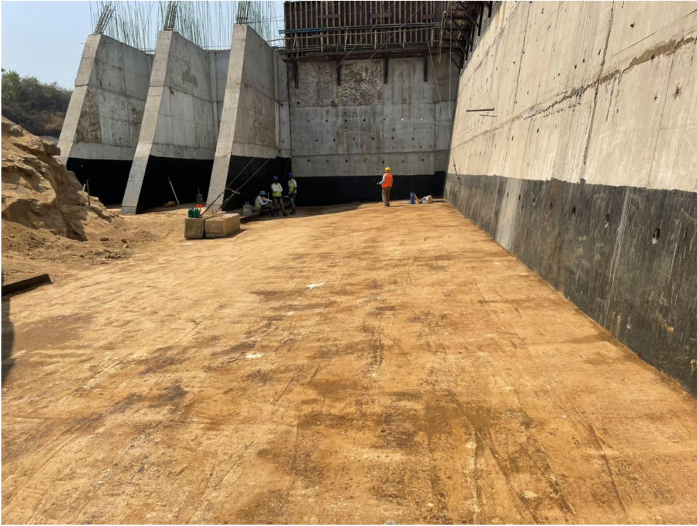
Photo No. 1: LMP & RMP A2 Abutment backfilling work in progress
