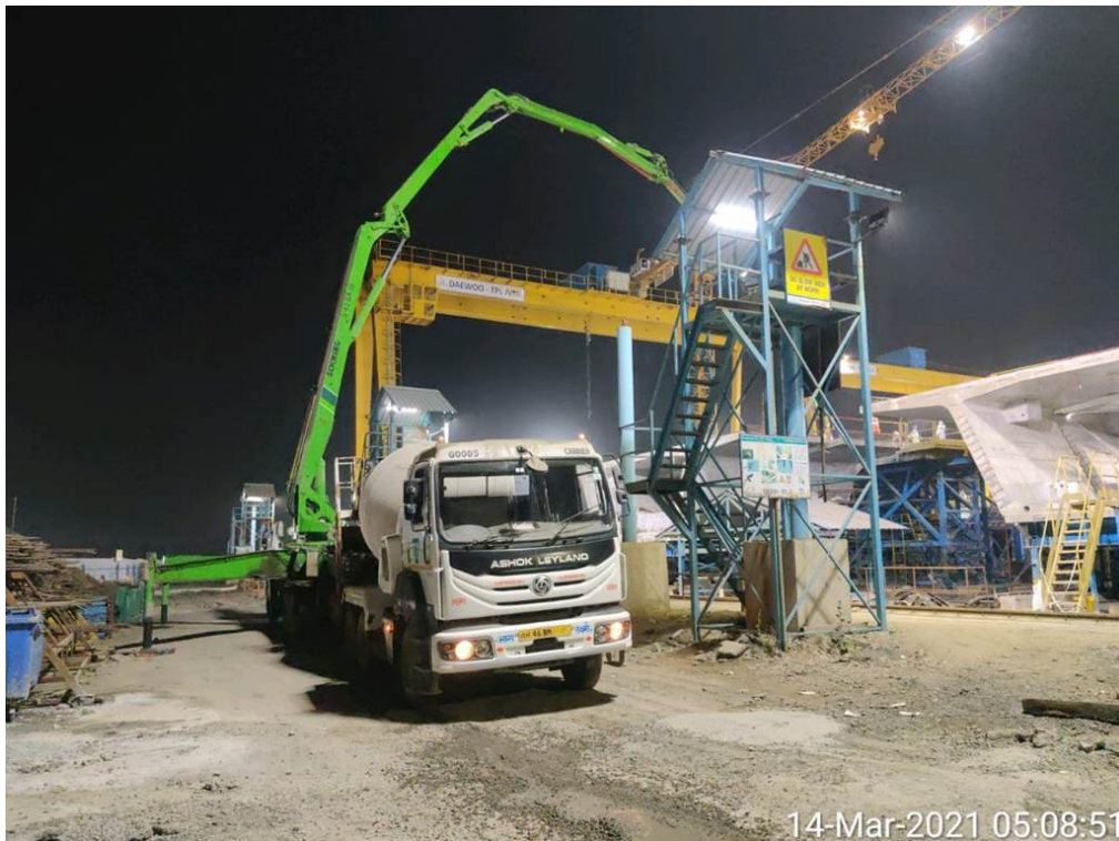
Photo No. 8: Segment concreting at Bay-2 in progress
