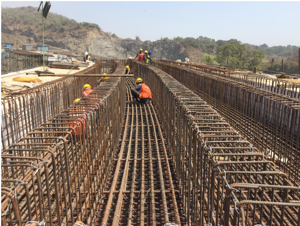
Photo No. 8: PMP11 to PMP12 Voided slab soffit reinforcement in progress
