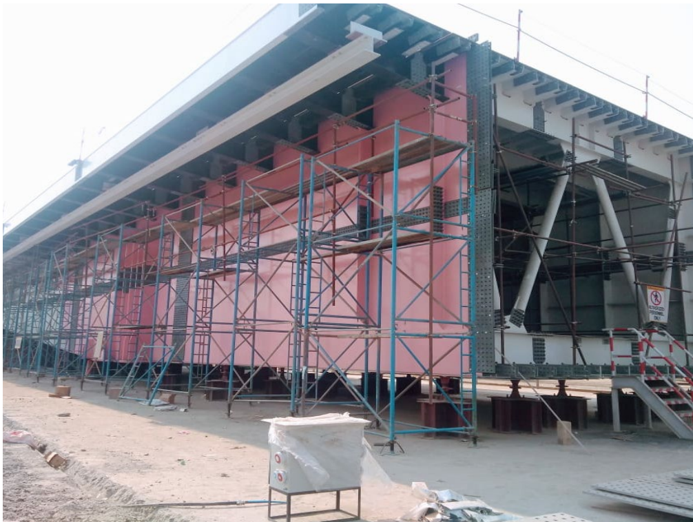
Photo No. 6: OSD-2 Super Structure Assembling Works in progress
