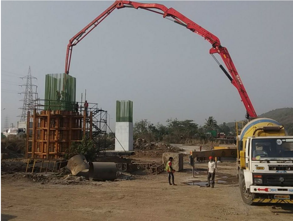
Photo No. 5: RP 36 Pier concrete pouring in progress
