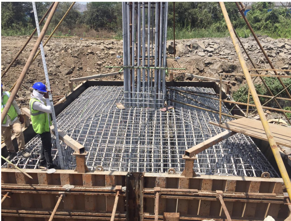
Photo No. 4: JMP 4 foundation final checking before concreting
