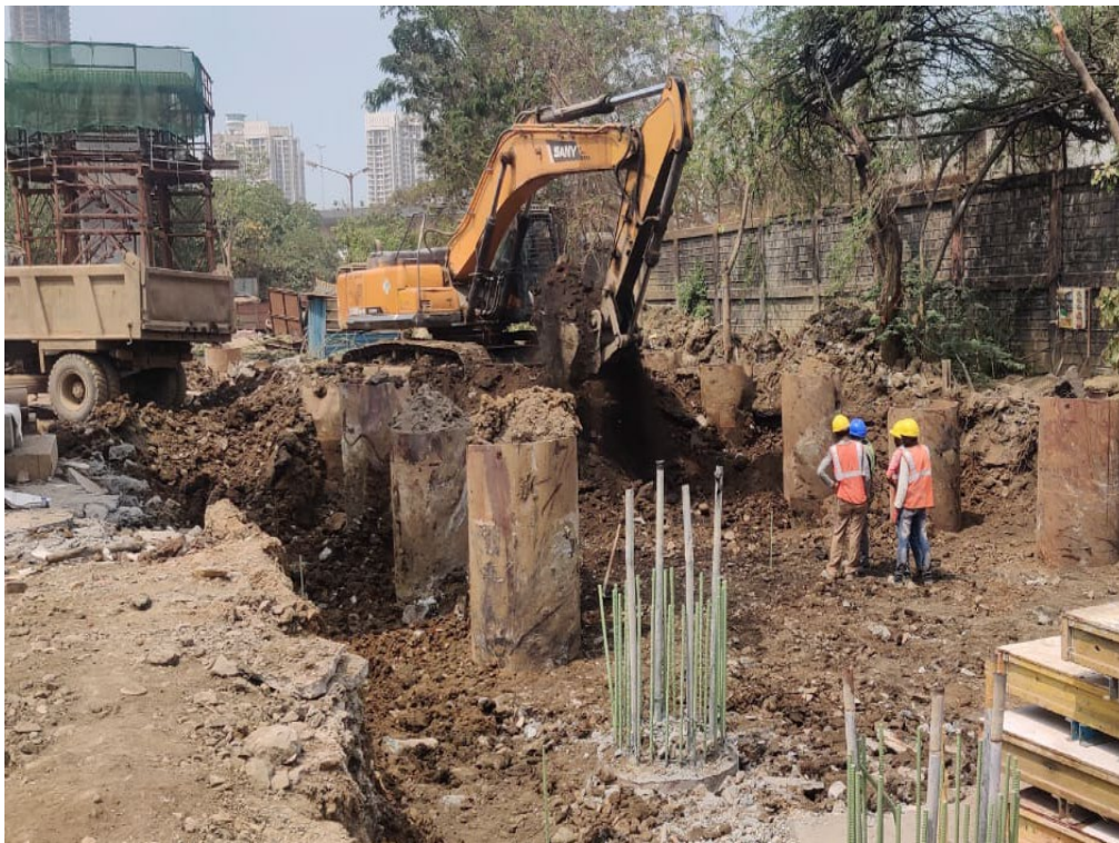
Photo No. 12: F Ramp Retaining Wall Zone-3 Excavation Works in progress
