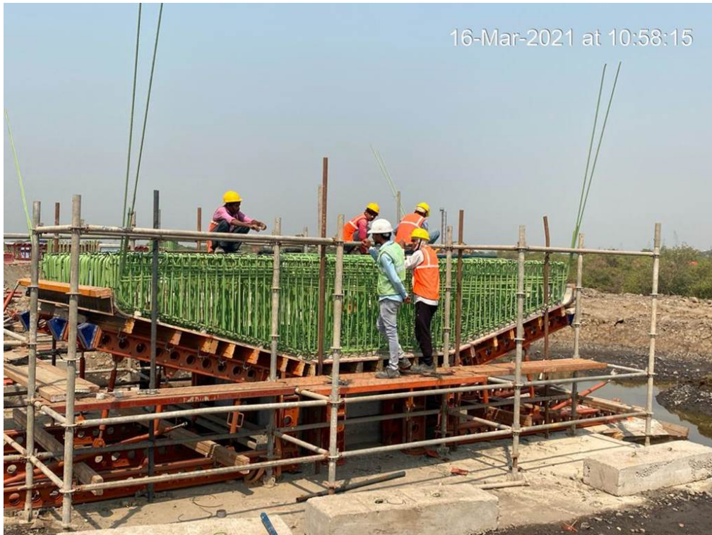
Photo No. 6: Pier cap reinforcement works at CAA-1 in progress
