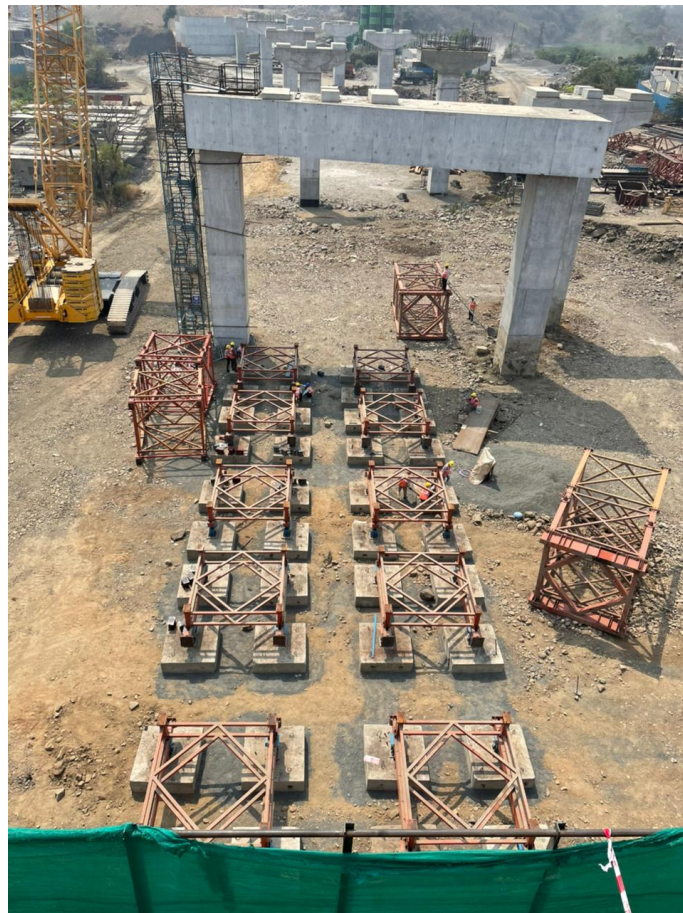
Photo No. 10: Span LMP 278-279 under slung trestle installation in progress
