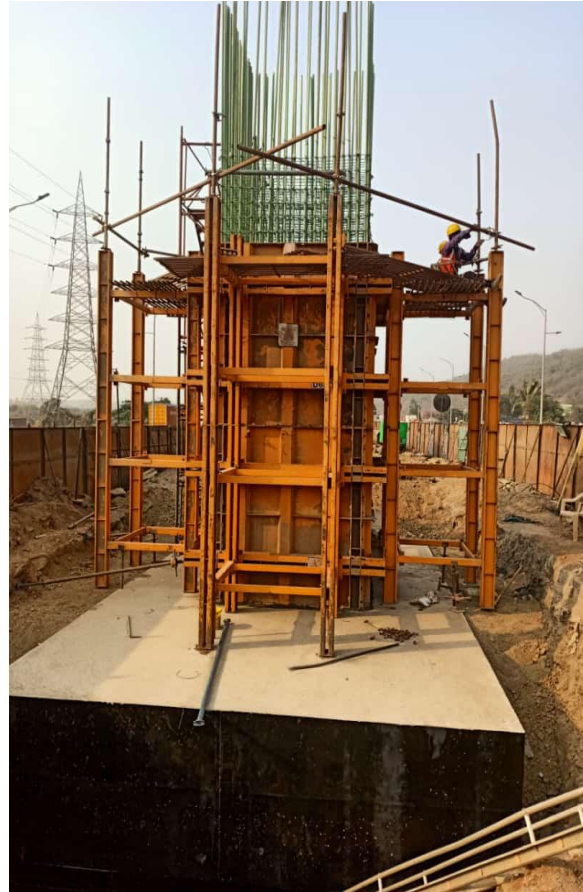
Photo No. 3: LP35 pier shuttering works in progress
