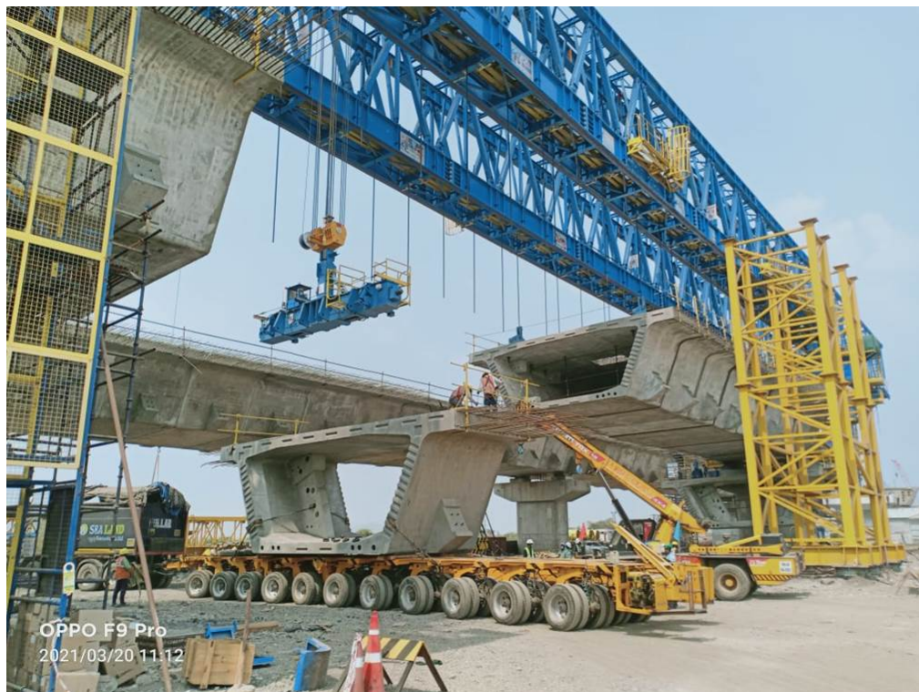
Photo No. 4: LG-2 Segment erection at Span MP 243-244 LHS in progress
