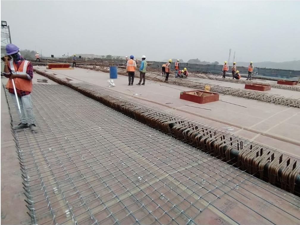
Photo No. 9: RP4-3 Cast in-situ 3 cell box girder Deck slab reinforcement in progress
