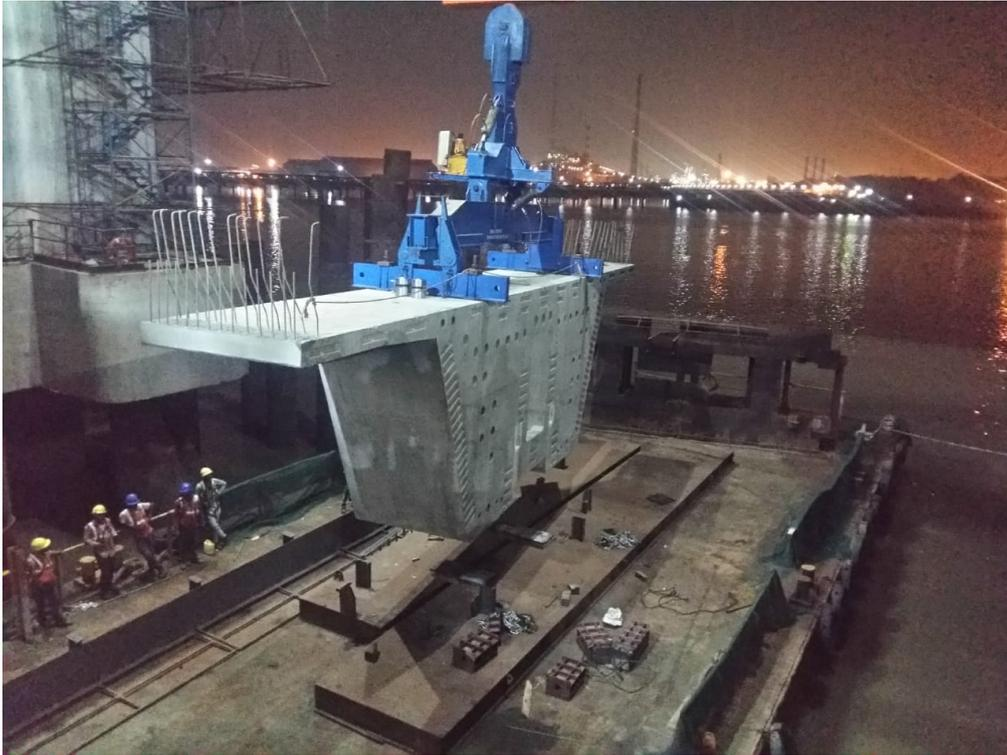
Photo No. 9: Erection of Pier segment for LG-03 at MP81 in progress
