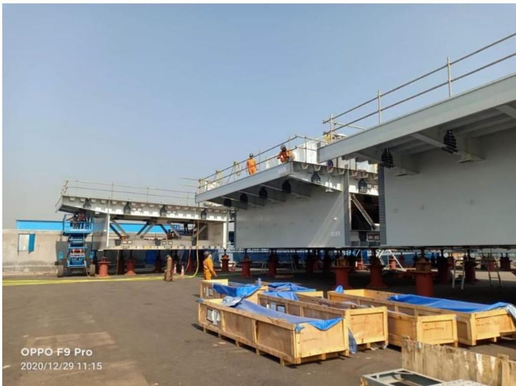
Photo No. 4: OSD small block assembling and welding at Karanja Port in progress
