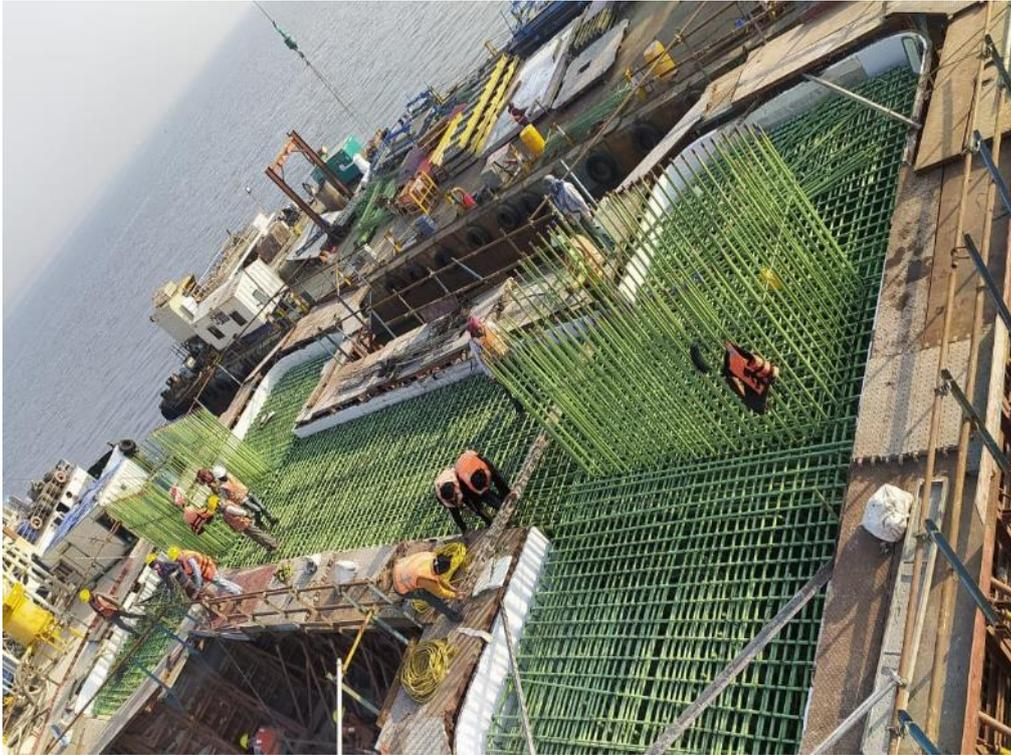
Photo No. 9: MP 123 Pile Cap Pre-Pour Checking at Marine Section in progress
