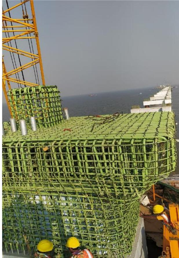
Photo No. 5: MP100 S Pier Head Rebar Inspections at Marine Section in progress
