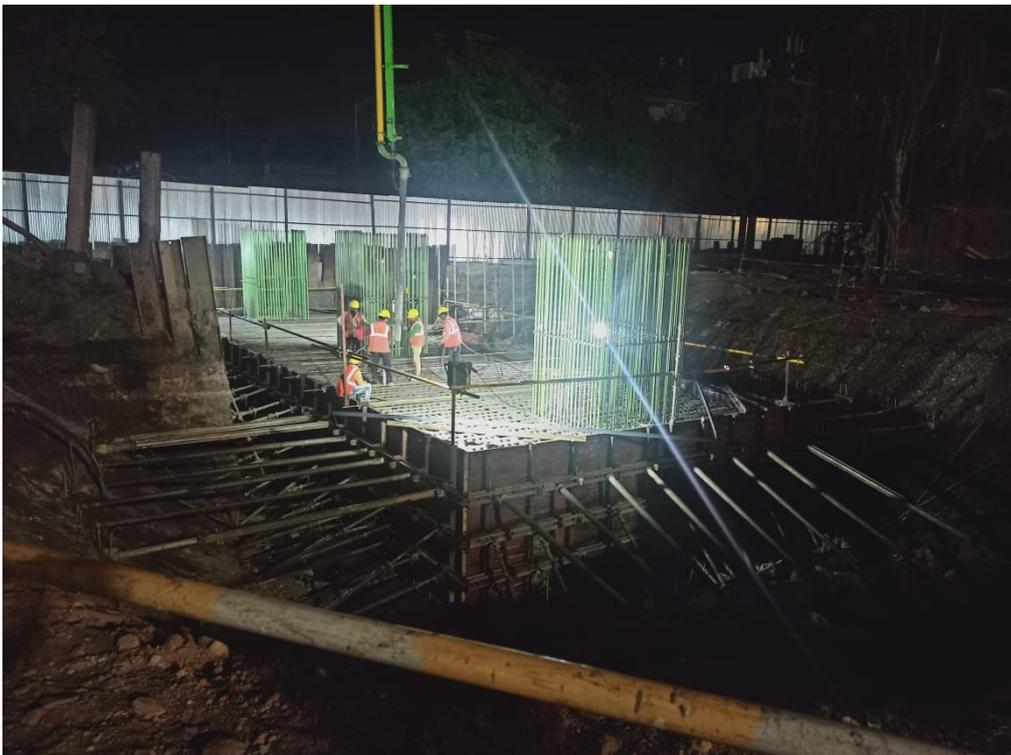
Photo No. 4: Casting of combined Pile cap at Interchange Section in progress
