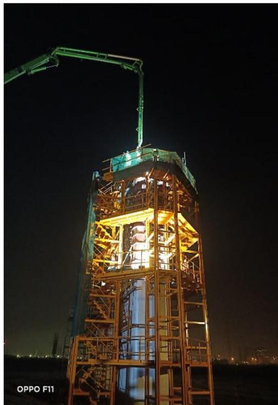
Photo No. 2: MP44S L2 (Final Lift) Pier Concrete Works – Intertidal Location in progress
