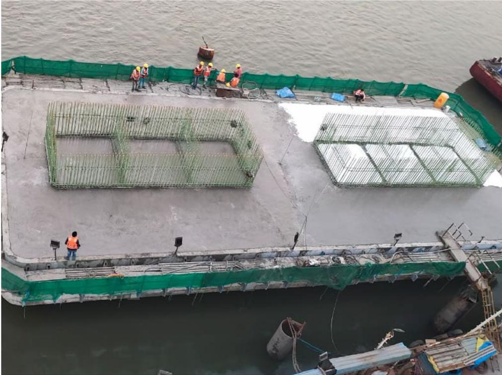
Photo No. 3: Casting of OSD Pile Cap at MP125 – Marine Section in progress
