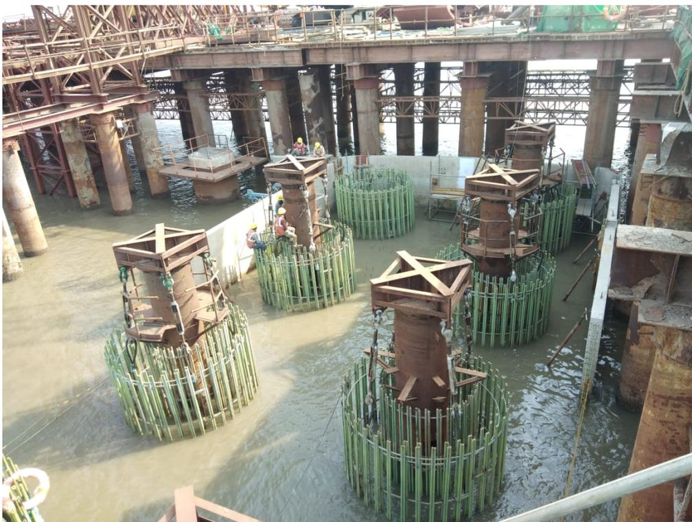
Photo No. 2: MP 52 OSD Pile Cap Works at the Marine Section in progress
