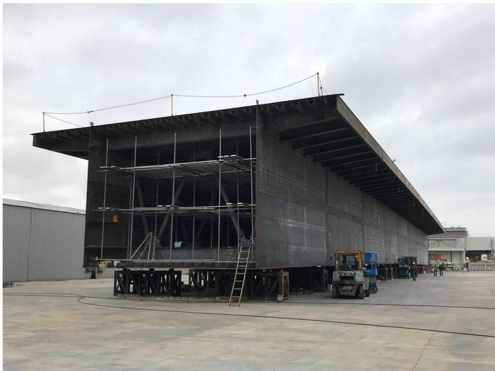
Photo No. 12: Trial Assembly completion for OSD Girder Bridge P1-OS01-SG (Lot5) / Seg. 12~17
