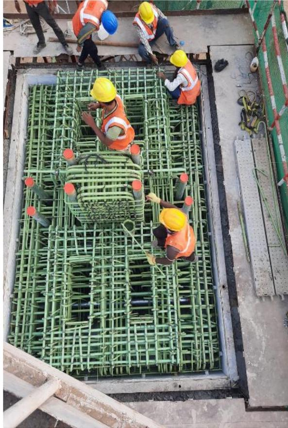
Photo No. 3: LP 6 N Pier Head Pre-Pour Checking - Interchange Location in progress
