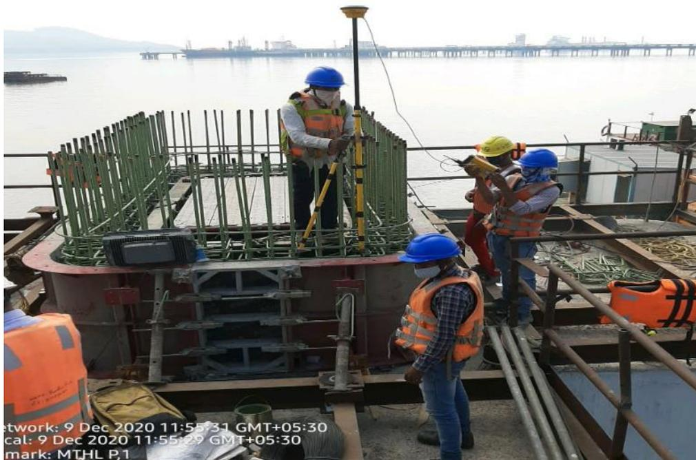
Photo No. 11: MP 97 S Starter Co-Ordinates Checking at Marine Location in progress
