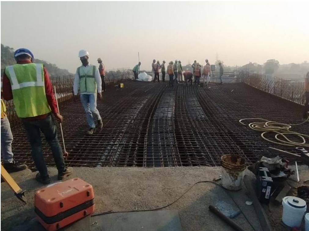
Photo No. 8: voided slab and cantilever portion reinforcement at Span MJP6 - MJP7 in progress
