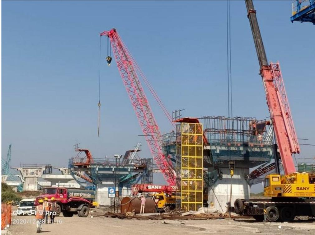
Photo No. 5: Pier head segment reinforcement tying at MP 242 LHS in progress
