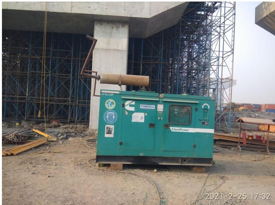
**Photographic evidences of construction equipment used by contractors are provided with exhaust silencers to reduce noise**
