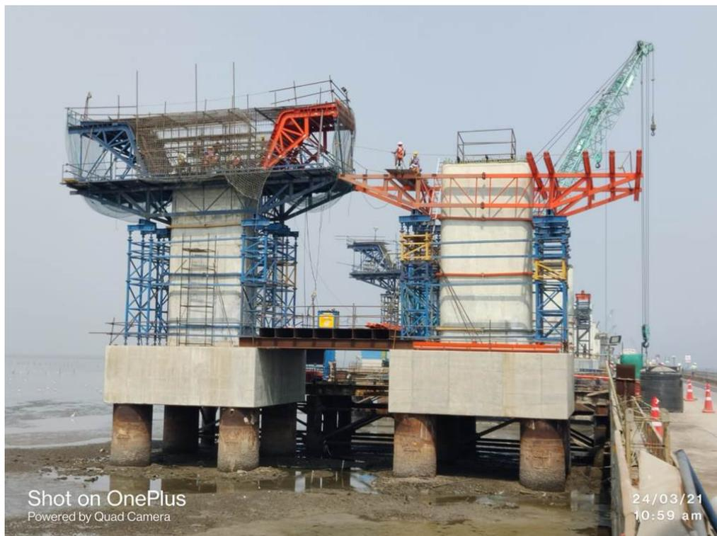
Photo No. 2: Pier head segment scaffolding and reinforcement at MP 229 LHS and RHS respectively in progress
