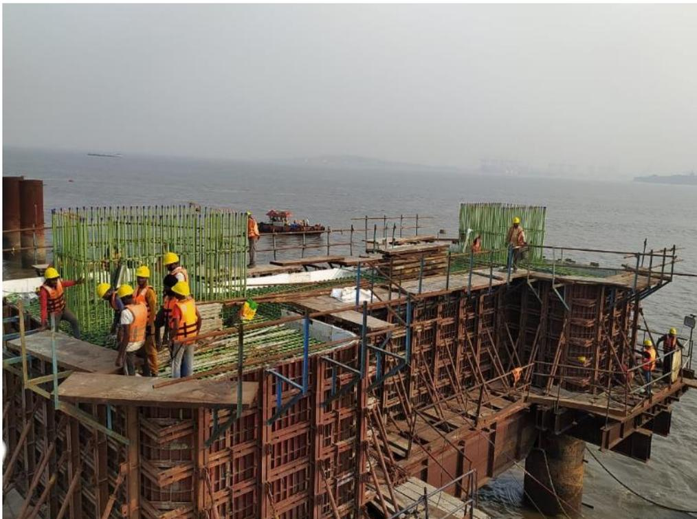
Photo No.8: MP 120 Pile Cap Pre-pour Checking at Marine Section in progress
