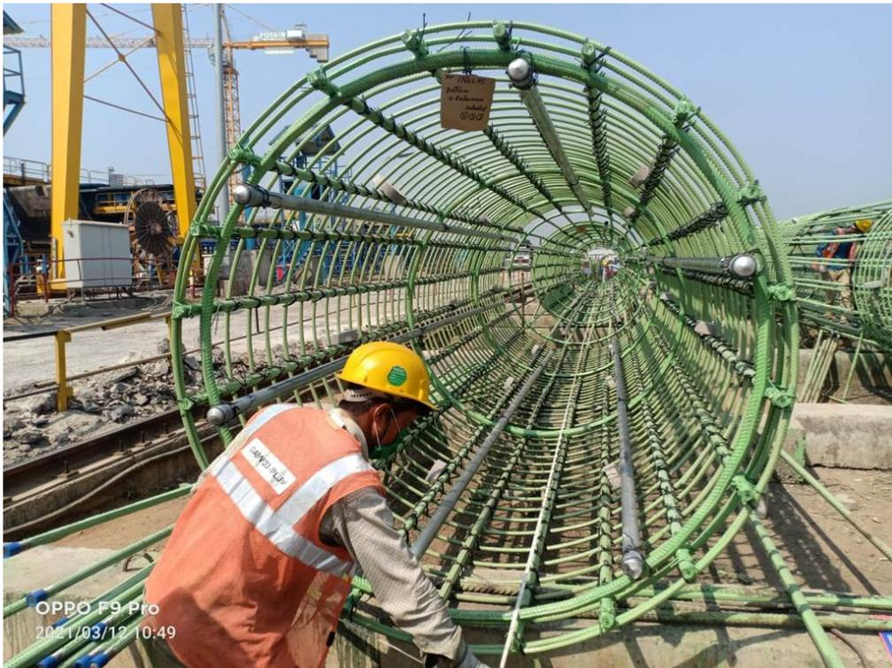
Photo No. 10: Pile reinforcement cage inspection at the Casting Yard in progress
