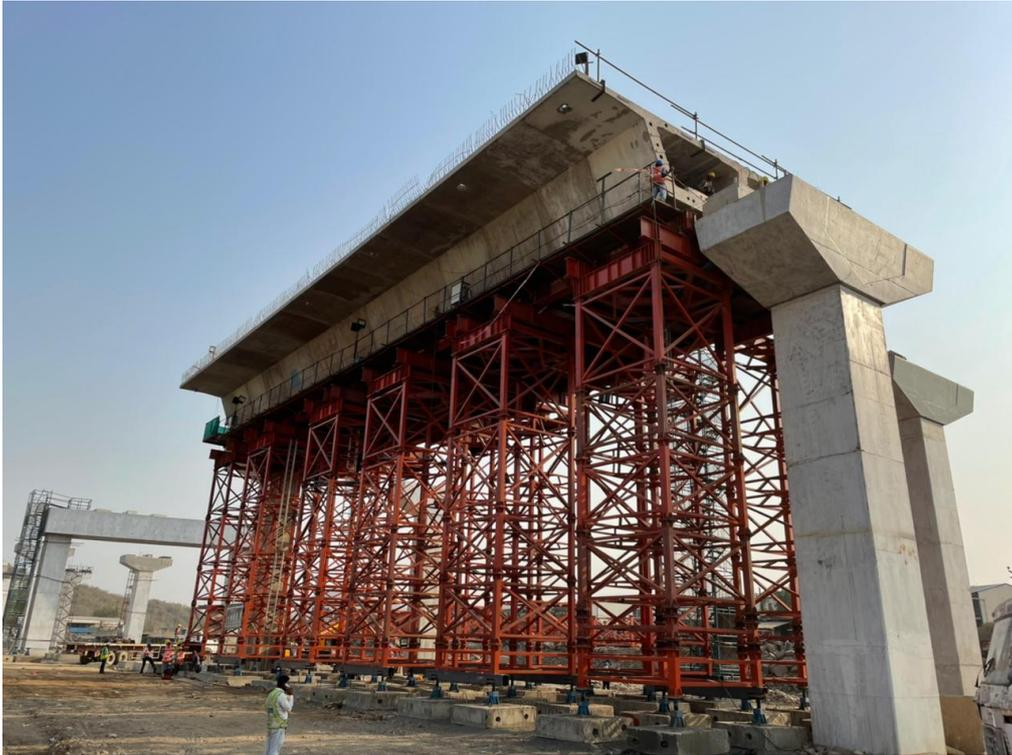
Photo No. 11: Span LMP 277-278, Segment gluing and temporary pre-stressing work in progress
