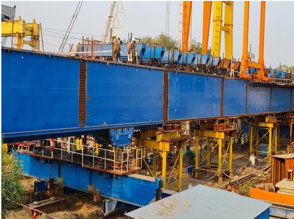
Photo No. 4: LG-3 Load Test at the Precast Yard Location in progress
