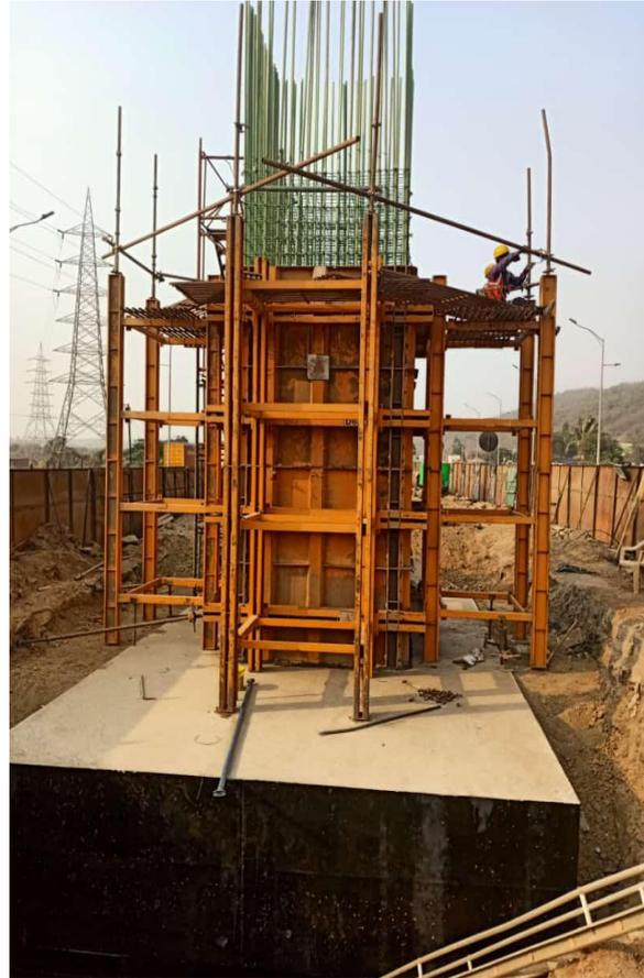
Photo No. 3: LP35 pier shuttering works in progress
