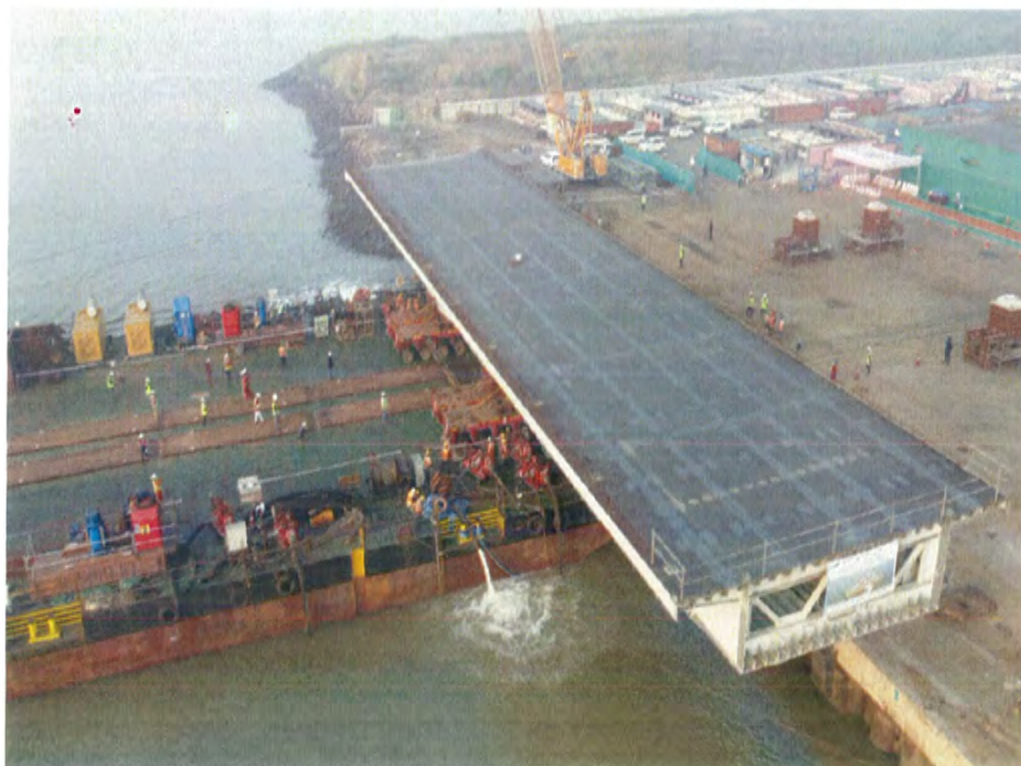
Photo No. 2: Load-out of the 1st OSD Span on the barge
