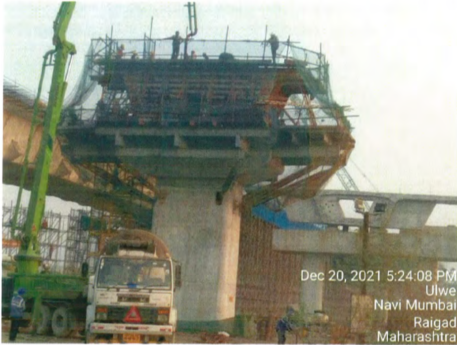
Photo No. 9: Pier Head Segment concreting at MP 258 RHS
