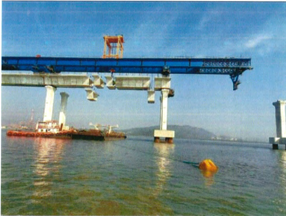
Photo No. 11: View of LG-03 (erection of span MP87-88)
