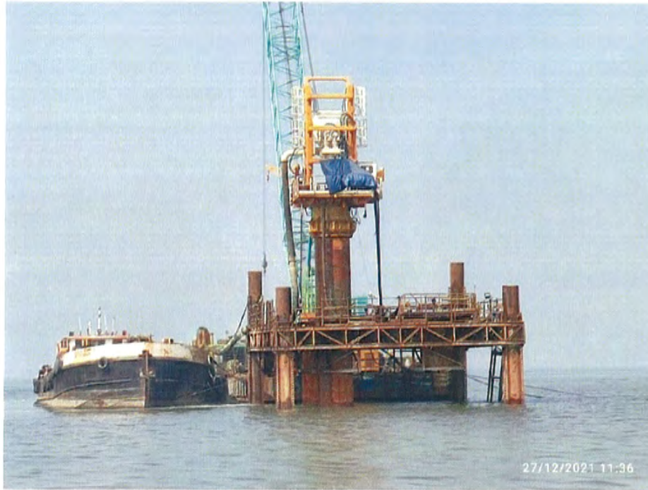
Photo No. 5: Pile boring at MP 173 RHS in progress
