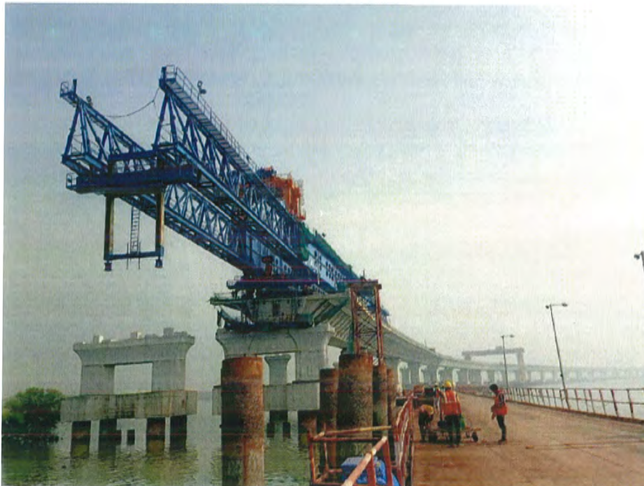
Photo No. 2: Erection of segment at MP04-05 south
