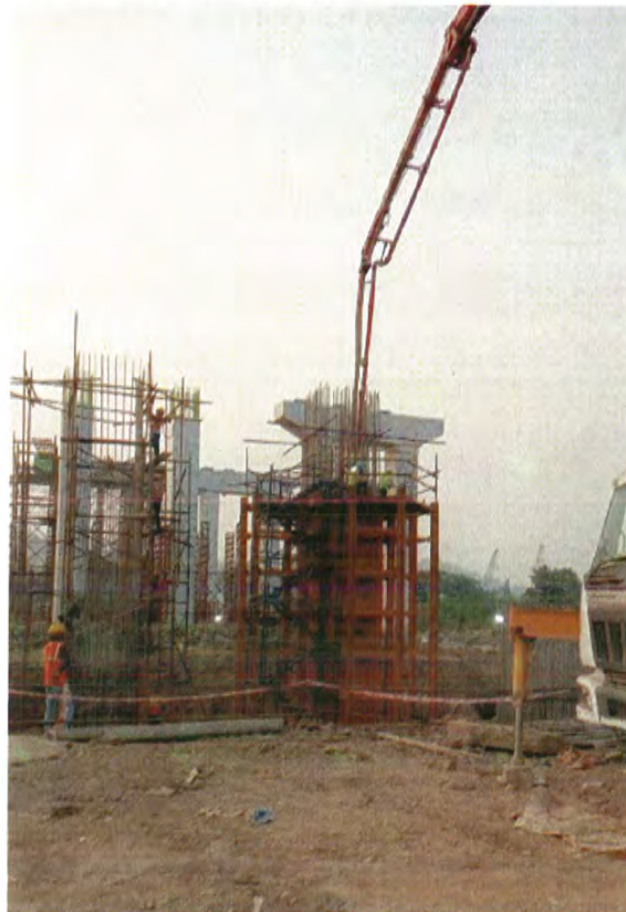
Photo No. 8: RP 24C pier 1st lift 6.5m concrete pouring work in progress
