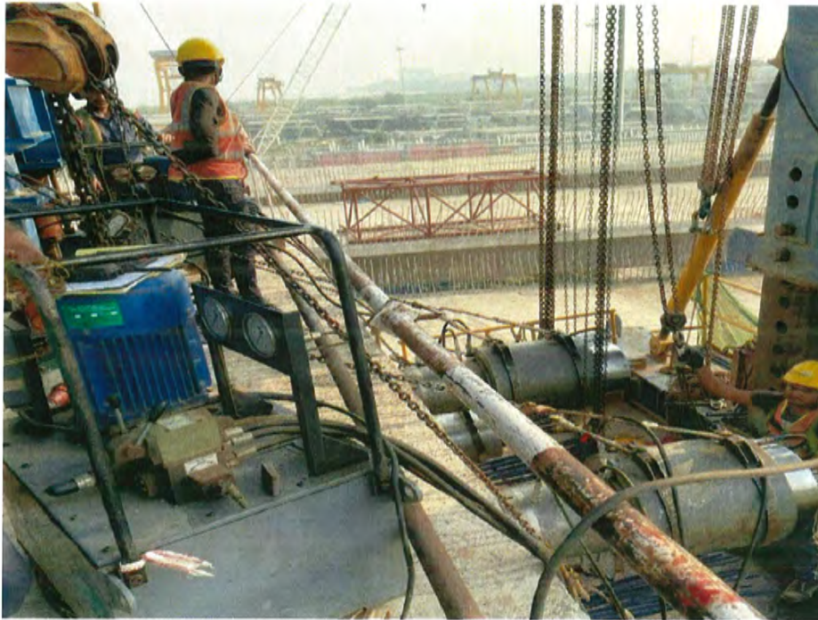
Photo No.7: Stressing activity for Interchange LPS Ramp in progress
