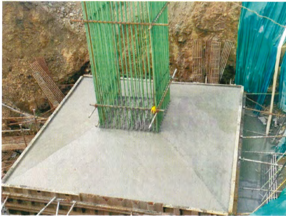
Photo No. 7: LMP 271 Foundation completed
