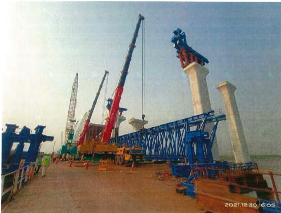
Photo No. 5: Erection of LG-05 at MP53-54 South in progress
