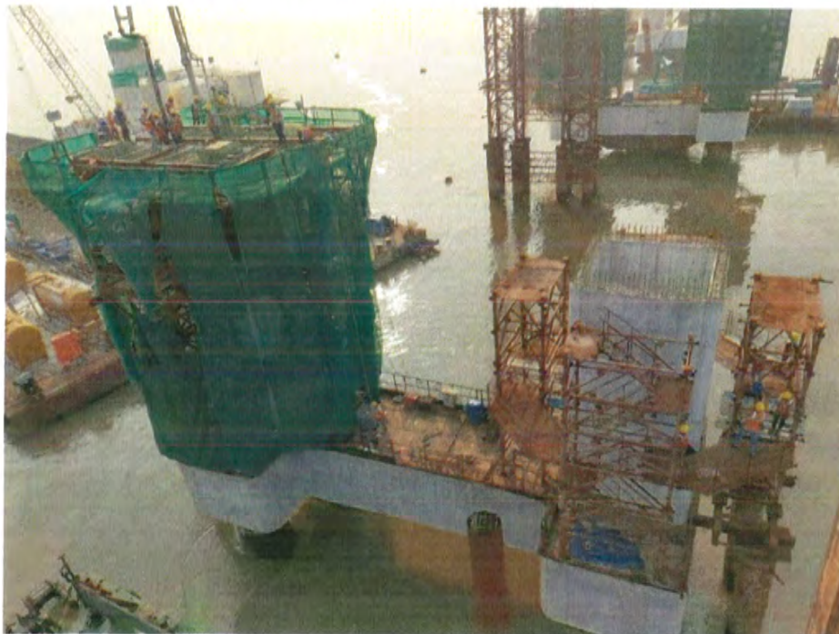
Photo No. 10: Concreting of Pier Cap – MP 148 South in progress
