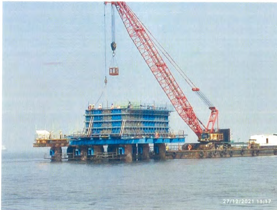
Photo No. 7: Pile cap formwork alignment at MP 176 RHS in progress
