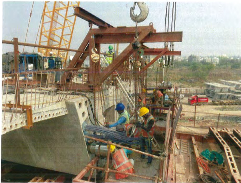
Photo No. 12: Span LMP 282-283, 1st stage stressing work in progress
