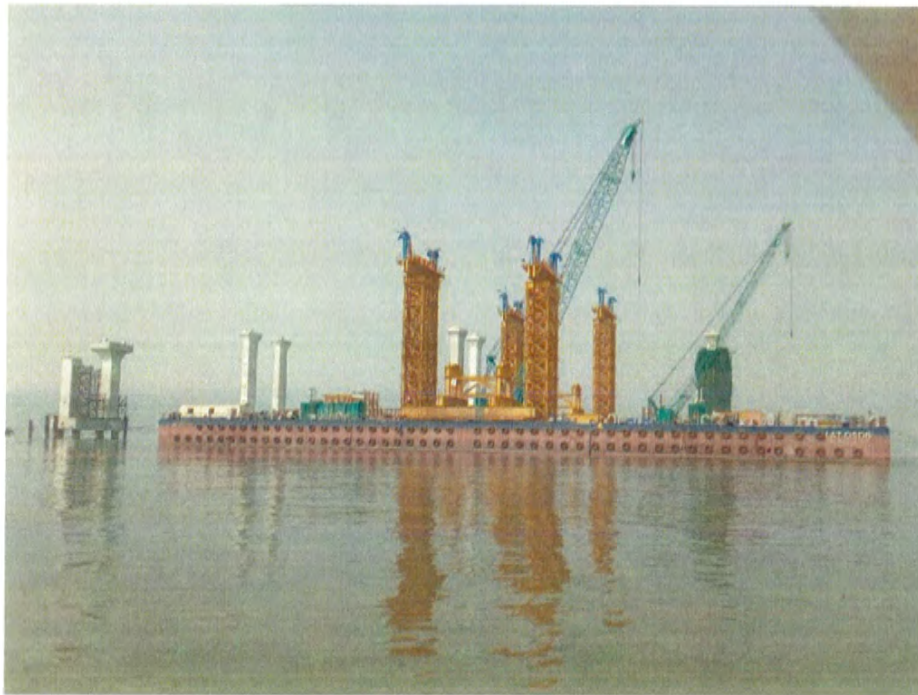
Photo No. 12: OSD barge at MP130 (Trussell erection) in progress
