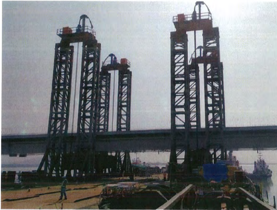
Photo No. 3: OSD lifted by Strand Jack for Load Test at Karanja Port in progress
