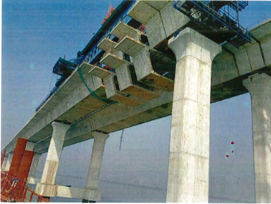
Photo No. 1: Erection of segment at Span MP47-48 south
