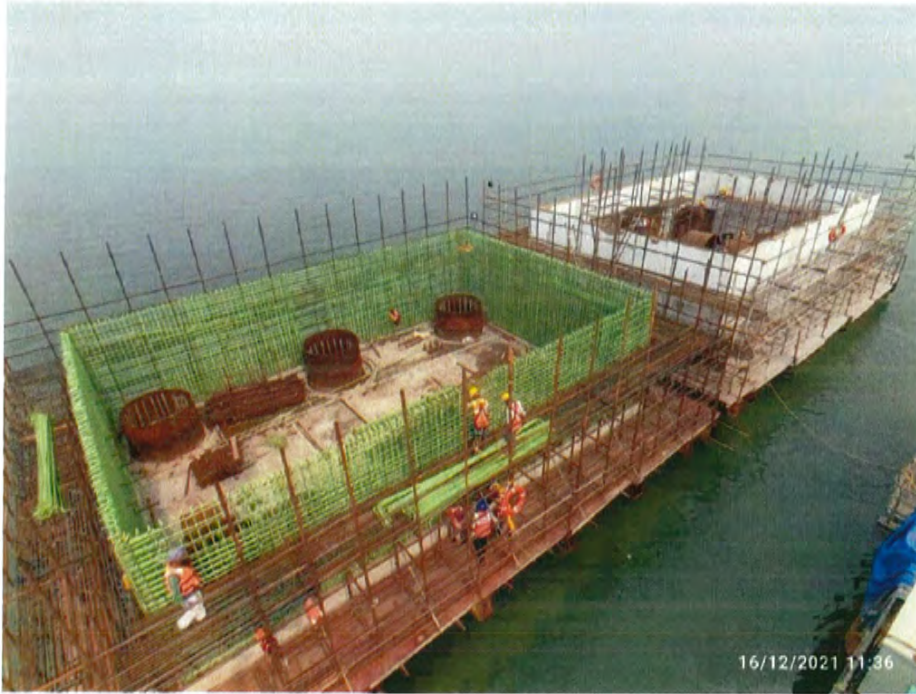
Photo No. 11: PC Shell wall reinforcement tying at MP 185 RHS in progress
