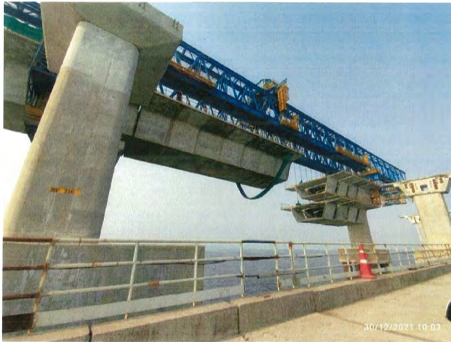
Photo No. 1: LG-1 Segment gluing at Span MP 215-216 RHS in progress
