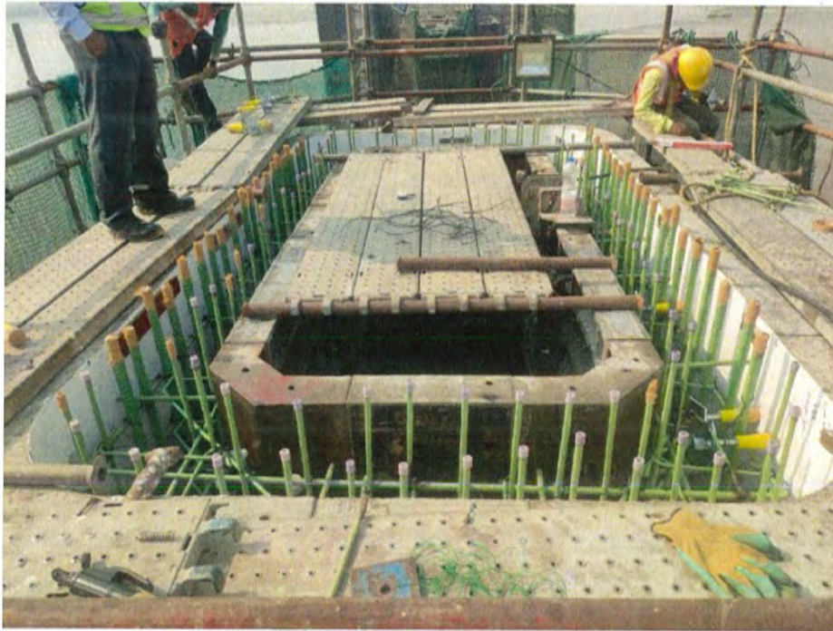
Photo No. 11: MP 68 S Pier Shuttering Works in progress
