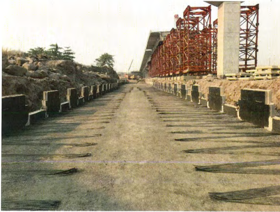
Photo No. 11: Jasai JM Ramp RE wall Panel erection in progress
