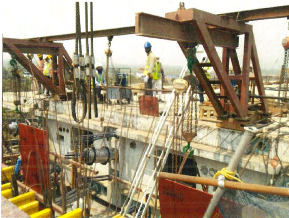
Photo No. 10: Gavan span RMP 269-270 1st stage prestressing work in progress
