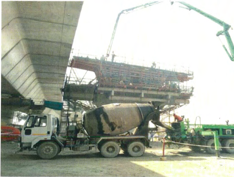
Photo No. 3: Pier head segment concrete at MP 246 RHS in progress
