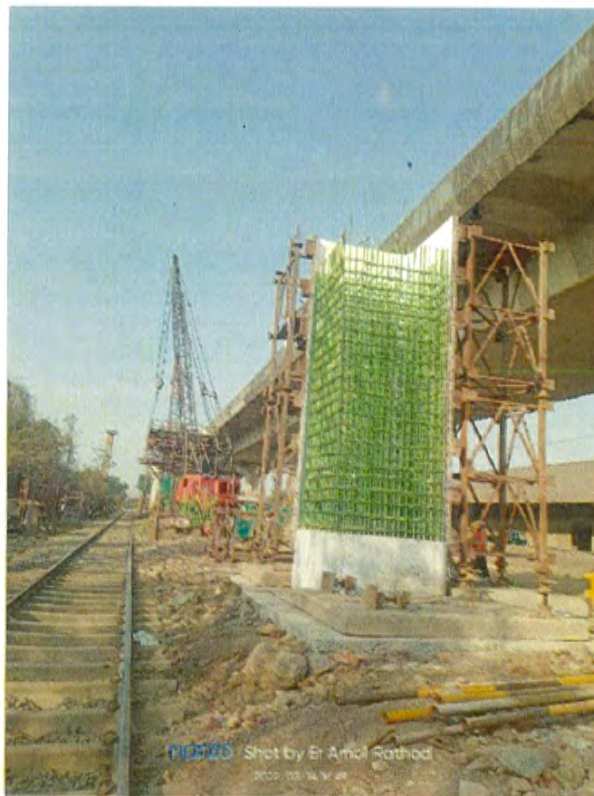
Photo No. 12: AP 08 Pier Reinforcement in progress
