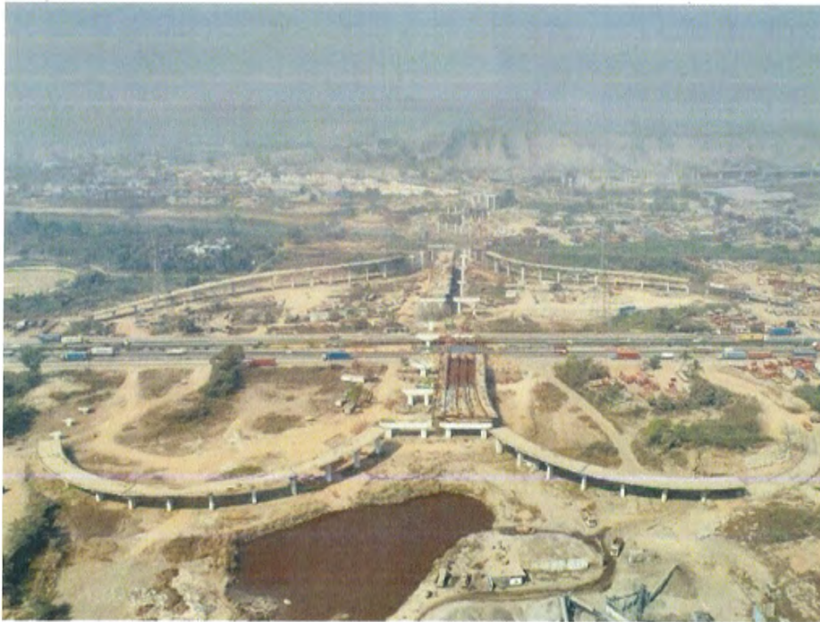
Photo No. 5: A view of MTHL Bridge at Chirle Interchange
