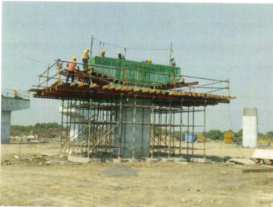
Photo No. 12: Pier cap reinforcement tying at CAP-4 in progress
