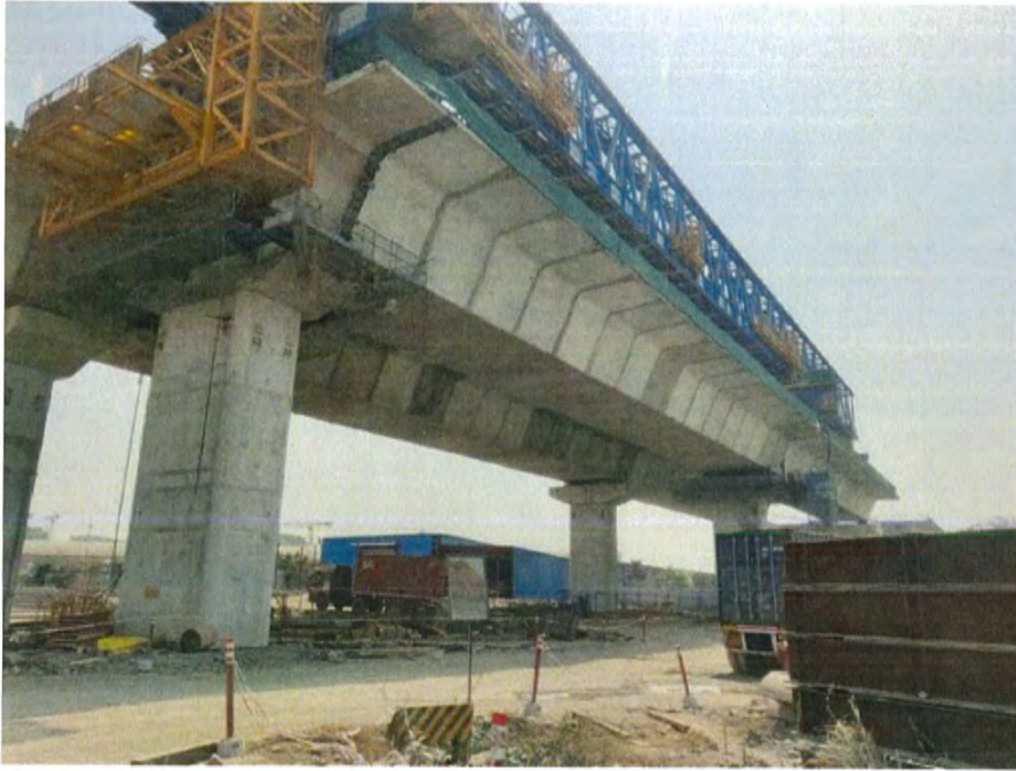
Photo No. 1: LG-3 Wet joint formwork fixing at Span MP 264-265 RHS in progress
