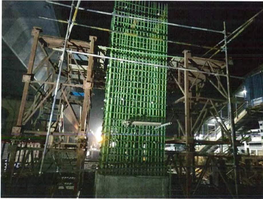
Photo No. 9: BP 13 Pier Reinforcement in progress
