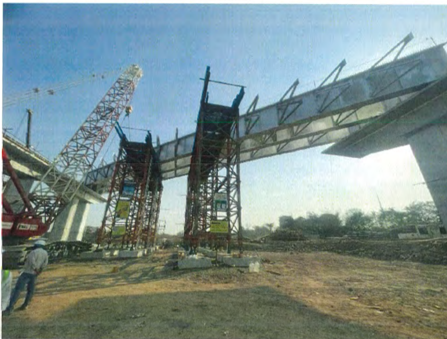
Photo No. 2: RMP 274-275 ROB structural steel erection work in progress
