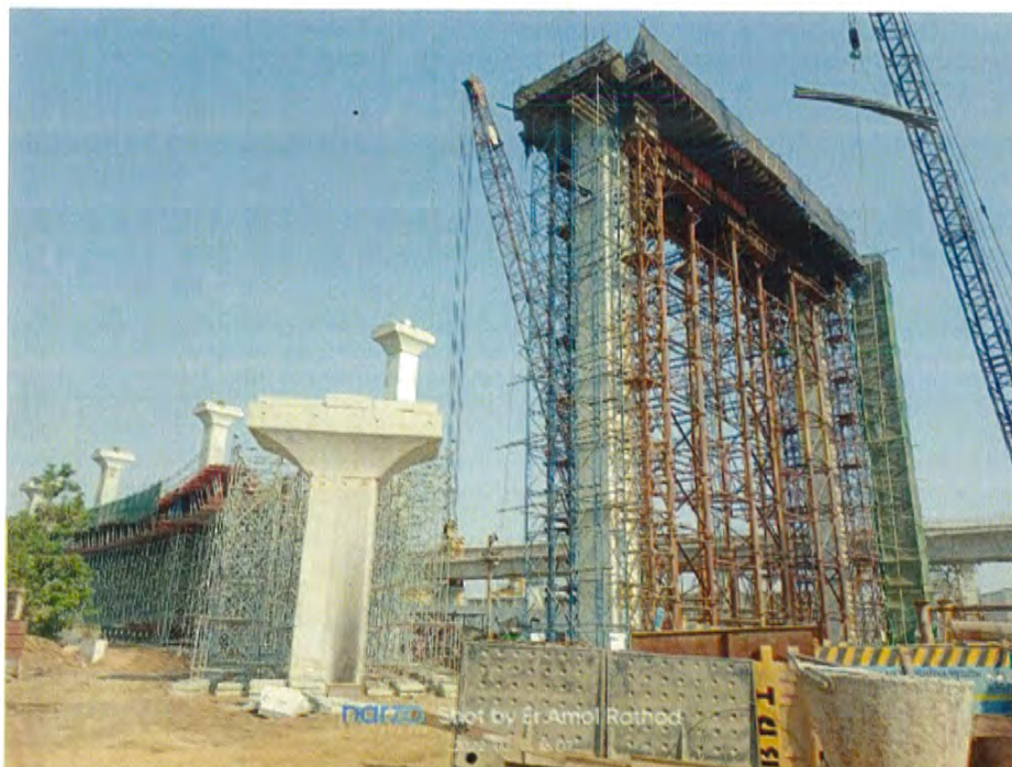
Photo No. 10: AP 41 Portal Beam Shuttering Works in progress
