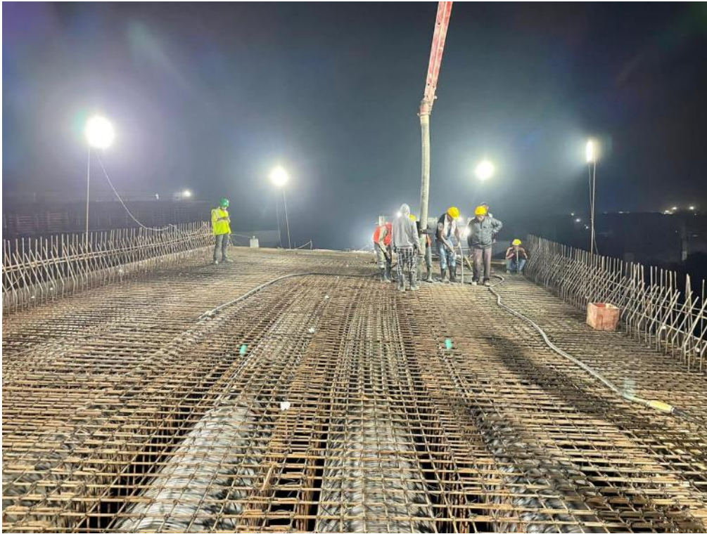
Photo No. 1: Voided slab MPP 9-8 concrete pouring in progress
