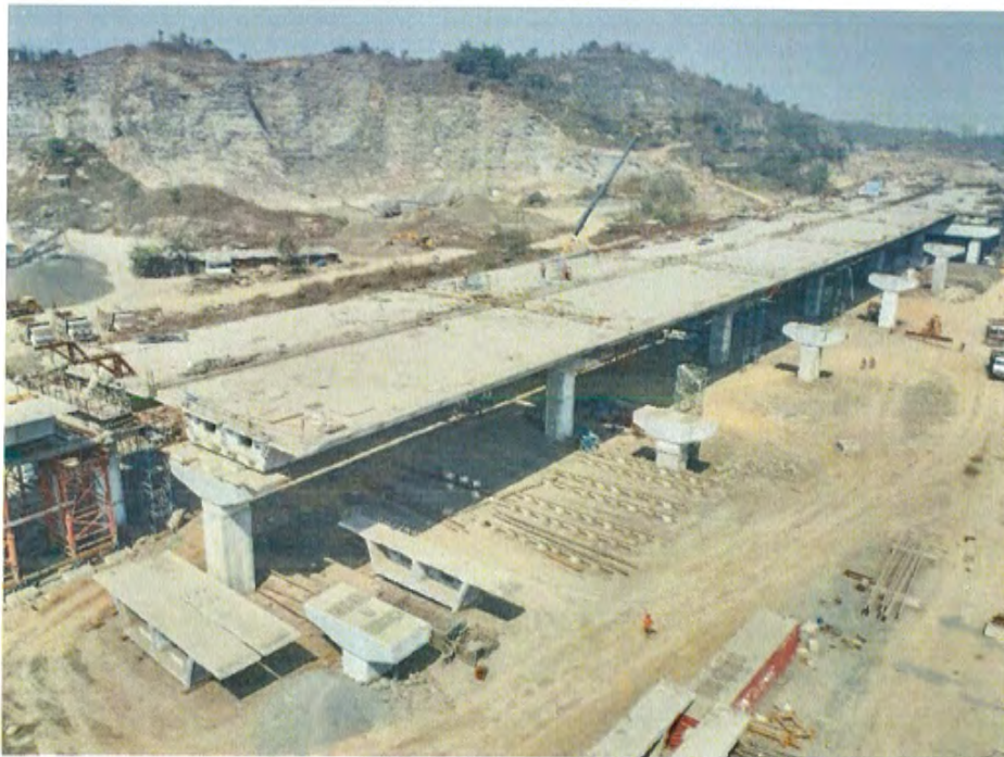
Photo No. 4: A view of MTHL Bridge at Jasai area
