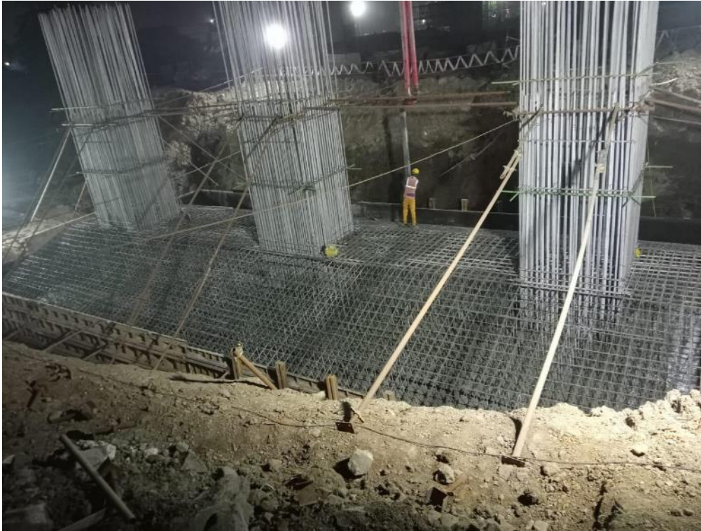
Photo No. 5: LP-24 foundation concrete pouring work in progress
