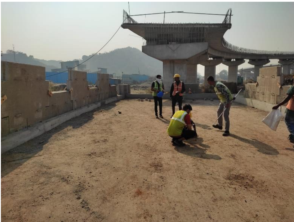
Photo No. 2: MJP Loop Chirle RE wall work in progress
