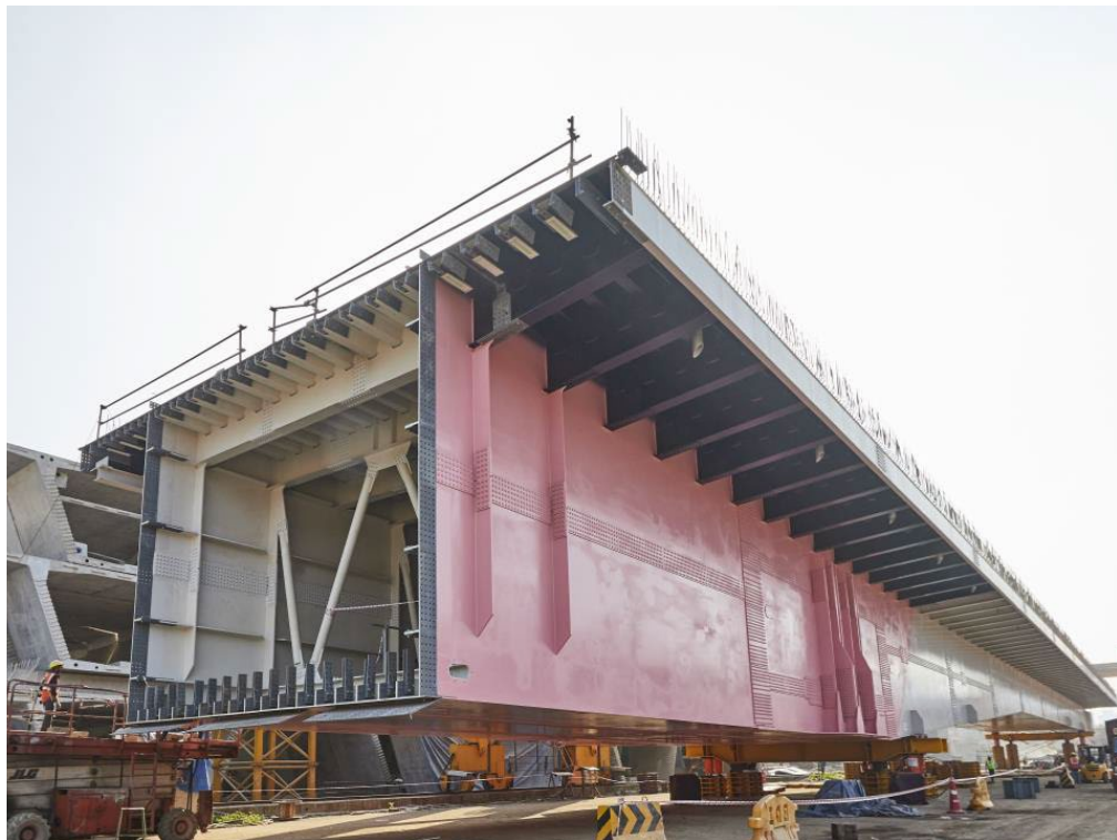
Photo No. 8: OSD04-N Assembly ready for loadout – Assembly Yard
