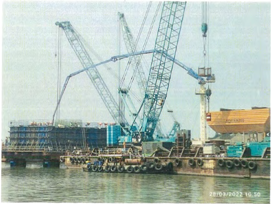
Photo No. 7: Pile cap concrete at MP 175 LHS in progress
