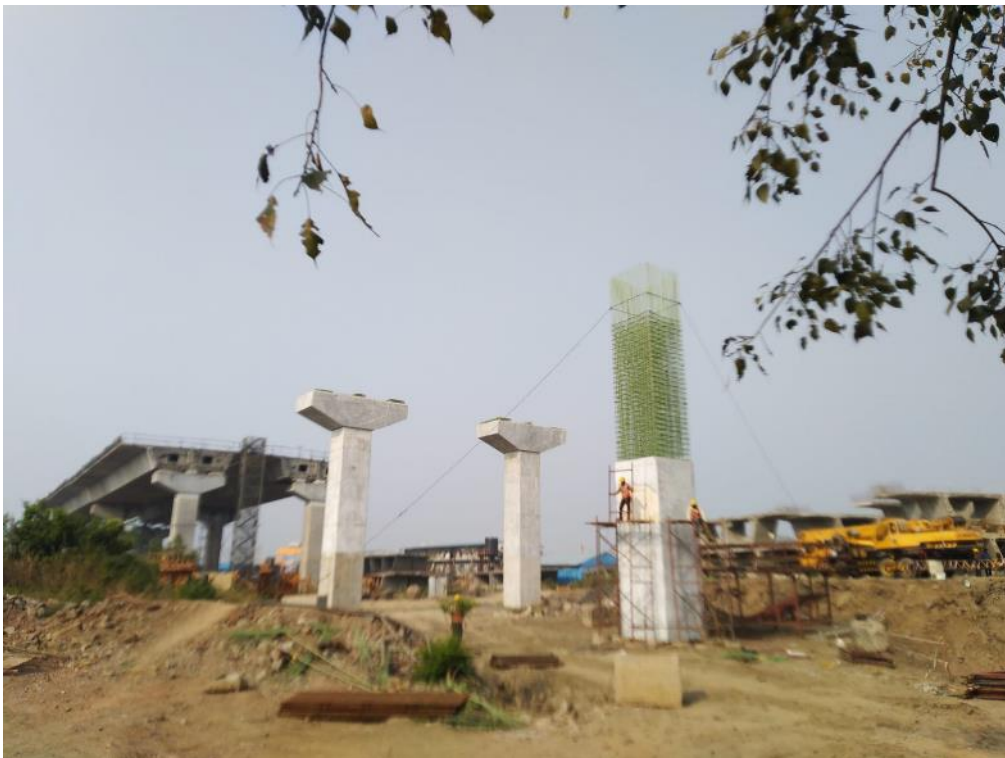
Photo No. 4: RMP 271 Pier 3rd lift Reinforcement work in progress
