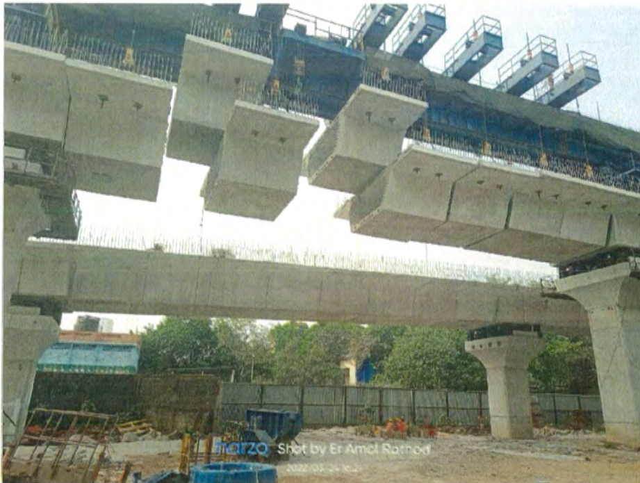
Photo No. 2: LG 6 EP 22-23 Segment lifting in progress
