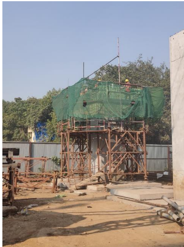
Photo No. 6: FP-03 Pier cap reinforcement activity in progress
