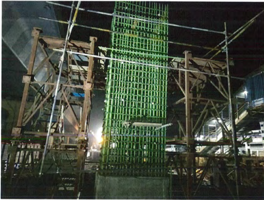
Photo No. 9: BP 13 Pier Reinforcement in progress
