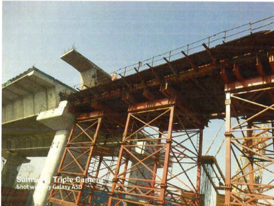
Photo No. 1: Gavan Span RMP 266-267, interface location, segment erection work in progress
