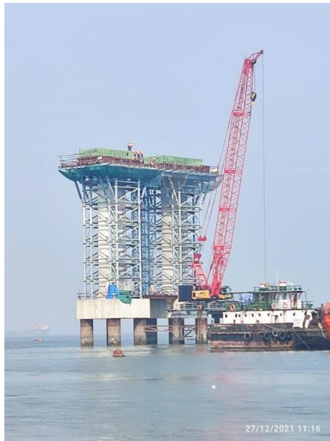
Photo No. 6: OSD Pier Cap reinforcement tying at MP 180 LHS and RHS in progress
