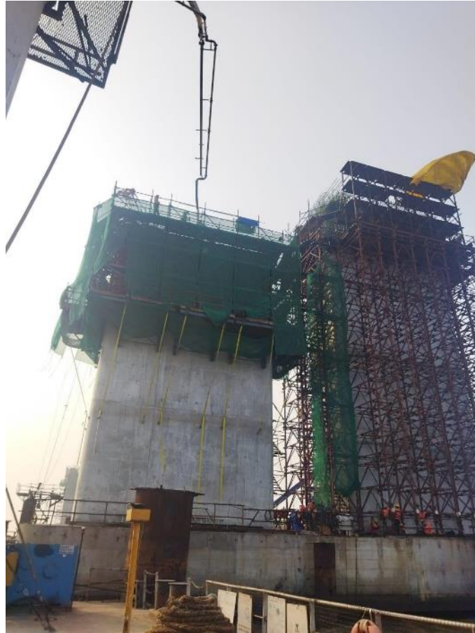
Photo No. 9: Concreting for Pier MP126 South in progress
