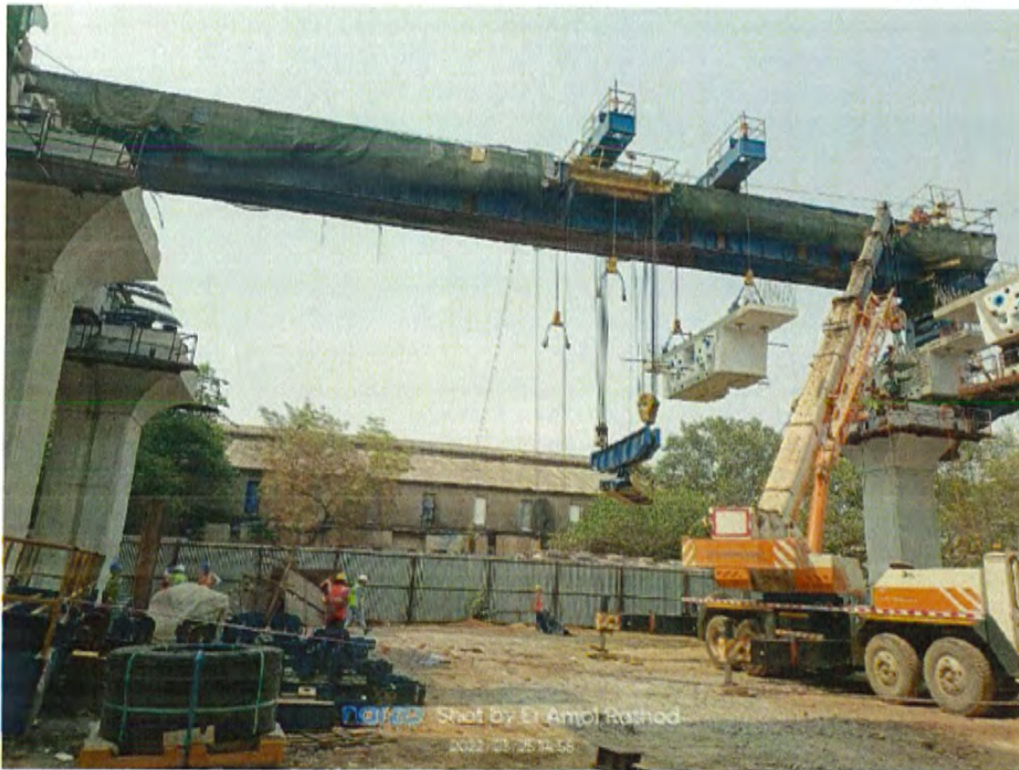
Photo No. 4: LG 05 FP 04-05 Segment lifting in progress
