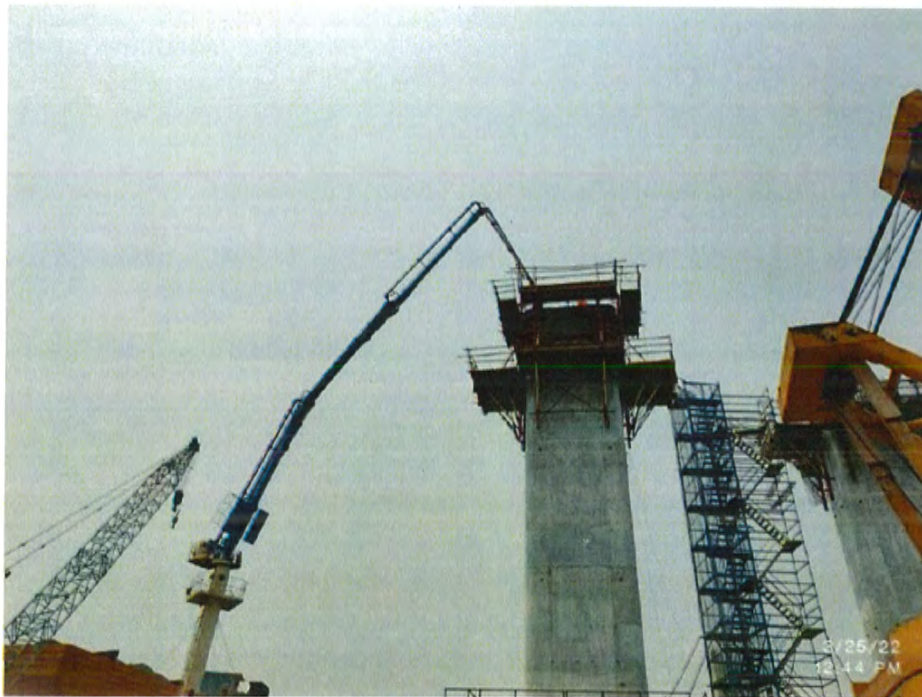
Photo No. 4: Pier final lift concrete at MP 167 LHS in progress
