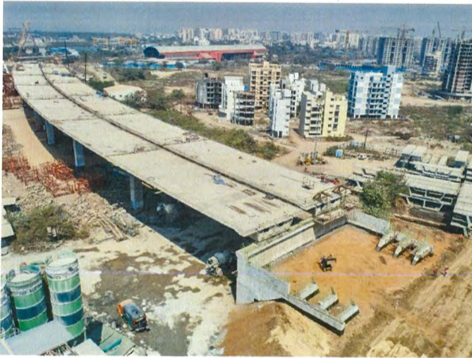
Photo No. 3: A view of MTHL Bridge at Gavan area
