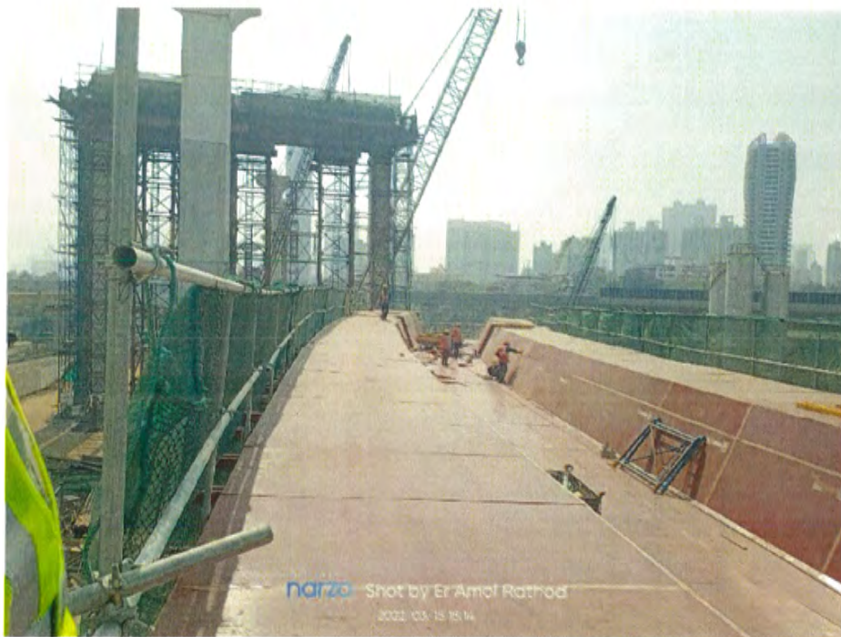
Photo No. 6: EP 14 Cast In-Situ Shuttering work in progress
