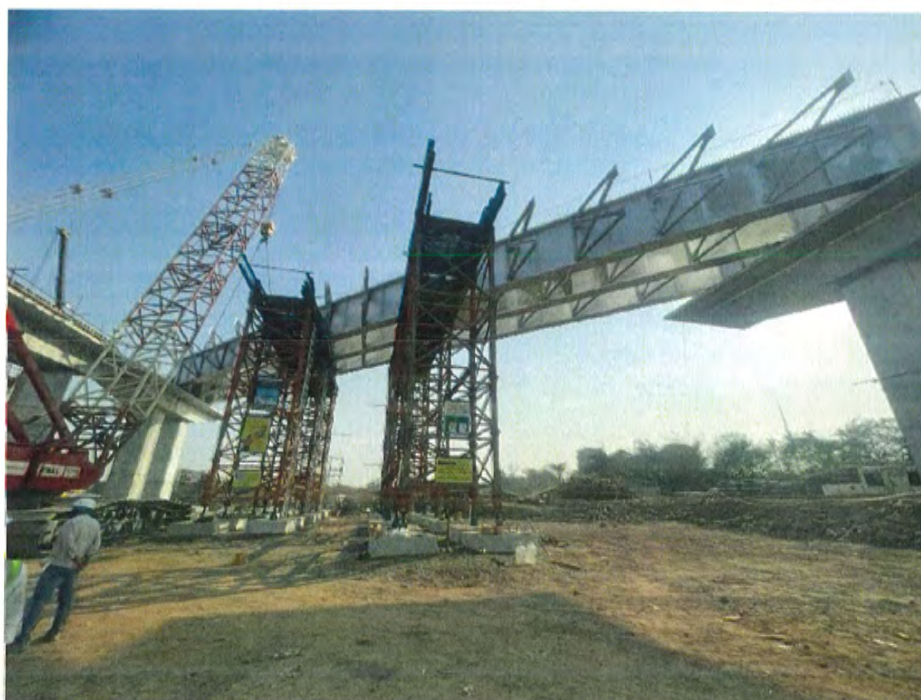
Photo No. 2: RMP 274-275 ROB structural steel erection work in progress
