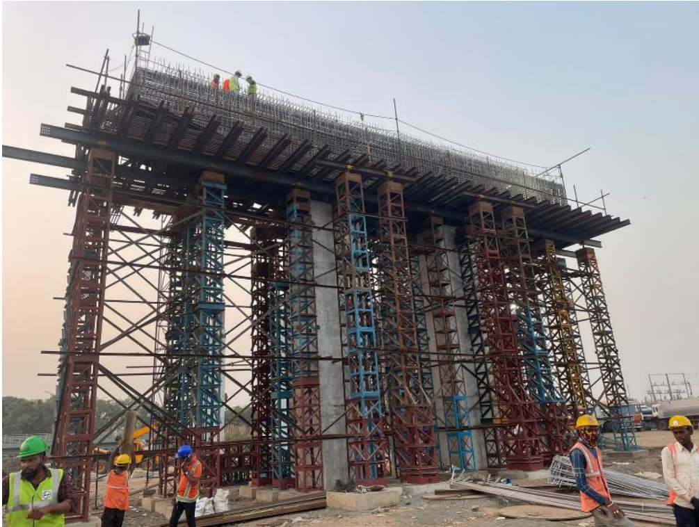
Photo No. 3: LMP 276 Portal Piercap reinforcement in progress
