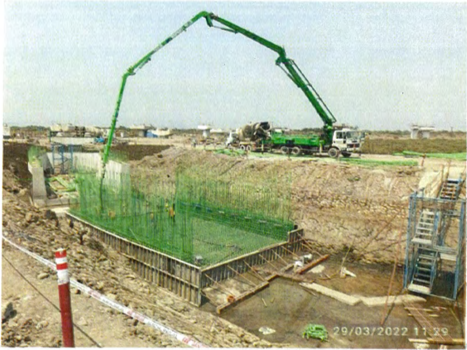
Photo No. 8: Retaining wall raft concrete at Ramp CA in progress
