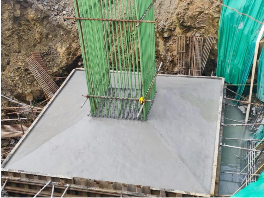
Photo No. 7: LMP 271 Foundation completed
