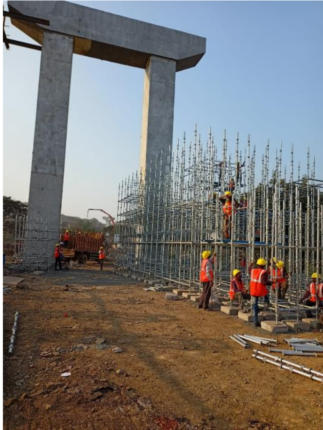
Photo No. 11: Span LP 22-23 Staging work for Cast-in-situ 3 Cell box girder in progress
