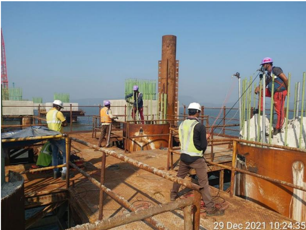
Photo No. 4: Sonic Tube Testing in progress at MP 170 RHS in progress
