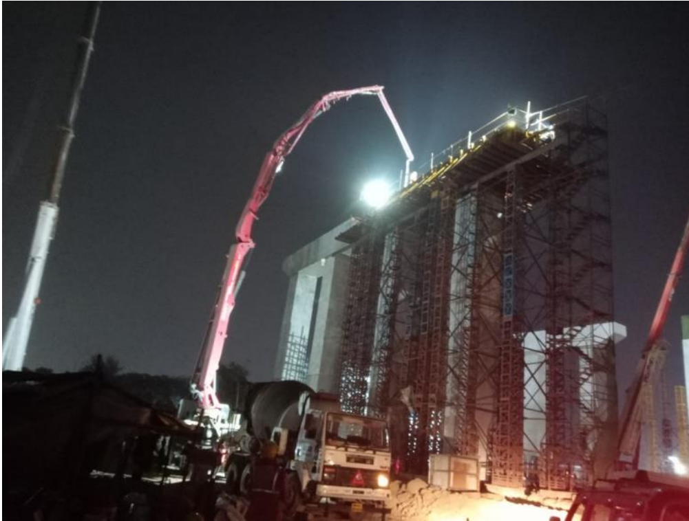
Photo No. 9: RP 22 Portal concrete pouring work in progress
