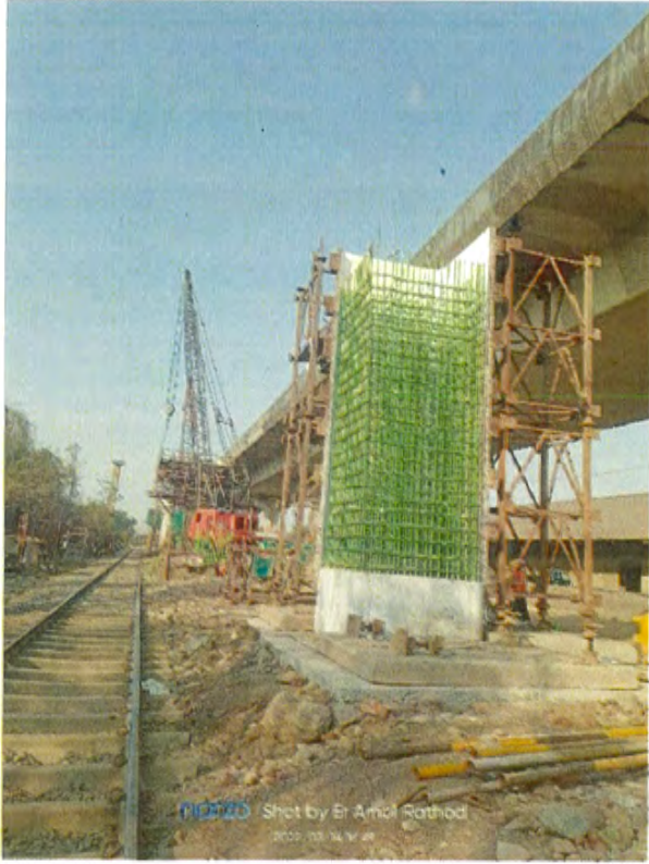
Photo No. 12: AP 08 Pier Reinforcement in progress
