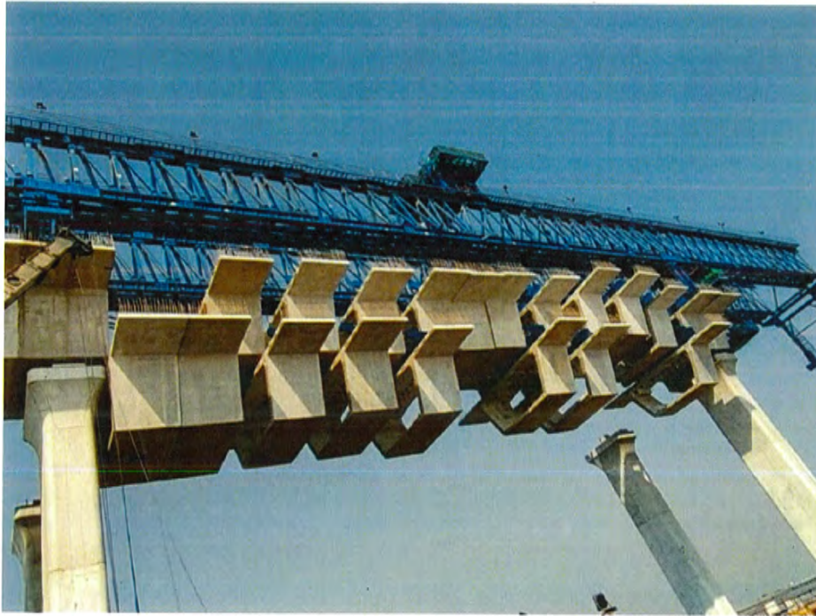
Photo No. 3: LG 08 MP 54-55 S Segment lifting in progress
