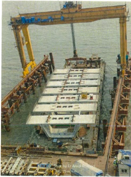
Photo No. 7: Segments Shifting to L-3 & 4 in progress
