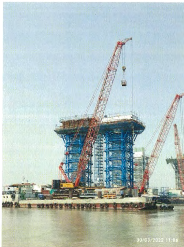
Photo No. 10: Pier cap reinforcement tying at MP 177 RHS in progress
