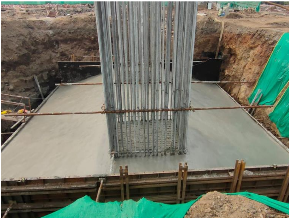
Photo No. 6: LMP 273 Foundation completed
