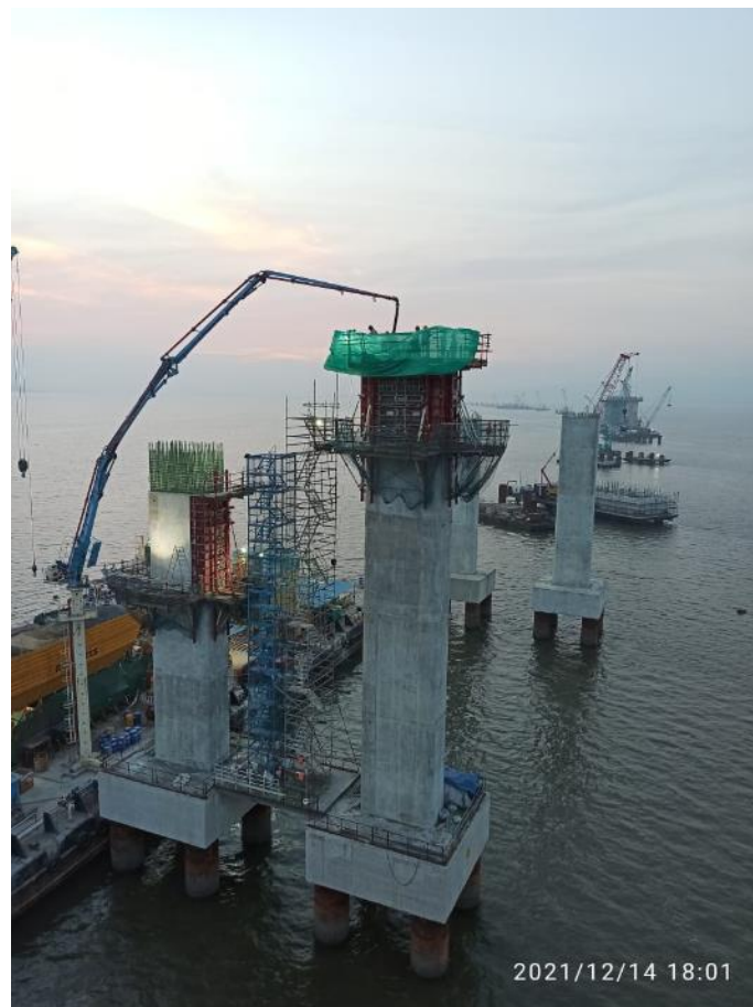
Photo No. 12: Pier final lift concreting at MP 187 LHS in progress
