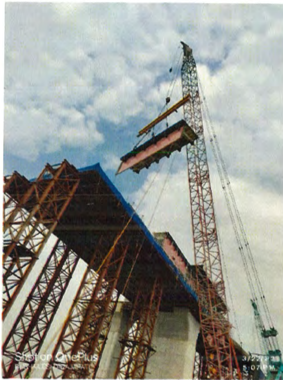
Photo No.8: OSD-1 assembly works in progress
