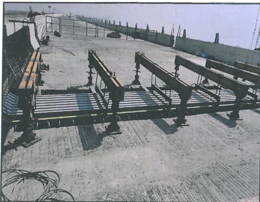
Photo no.6 Intertidal Section- Ej Fixing Trail Work At MP-20
