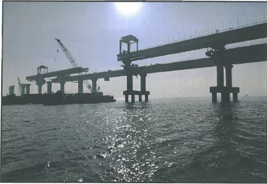
Photo no.9 Marine Section- LG-4 MP 104-105 N
