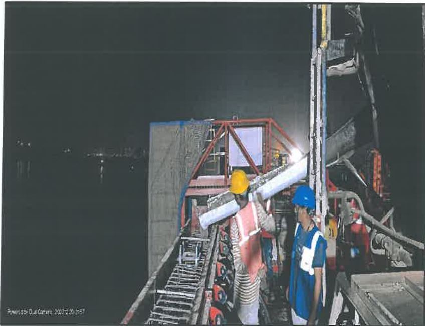
Photo no.8-Crash barrier concrete in progress at Span MP 212-213 LHS.
