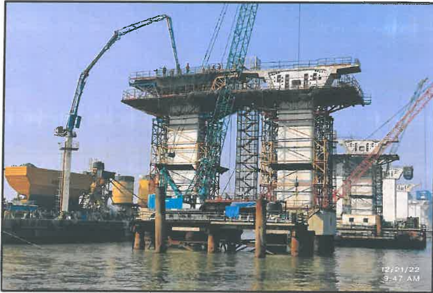
Photo no.7-Integral Pier Head Segment concrete in progress at MP 160 RHS.
