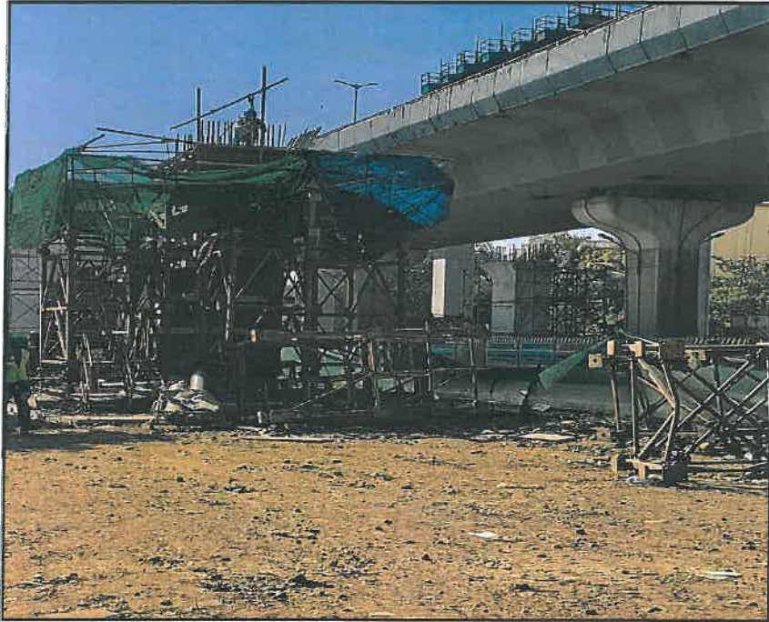
Photo no.3 Interchange Section - C1P8 Pier Shutter
