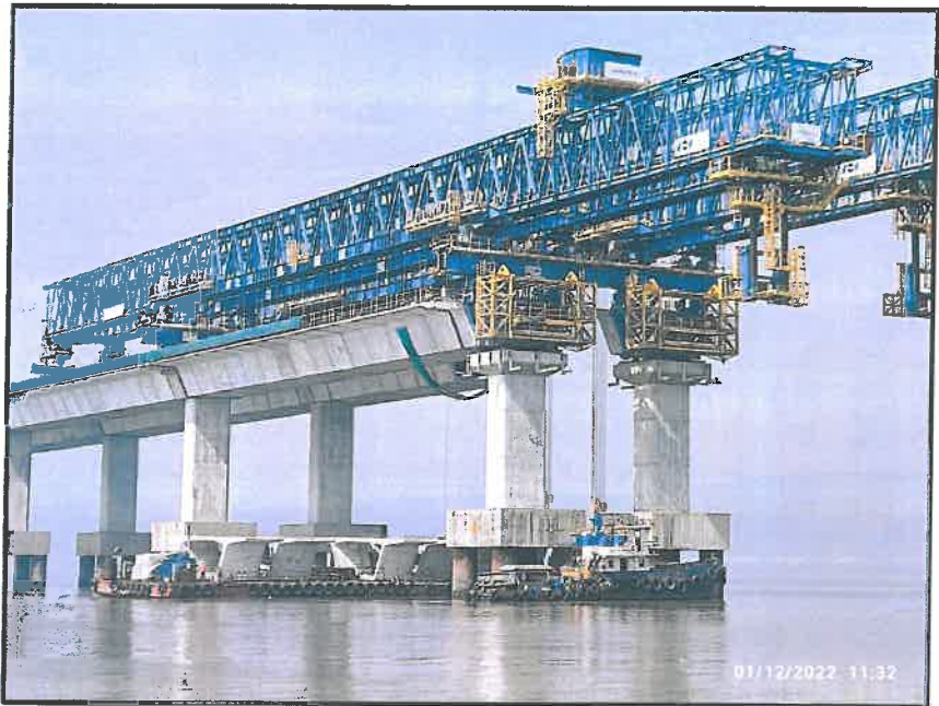
Photo no.12- Wet joint formwork in progress at span MP 152-153 RHS and segment lifting in progress at span MP 152-153 LHS.
