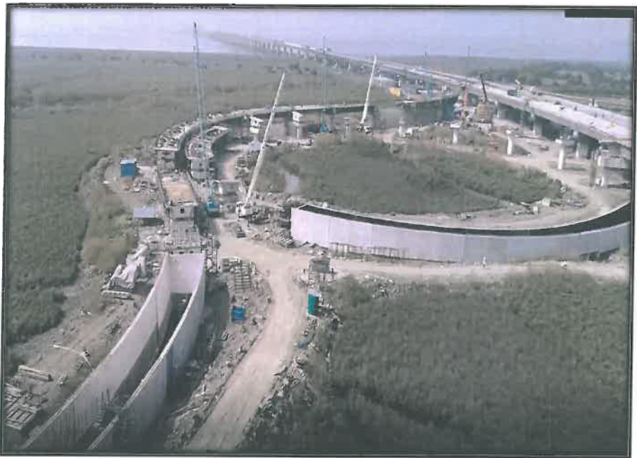
Package-2 Aerial View
