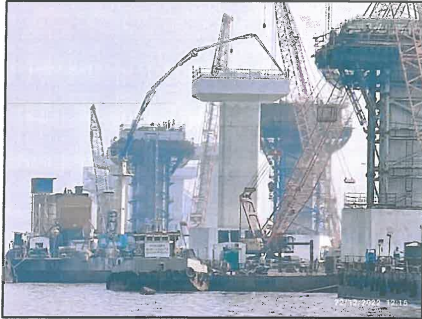
Photo no.5-Pier cap concreting in progress at MP 173 LHS.
