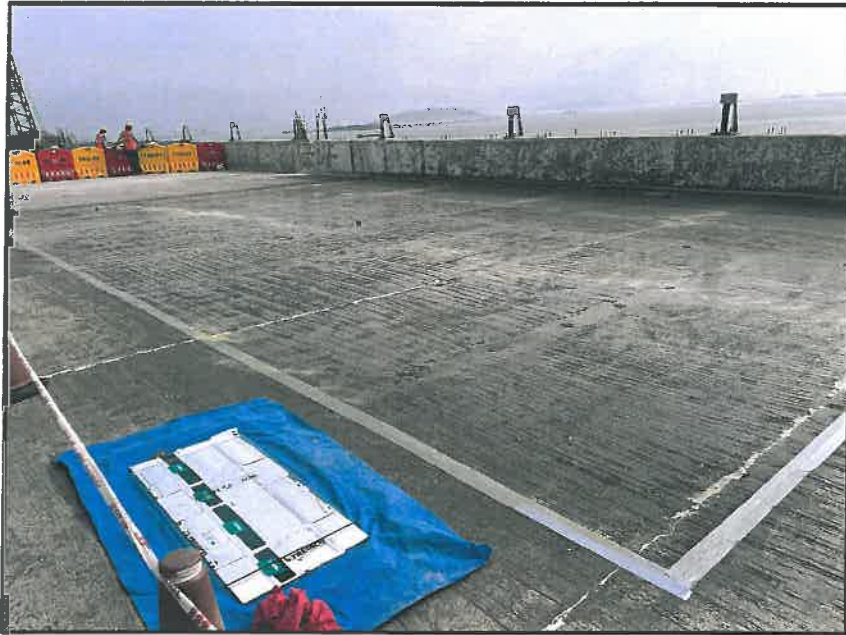
Photo no.7 Intertidal Section- Surface Preparation Work For Water Proffing Mockup
