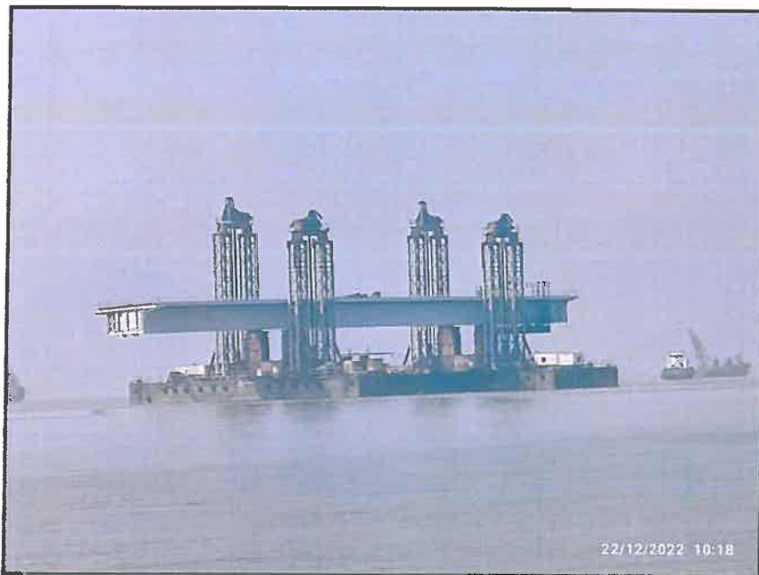
Photo no.4-15th OSD span for arrived at Marine Parking.
