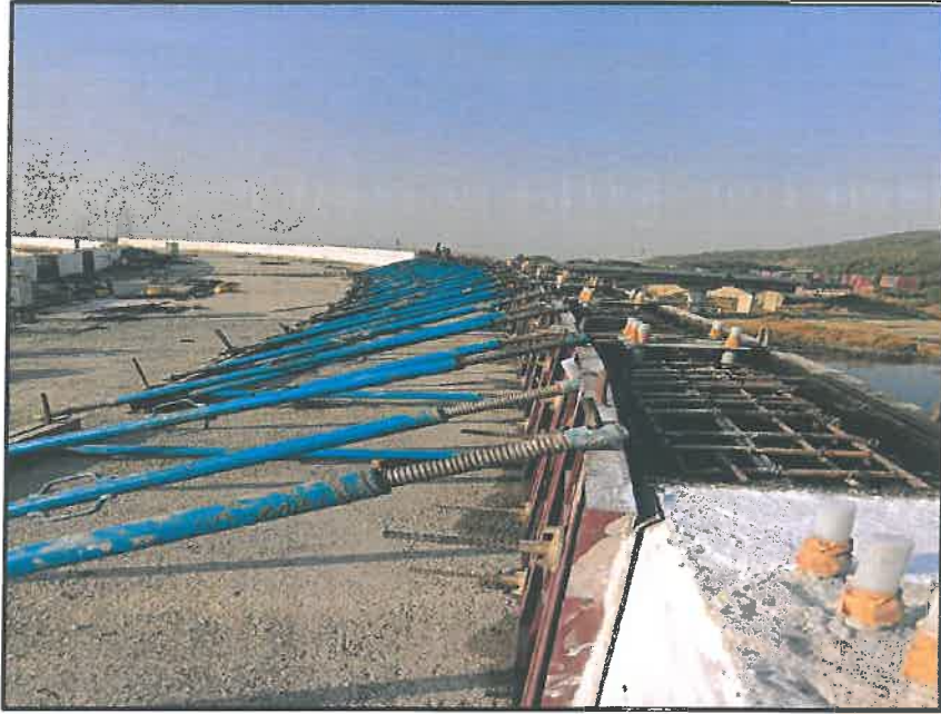
Photo no.1- Chirle Ramp PMP outer crash barrier shuttering work.
