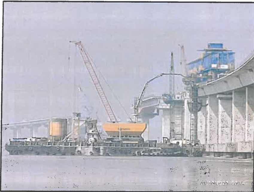
Photo no.3- Pier final lift concreting in progress at MP 191 RHS Substation.
