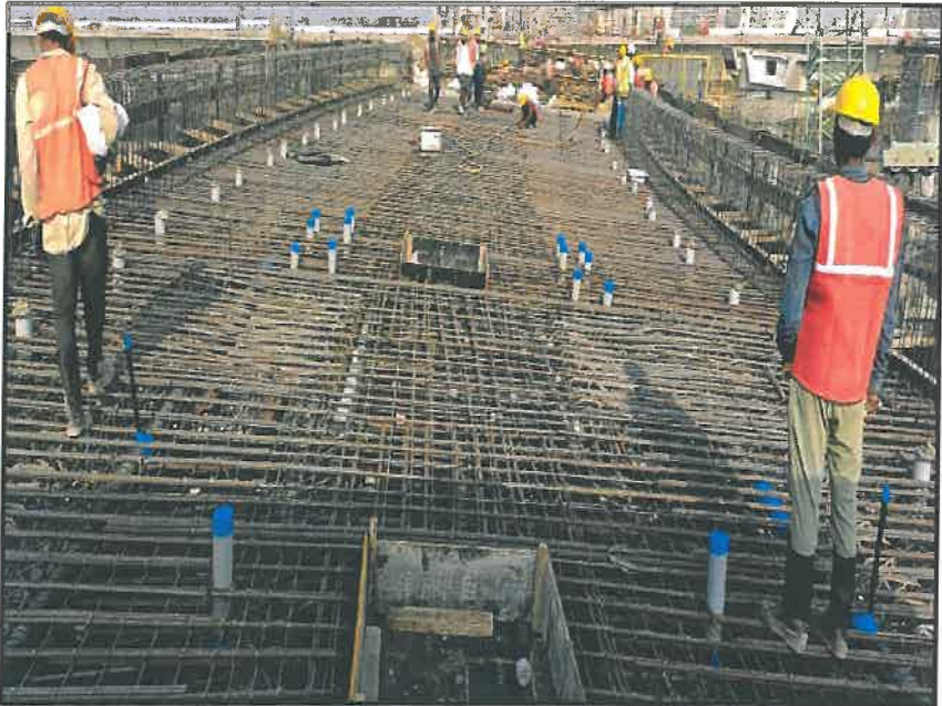
Photo no.1-Ramp CA- Top slab side formwork alignment in progress at Span CAP-4 to CAP-5.
