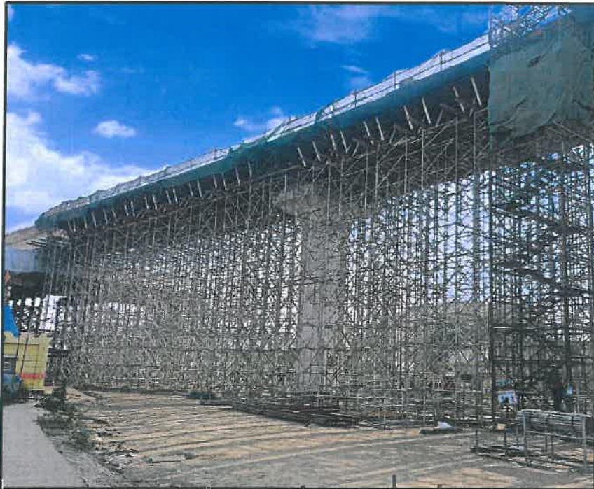
Photo no.4 Interchange Section - BP31- BP33
