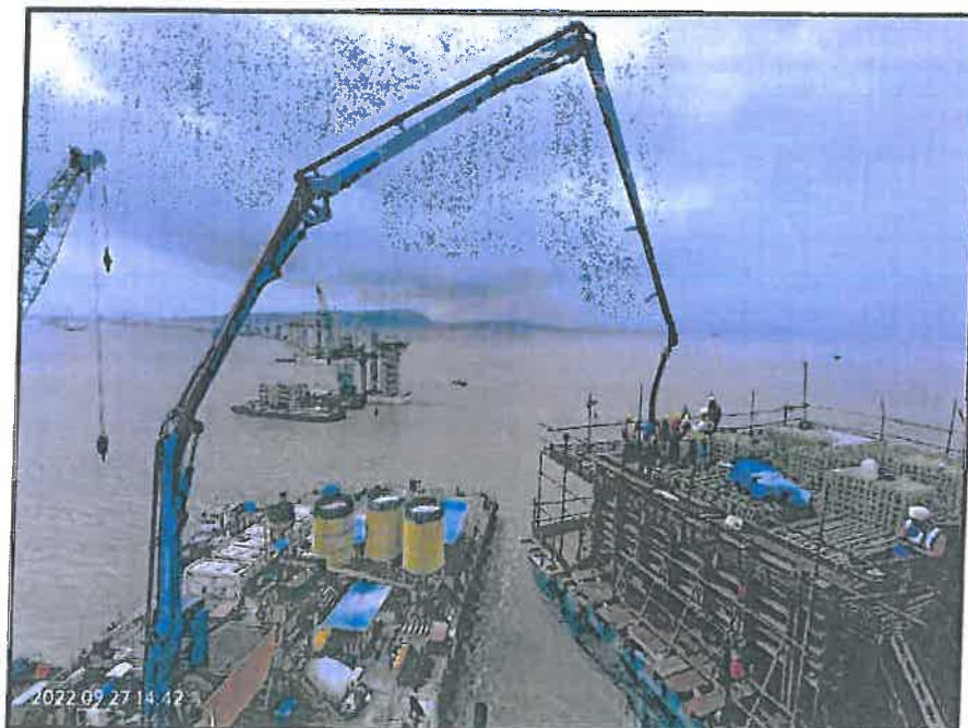
Photo No. 4: Pier cap concrete at MP 185 RHS in progress
