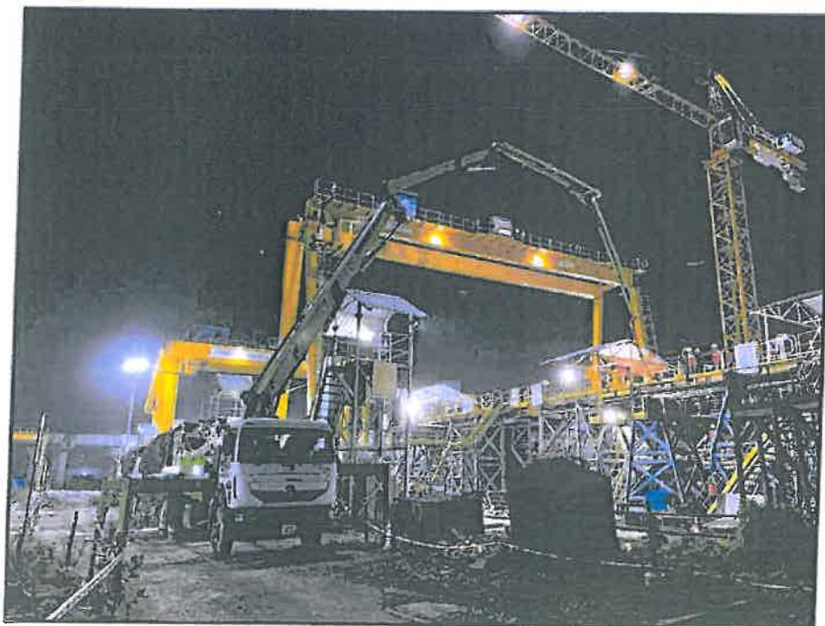
Photo No. 2: Segment concreting at Bay-3 in progress
