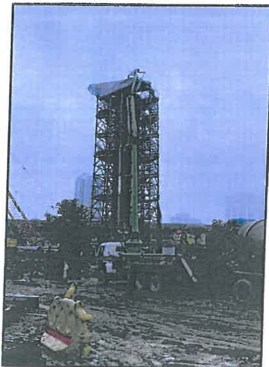
Photo No. 7: AP 35 Pier cap casting in progress
