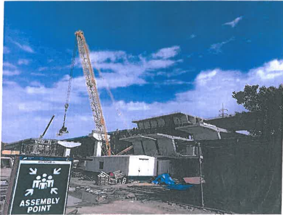
Photo No. 9: Chirle span LP32-33 segment erection work
