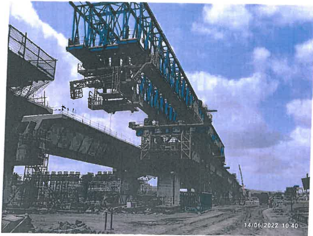
Photo No. 1: LG-3 Wet joint formwork fixing at Span MP 253-255 RHS in progress
