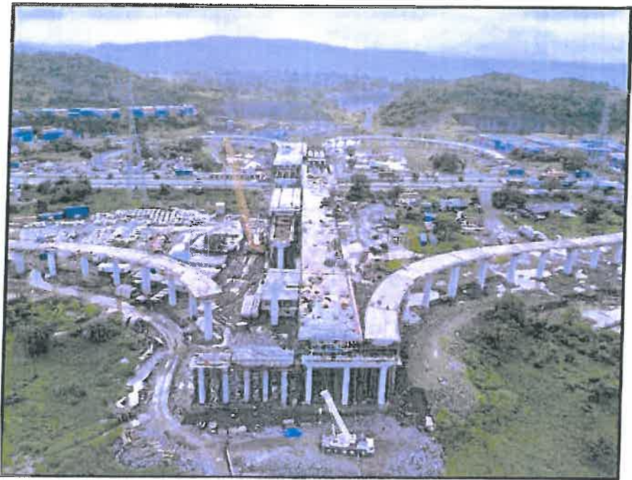
Photo No. 5: Chirle Interchange works in progress
