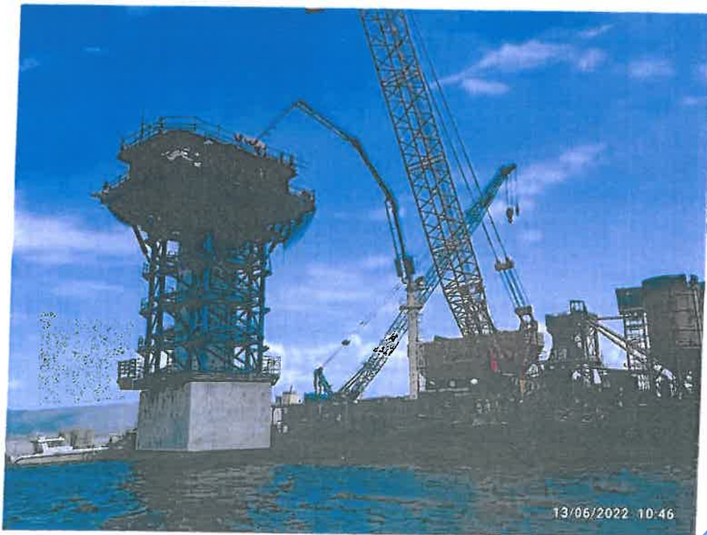
Photo No. 2: Pier cap concrete at MP 173ARHS in progress
