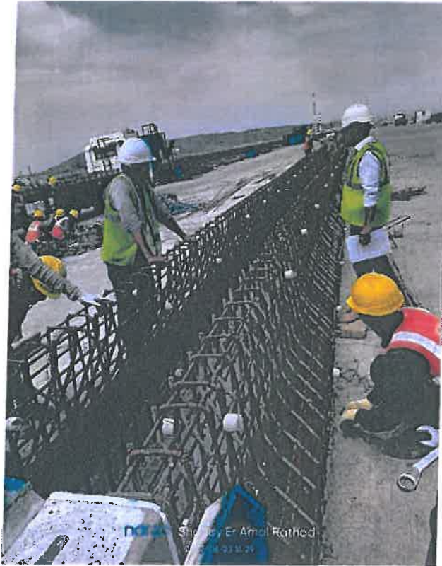
Photo No. 11: Median Crash Barrier Reinforcement in progress
