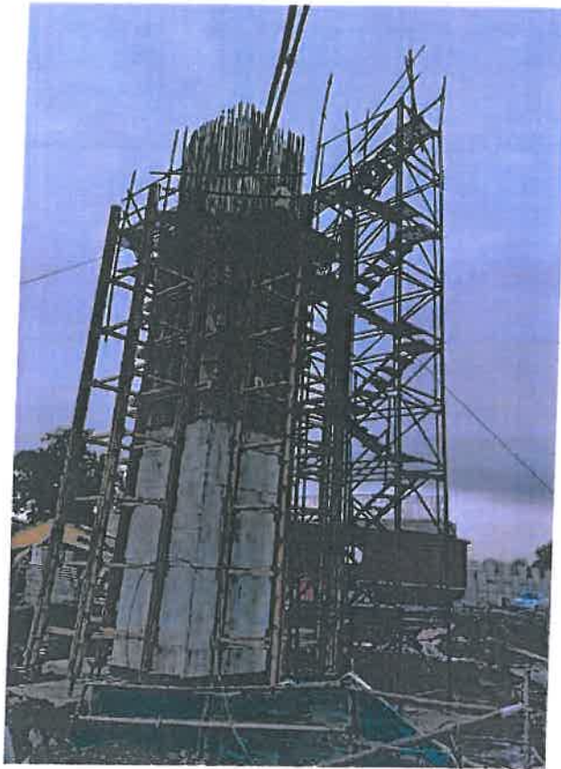
Photo No. 11: Jasai LP-20, Pier 3rd lift concrete work
