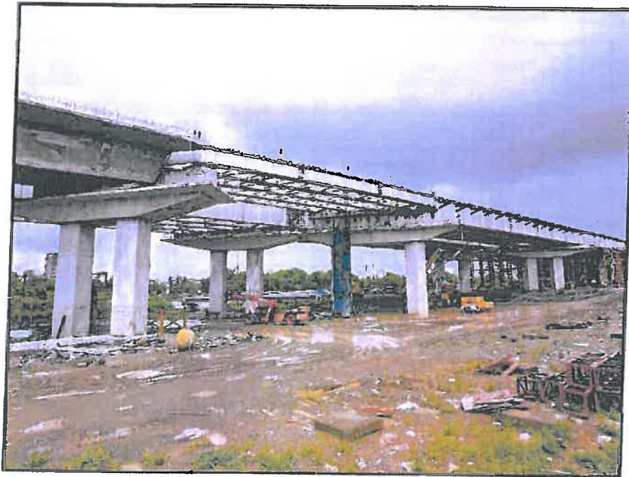
Photo No. 1: Gavan ROB structural works in progress
