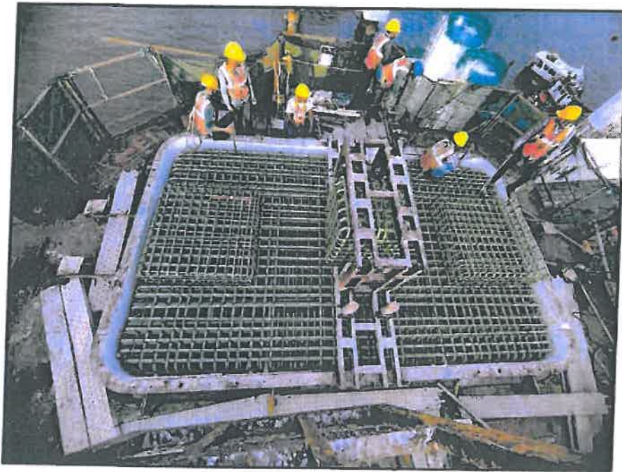
Photo No. 4: MP 113 S Pier Head Shuttering
