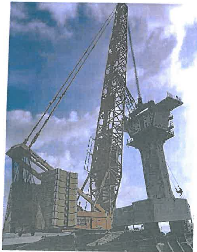
Photo No. 10: LG 1 Pier Head Lifting in progress
