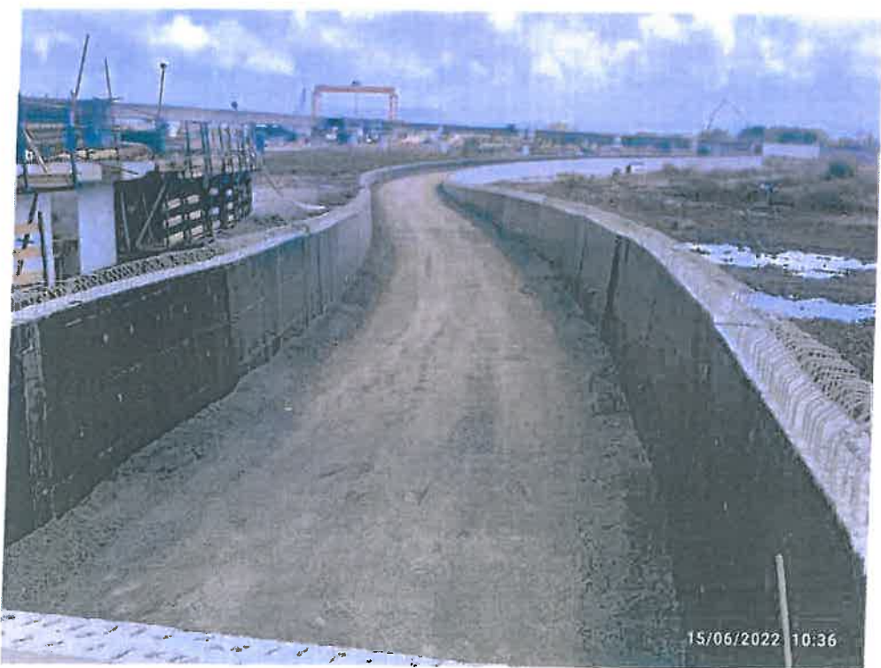
Photo No. 8: Retaining wall backfilling works at ramp Area in progress
