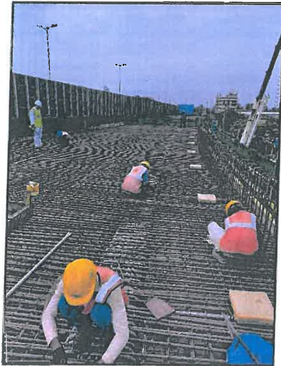
Photo No.8: EP 08-09 Top slab Cast in situ reinforcement in progress
