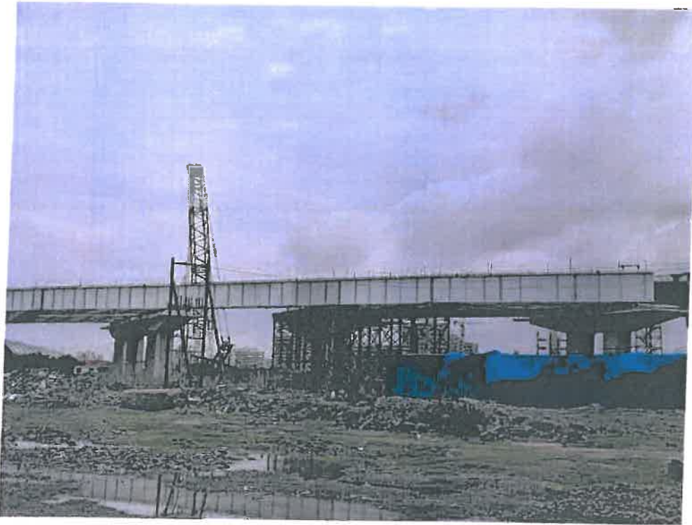
Photo No. 1: Gavan Span RMP 275-276 ROB structural steel Girder erection completed
