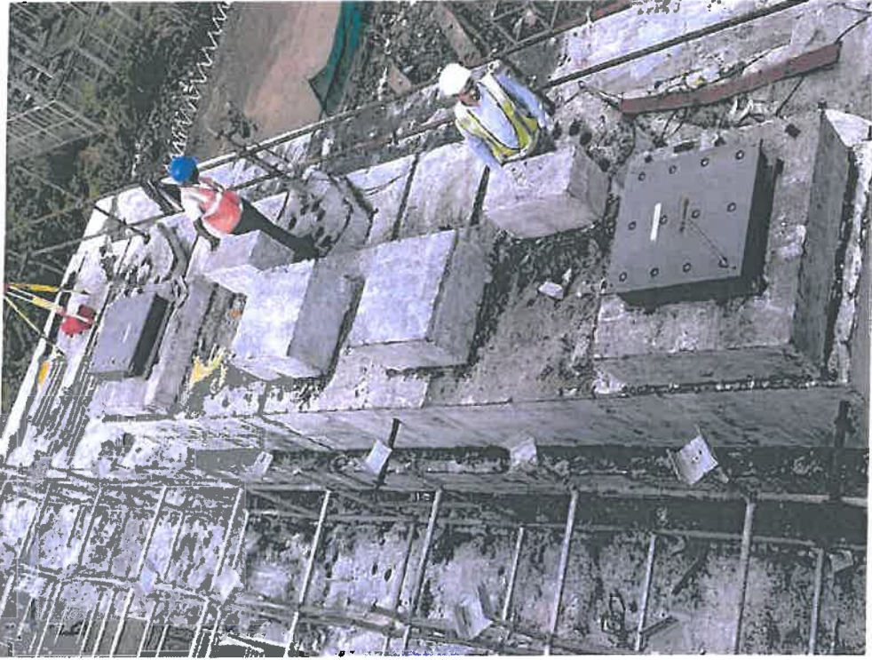
Photo No. 5: Pier LMP 273 Bearing Installation survey Inspection work
