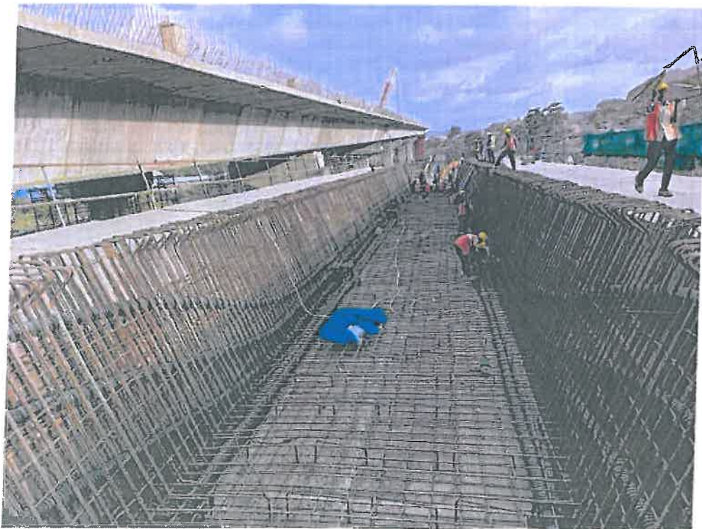
Photo No. 4: Jasai span JMP 04-05 reinforcement and profile work
