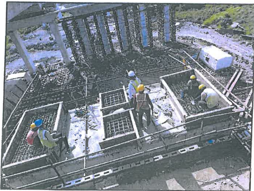
Photo No. 8: Chirle Pier cap LP 30 pedestal & seismic arrester pre-pour inspection works in progress
