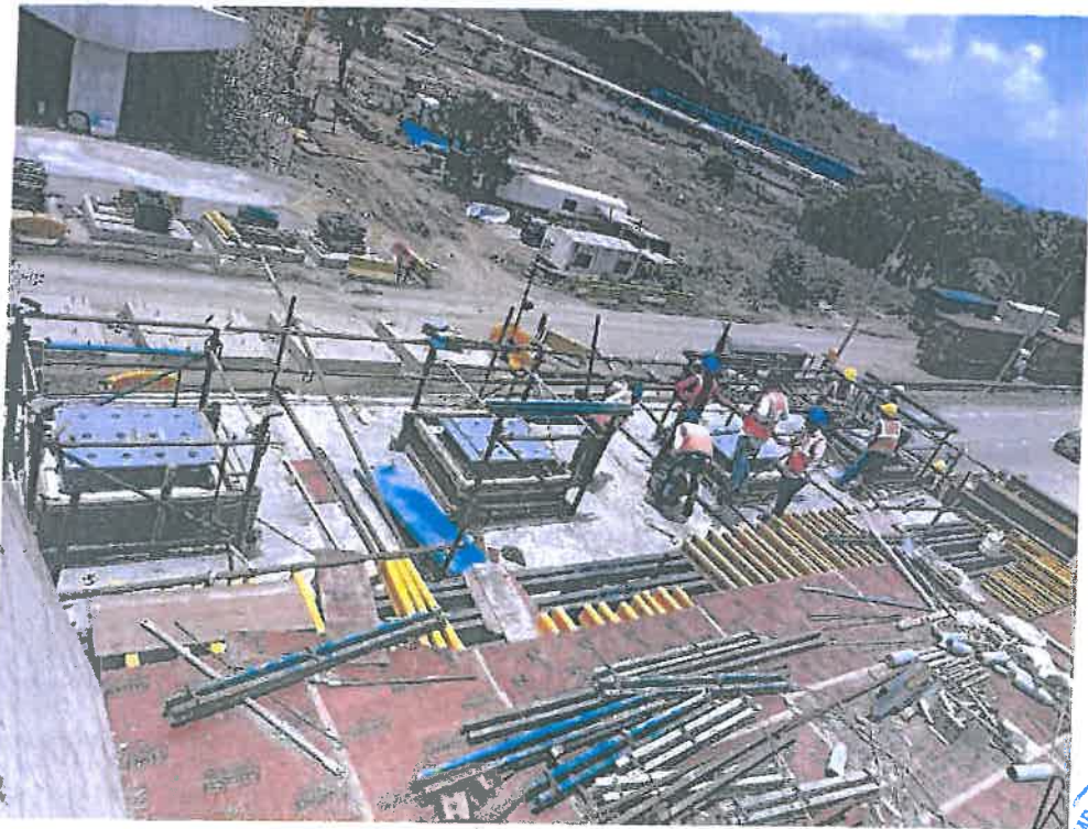
Photo No. 8: Chirle RP-35 Bearing installation survey work
