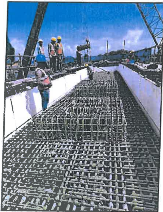
Photo No. 6: BP 33 Portal Pier Cap in progress
