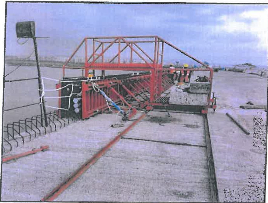
Photo No. 3: Outer Crash barrier formwork alignment at Span MP 222-223 LHS in progress
