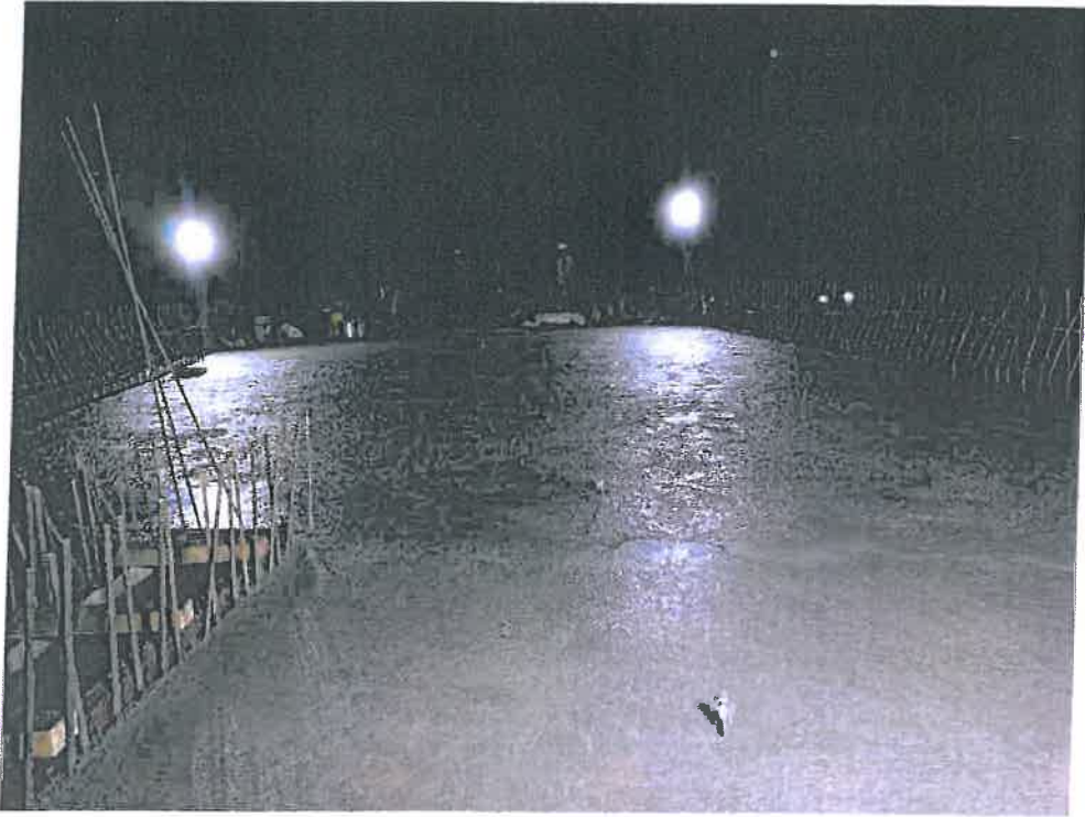
Photo No. 3: Chirle interchange ramp MJ1-2 voided slab concrete casting completed
