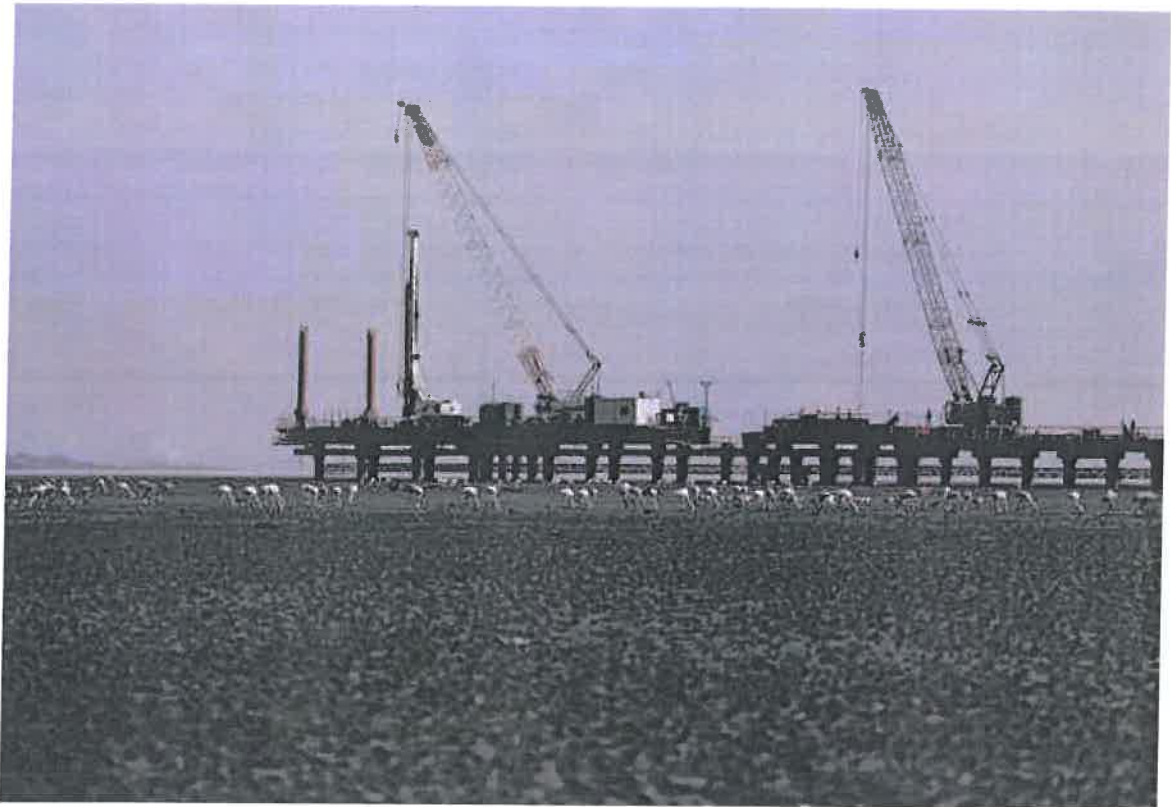
Sewri Construction site
