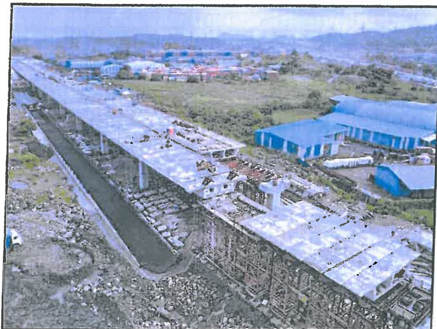
Photo No. 4: Jasai viaduct works in progress
