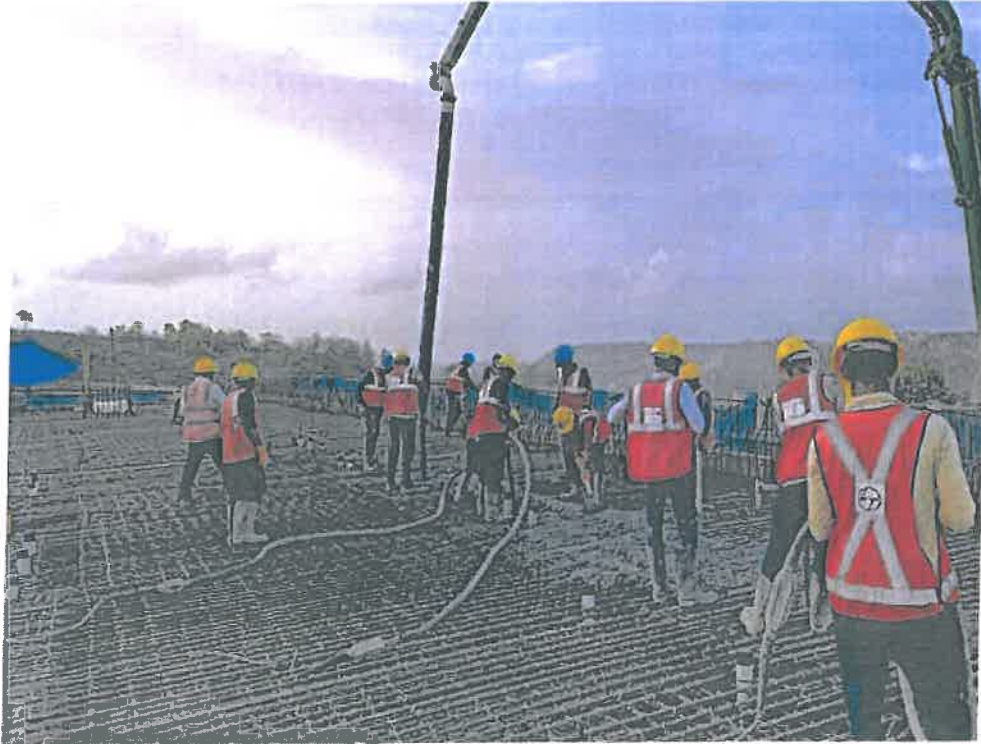
Photo No. 6: Jasai span LA01-LP01 deck slab concrete pouring work
