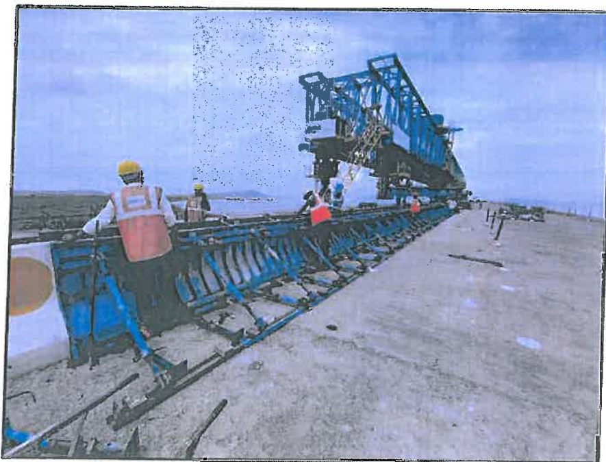
Photo No. 6: Median side crash barrier formwork fixing at Span MP 234-235 LHS in progress
