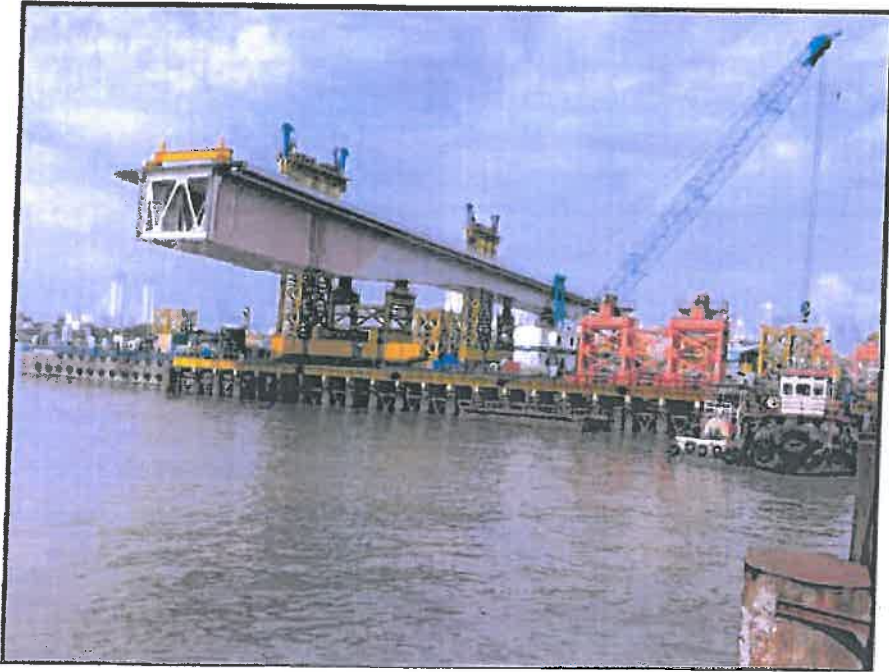
Photo No. 2: OSD 2 SPAN 1SOUTH MP 69-70 loading out in progress
