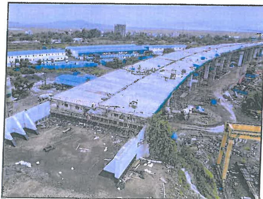
Photo No. 2: Gavan superstructure works in progress
