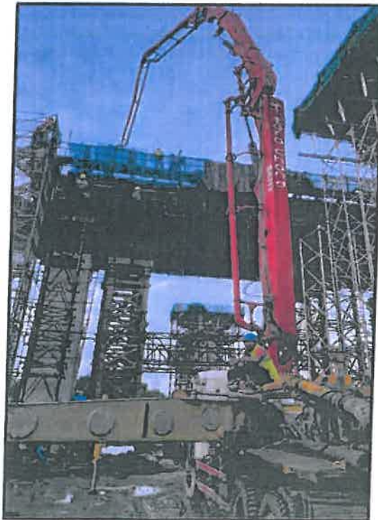
Photo No. 11: BP 33 portal pier cap casting in progress
