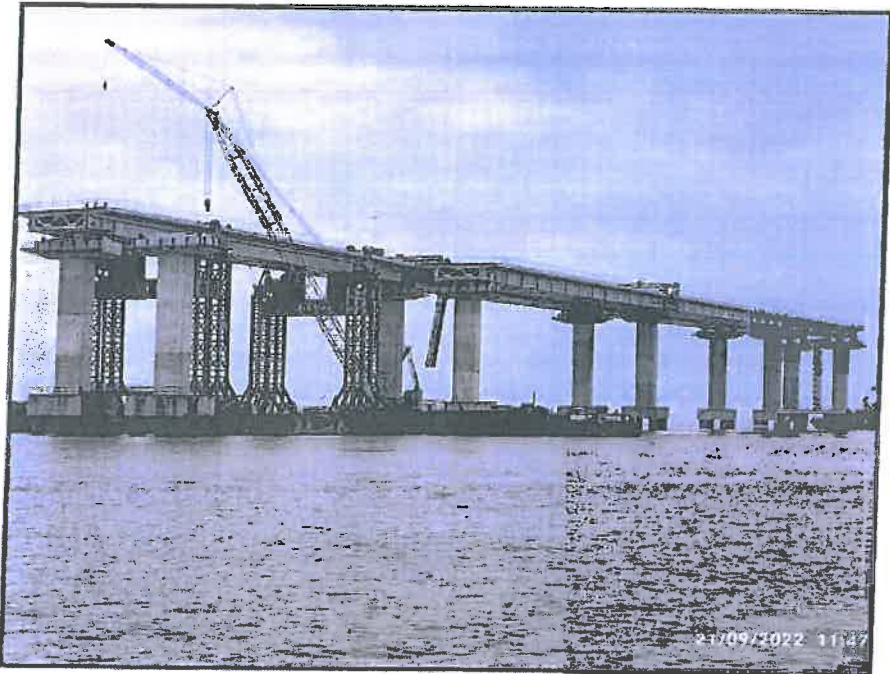
Photo No. 10: 7th OSD span erection at Span MP 178-179 LHS in progress
