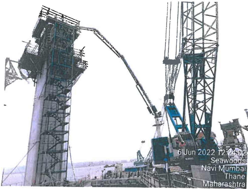
Photo No. 5: Pier final lift concreting at MP 184 RHS in progress
