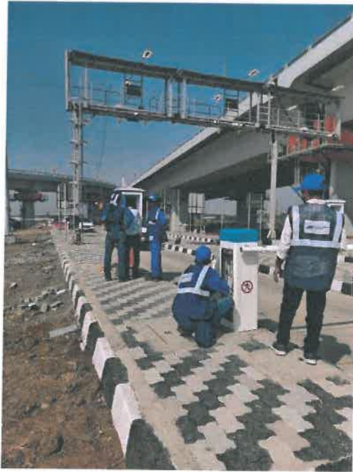
Photo 9,10,11- Temporary Road Connecting to Ramp 3 & 5 – Shivaji Nagar
