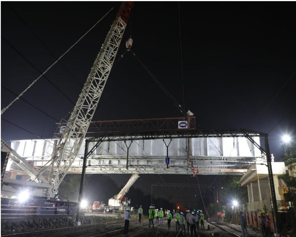
The 53-meter long girders were launched in three operations each comprising two girders at a time with the help of TEREX-DEMAG Crawler Crane of 600 MTonnes capacity. While the first two girders were launched between 1.06 am and 1.34 am on Sunday, the next two girders were launched between 2 am and 2.46 am on Monday. The remaining set of two girders was launched between 2.22 am and 3.18 am on Tuesday.
