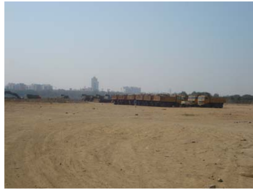
Vacant Area in BKC for Proposed BRTS Terminal
