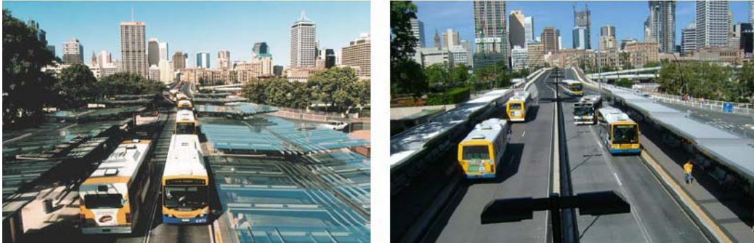
Figure 4.4 : Brisbane miscalculated demand (left, the problem eventually had to be corrected through a somewhat costly retrofit of a passing lane at the station (right)
