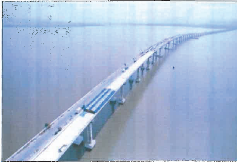
Figure 13: Deck water proofing at OSD section
