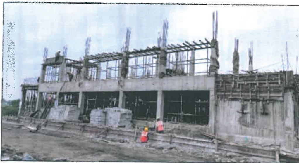
Figure 29: Shivaji nagar Sub-admin building- reinforcement fixing, binding and shuttering work is in progress
