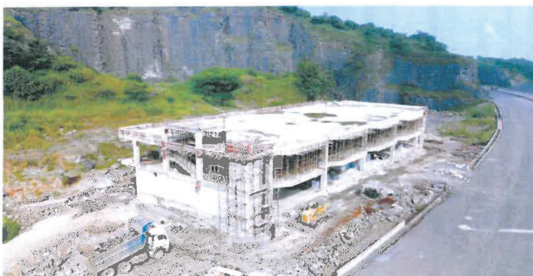
Figure 25: Food Plaza-1- First floor slab shuttering fixing is in progress.
