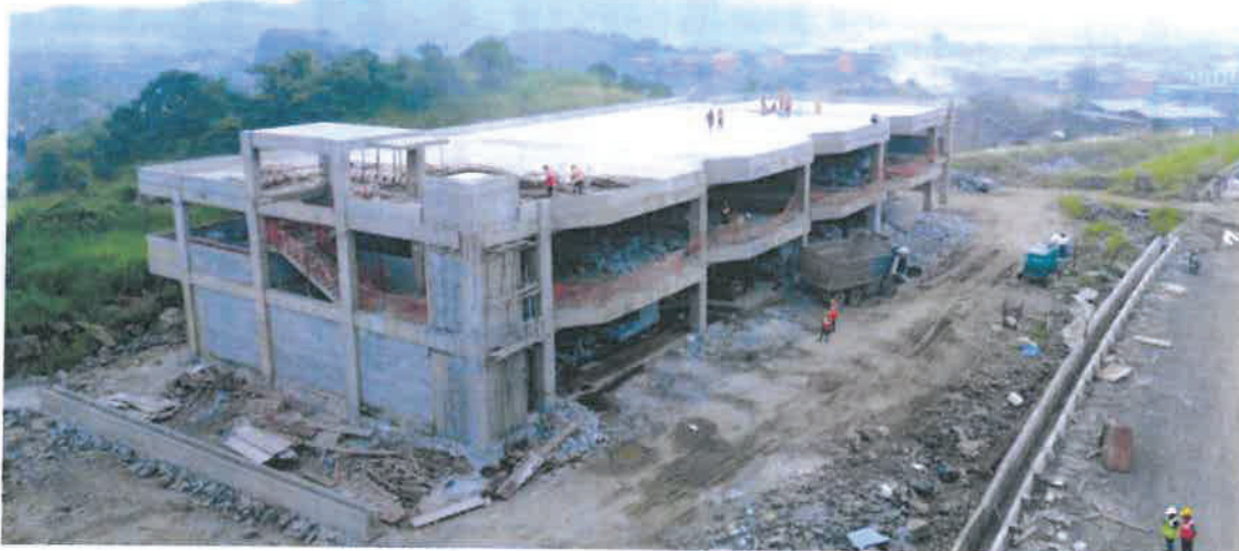
Figure 26: Flood plaza 2- First floor slab casting completed
