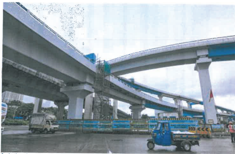
Figure 2: Anti carbonation painting with new shade & drainage system installation in progress at Ramp C1 & Ramp B
