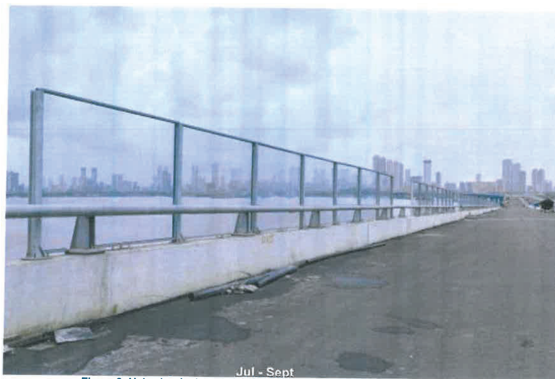
Figure 6: Noise barrier installation & crash barrier handrail fixing in progress
