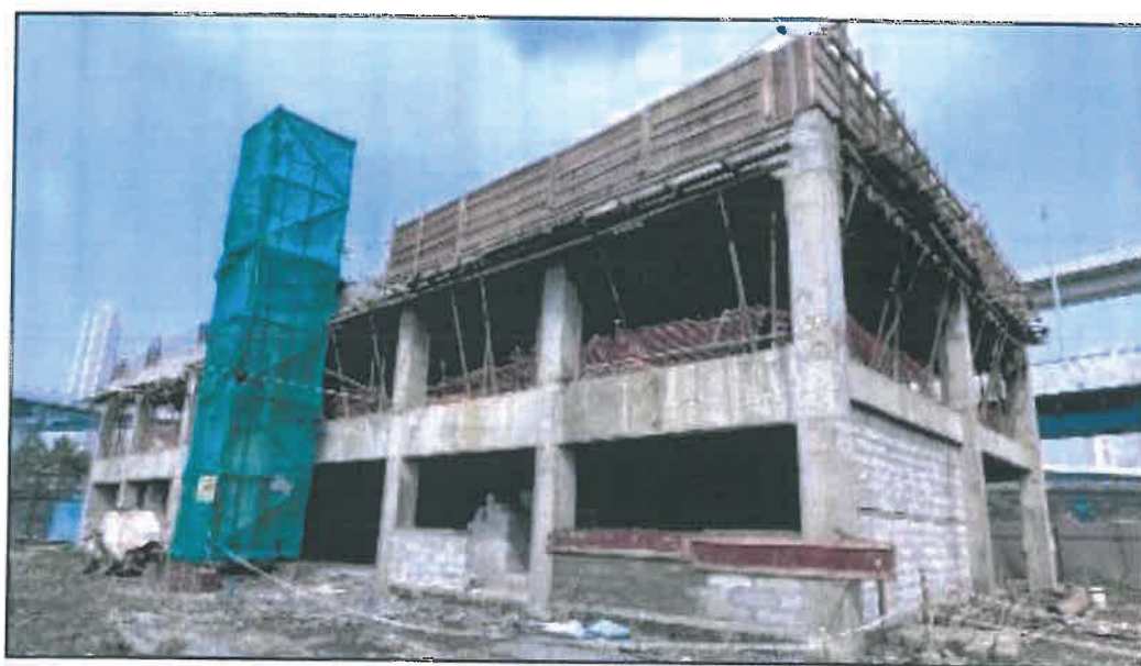
Figure 30: Sewri Sub admin building - First floor slab shuttering & block work is in progress
