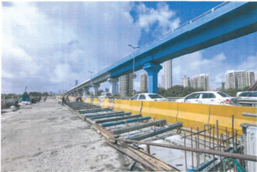
Figure 3: Longitudinal Expansion joint completed at C1 Ramp
