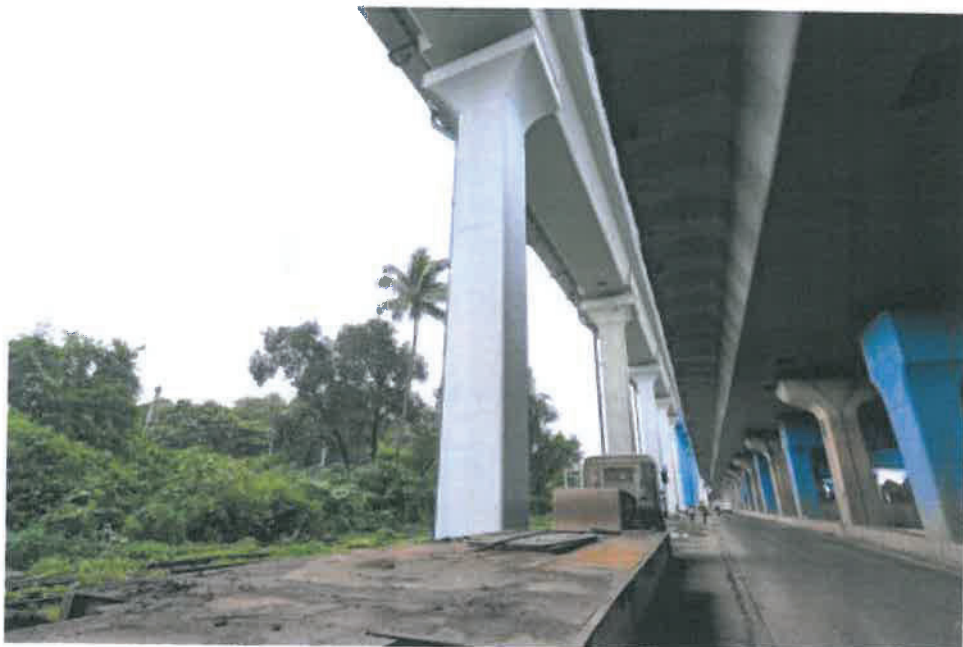
Figure 1: Anti carbonation painting with new shade & drainage system installation in progress at Ramp A
