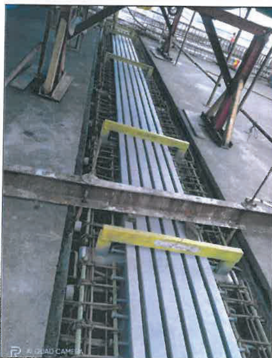
Figure 16: Expansion joint Rebar fixing in progress.
