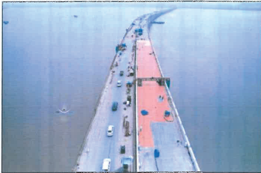
Figure 14: Deck water proofing at OSD section
