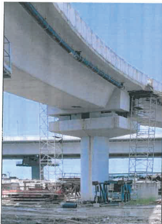
Figure 11: JM ramp runner pipe erection in progress
