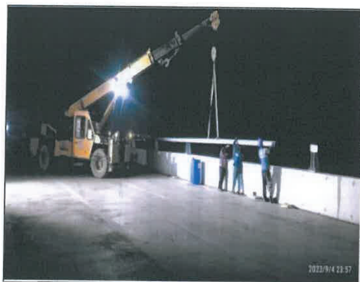
Figure 15: Hybrid rail fixing in progress
