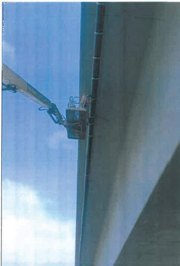
Figure 10: Runner Pipe Erection in Progress
