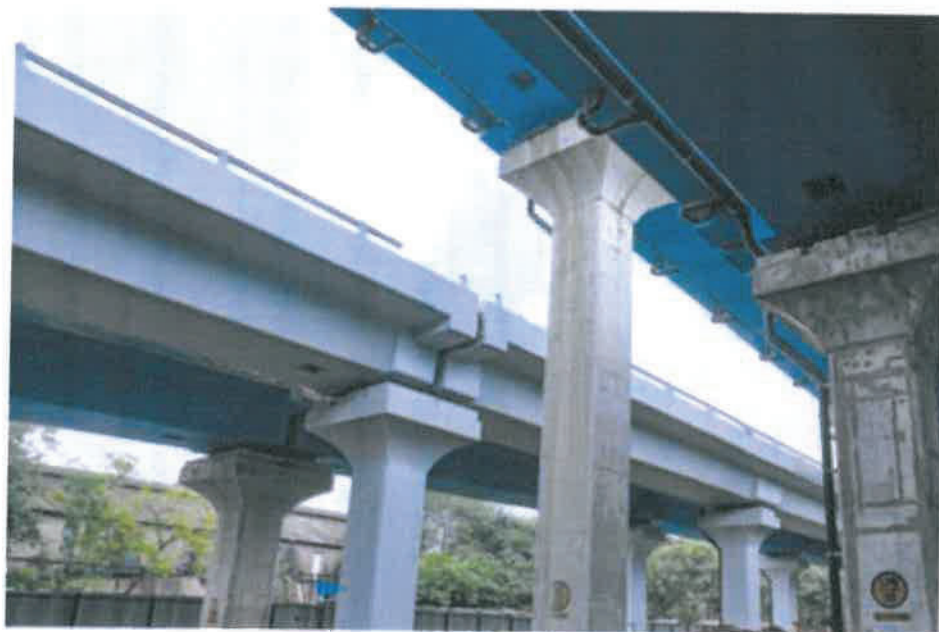
Figure 5: Anticarbonation painting in progress at Ramp E
