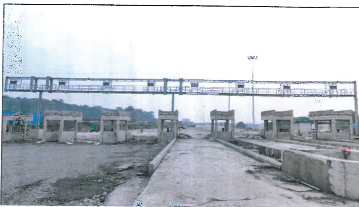
Figure 27: Gavhan Toll Plaza - LHS & RHA side gantry fixing is completed
